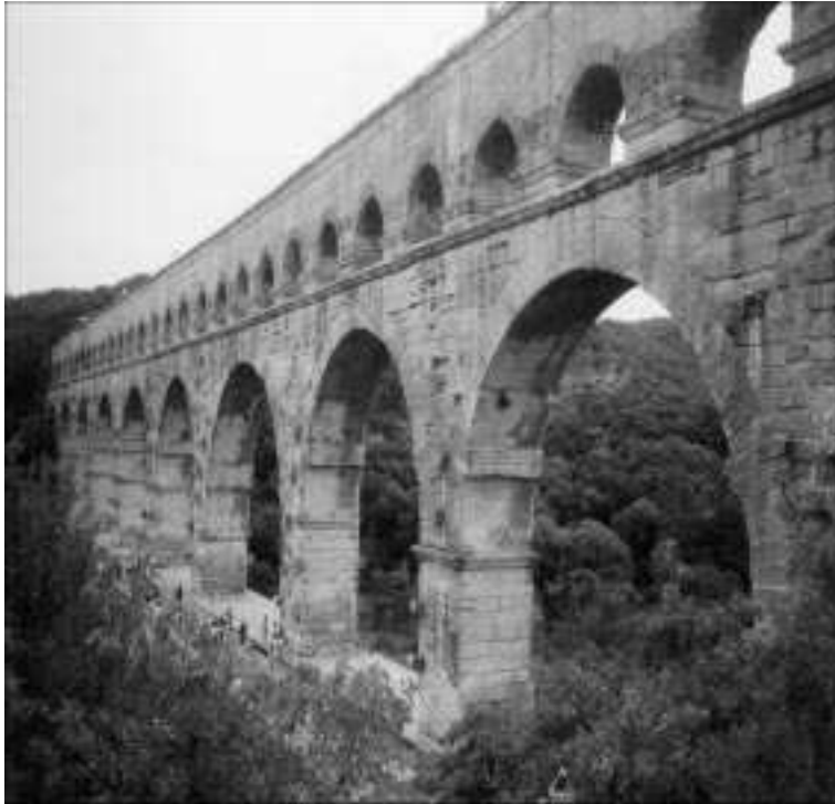
7.1 The Pont du Gard, part of a 50 km aqueduct constructed by the Romans in the first century AD near Nîmes in southern France, with mortar joints containing pozzolanic cement.
