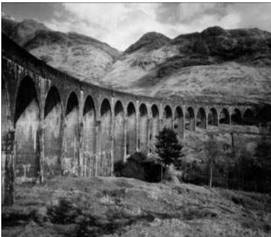
1.6 The Glenfinnan Viaduct, a 21-arch concrete railway viaduct constructed in 1897 in the West Highlands of Scotland.
