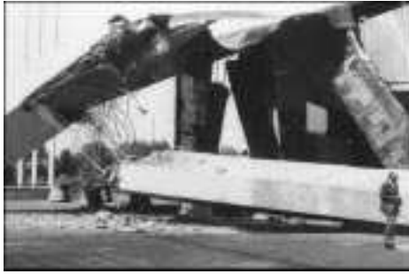
6.1 Collapse of southern outer roof of Berlin Congress Hall.
