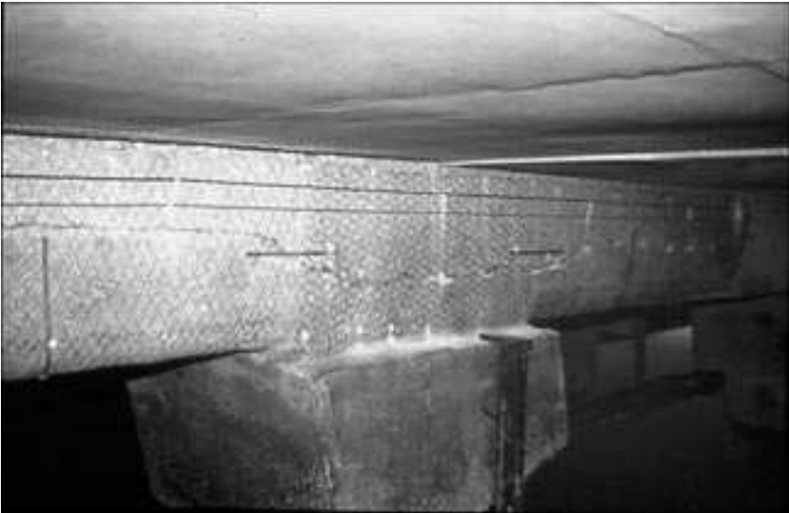
5.17 (a) Conductive paint extended anode for applying cathodic protection to a reinforced concrete structure. (b) Activated titanium mesh anode (shown prior to being coated with a concrete overlay) for applying cathodic protection to a reinforced concrete structure.
