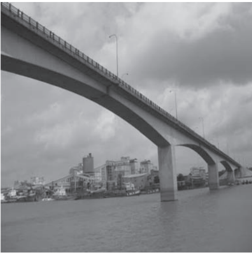
Figure 1. The Meghna Bridge.
