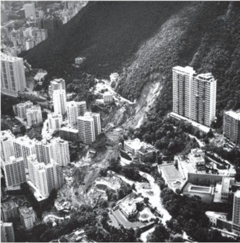
Figure 2. The Po Shan landslide on 18 June 1972.
