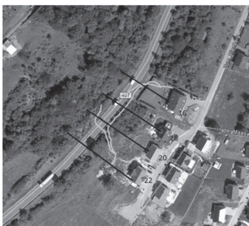
Figure 2. The road, four houses, four parallel cross sections and cracks in the ground (under laying photo: Google Maps).
