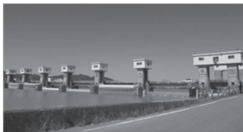
Figure 1. External appearance of the target dam.
