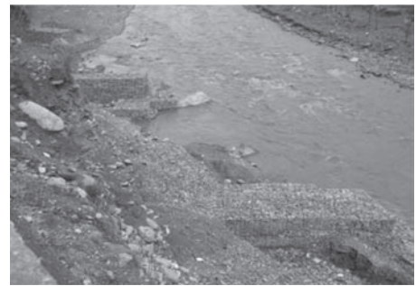
Plate 5. River erosion protection.
