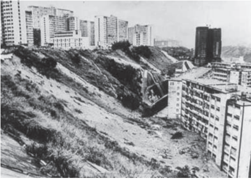
Figure 3. Fill slope failure at Sau Mau Ping on 25 August 1976.
