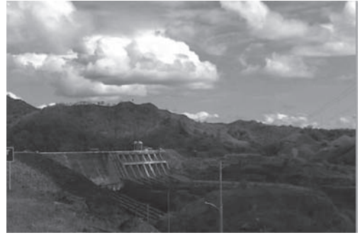
Figure 4. General view of the dam looking north west.
