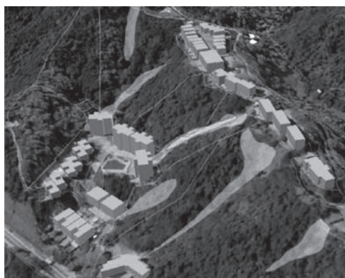
Figure 6. Residential buildings affected by landslide hazards at Sha Tin Heights (after Wong & Ho 2005).
