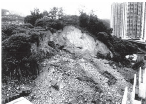
Figure 8. Failure of cut slope at Fei Tsui Road on 13 August 1995.
