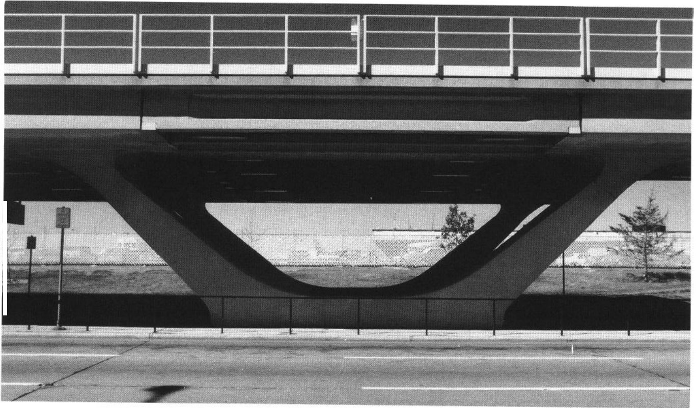
O'Hare Field elevated roadway (photo courtesy of Alfred Benesch and Company)
