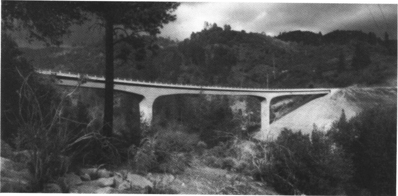
Post-tensioned concrete bridge in California cast monolithically with an integrated pier
