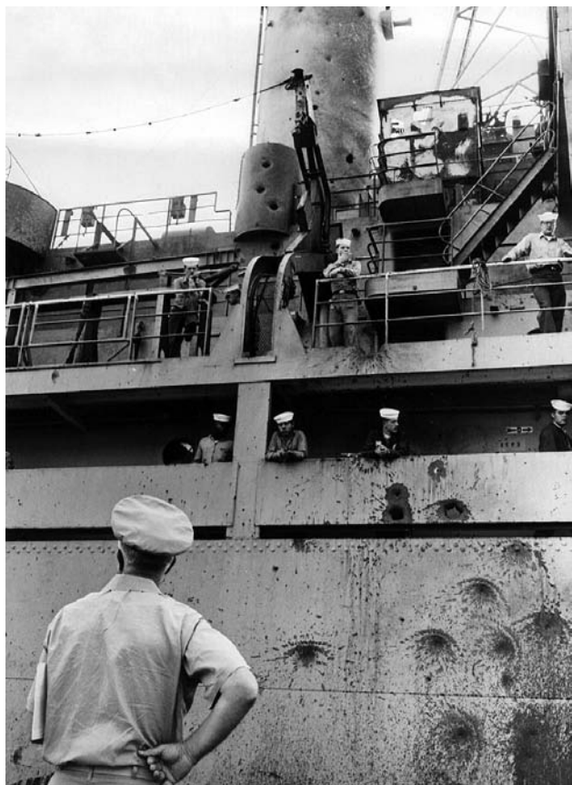
Gunfire and rocket damage to the U.S. Navy intelligence-gathering ship Liberty , inflicted when it came under attack by Israeli forces off the Sinai Peninsula on June 8, 1967. (U.S. Navy)
