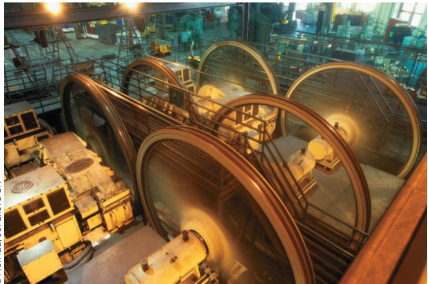
These pulleys and cables are part of the San Francisco cable-car system.
