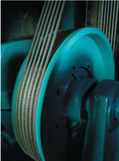
This pulley-cable system is part of an elevator mechanism.
