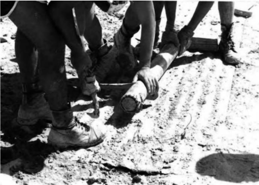
FIGURE 1.67 Removal of the cutting bit from the Denison core barrel after coring cemented silty sands.
