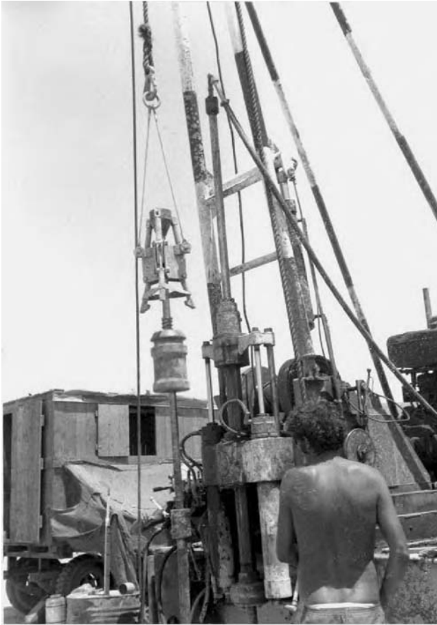
FIGURE 2.58 Quick-release drop hammer used in Israel and Europe for SPT sampling.
