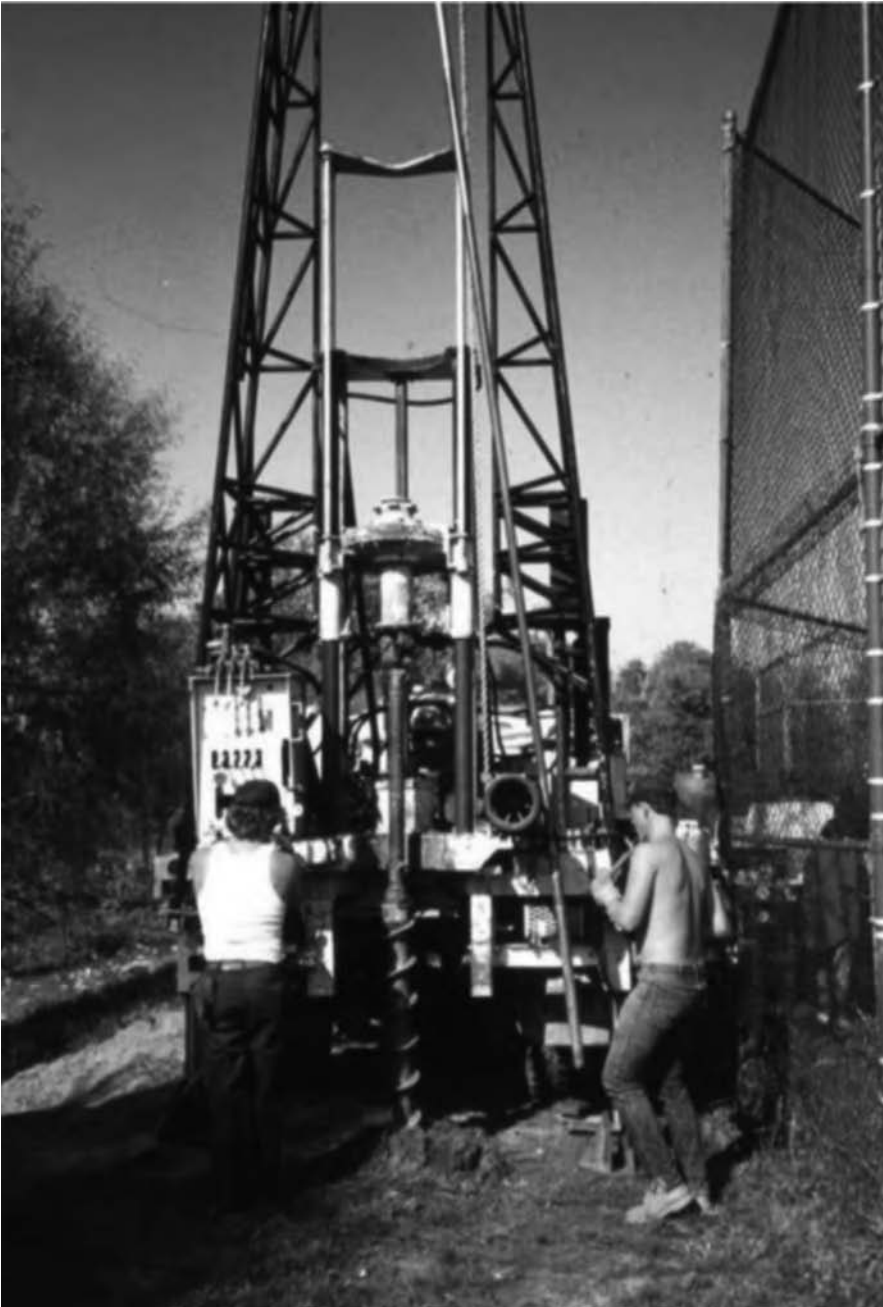
FIGURE 1.51 Rotary drill rig advancing boring with the continuous hollow-stem flight Auger.
