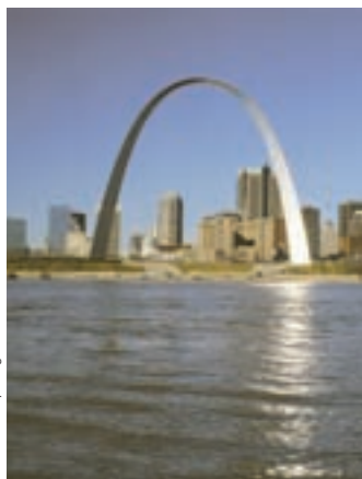
The Gateway Arch in St. Louis was designed using a hyperbolic cosine function (Exercise 48).
