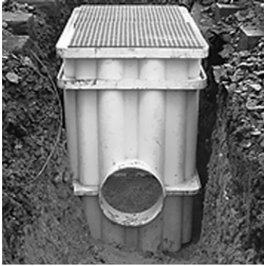
7.30 Water catchpit for rail track drainage applications (courtesy of Marton Geotechnical Services).
