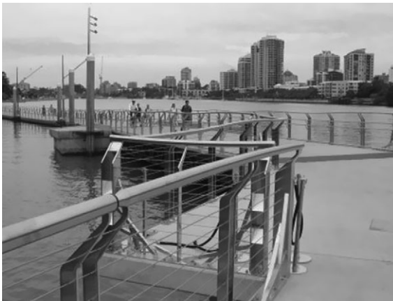
7.39 Brisbane river walkway constructed using GRP, Brisbane, Australia.
