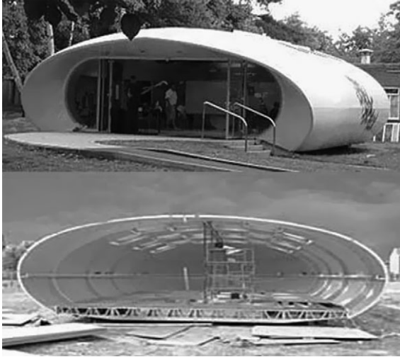
7.40 GRP classroom, complete and under construction (courtesy of White Young Green).
