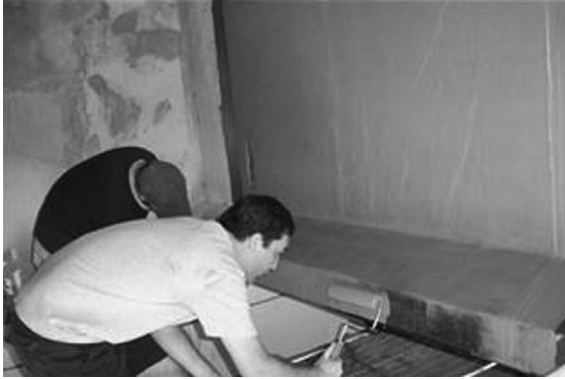
4.30 Latex-based coating application.
