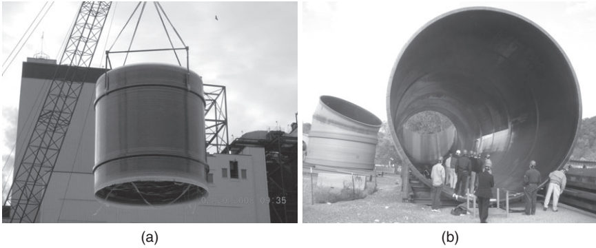
16.10 Large diameter FRP chimney flue liner: (a) module liner section; (b) connection elbow.
