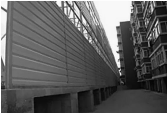
7.20 GRP absorbent noise barrier (courtesy of Jiangsu Shuangying Acoustics Equipment Co. Ltd).
