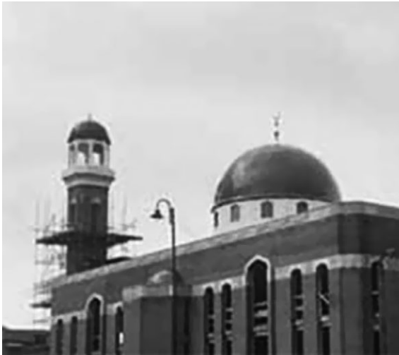
7.9 GRP dome on a mosque (courtesy of David Kendall).
