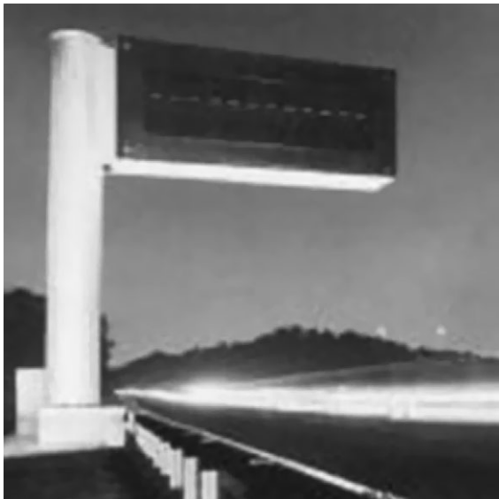
7.22 Motorway sign gantry (courtesy of NGCC).
