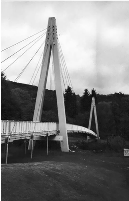
7.18 General view of Aberfeldy footbridge.
