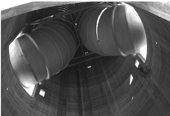
16.11 View of stack liner installation inside a power plant chimney.
