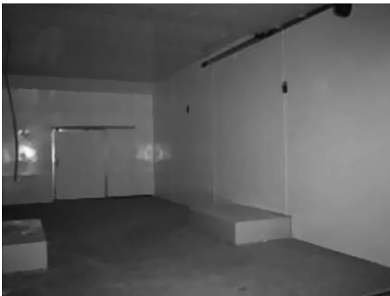
7.2 FRP wall panels used in a clean room (courtesy of Plastruct Canada Inc.).
