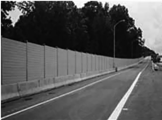
7.19 GRP reflective noise barrier (courtesy of NCN-UK).
