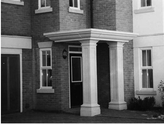
7.8 GRP pillars and porch (courtesy of IJF Developments Ltd).
