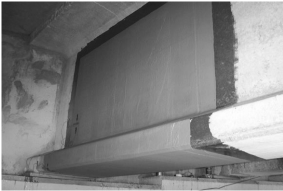
4.31 Final overall view of reinforced section.
