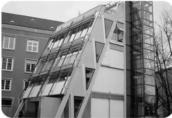
7.11 The Eyecatcher Building (courtesy of Fiberline Composites).
