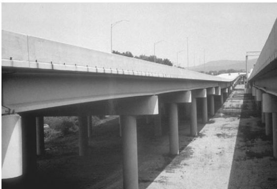
4.17 I-565 Highway bridge in Huntsville.
