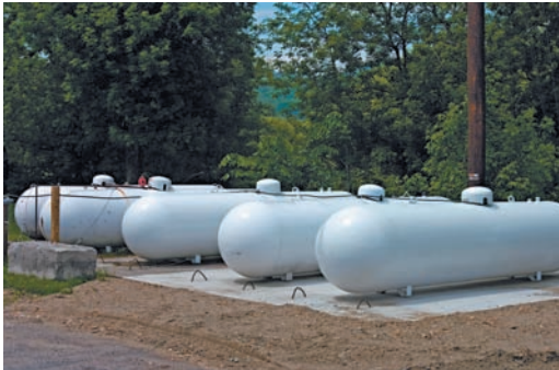
Photo 7.3 Cylindrical pressure vessels.
