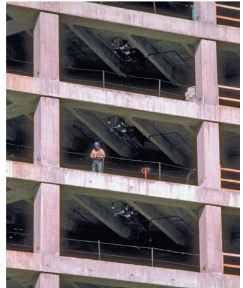
Photo 4.4 Reinforced concrete building.
