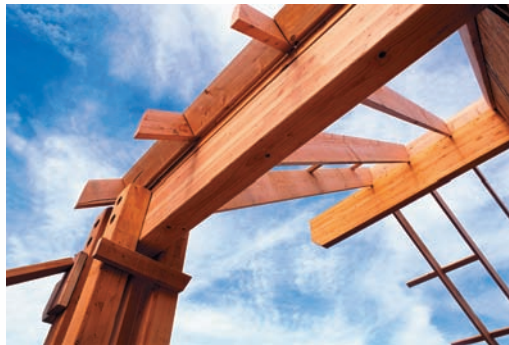
Photo 5.1 Timber beams used in residential dwelling.
