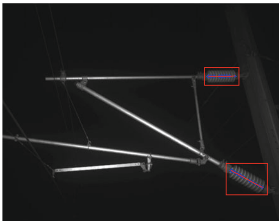
Fig. 6.11 Positioning result of multiple insulators
