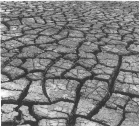
Dredged fill is particularly susceptible to dessication. (Photo courtesy U.S. Army Corps of Engineers.)
