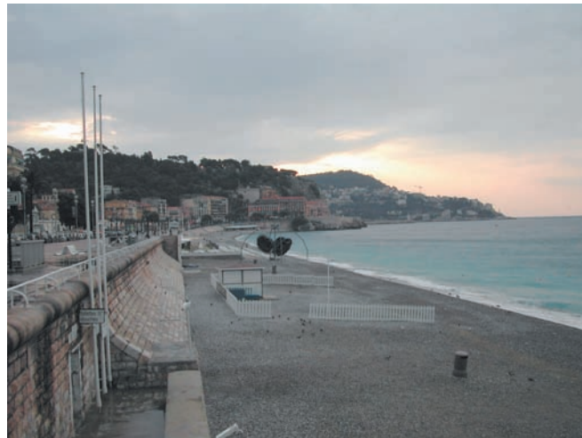
Plate 36.7. A protective sea wall constructed to repel and limit potential tsunami damage along the shoreline of Nice, France. This tsunami sea wall was constructed after Nice was struck by a tsunami triggered by a construction-generated shoreline landslide. (Source: author.)
