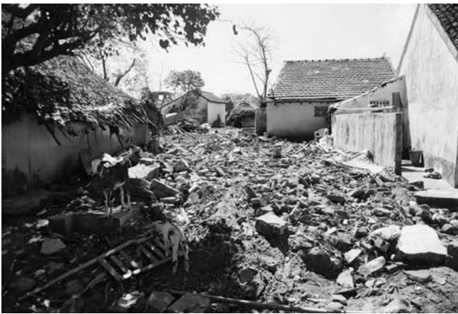
Figure 36.5. This picture taken in Karaikal, India after the 2004 Indian Ocean tsunami shows the debris field left by the tsunami waves. High-force movement of heavy debris and sharp objects within a tsunami wave cause major injuries to exposed humans and animals. (Source: United States National Oceanic and Atmospheric Administration, by Joseph Trainor, University of Delaware, Disaster Relief Center.) See color plate.
