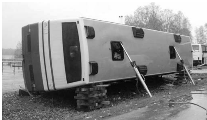
Figure 18.16. If people are trapped under a bus constructed of steel, it can be quickly lifted with extended hydraulic cylinders in the corners of roof hatches or with two air bags. See color plate.
