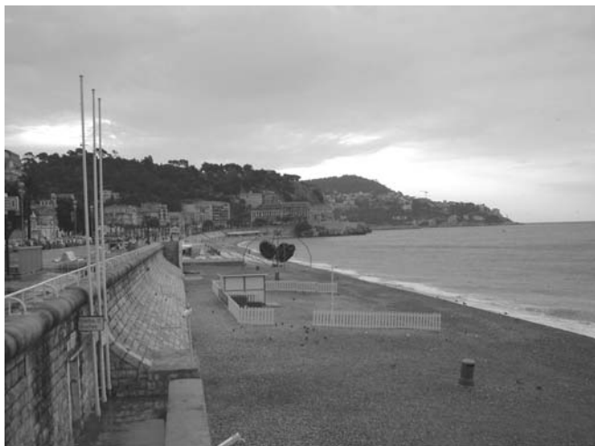
Figure 36.7. A protective sea wall constructed to repel and limit potential tsunami damage along the shoreline of Nice, France. This tsunami sea wall was constructed after Nice was struck by a tsunami triggered by a construction-generated shoreline landslide. (Source: author.) See color plate.
