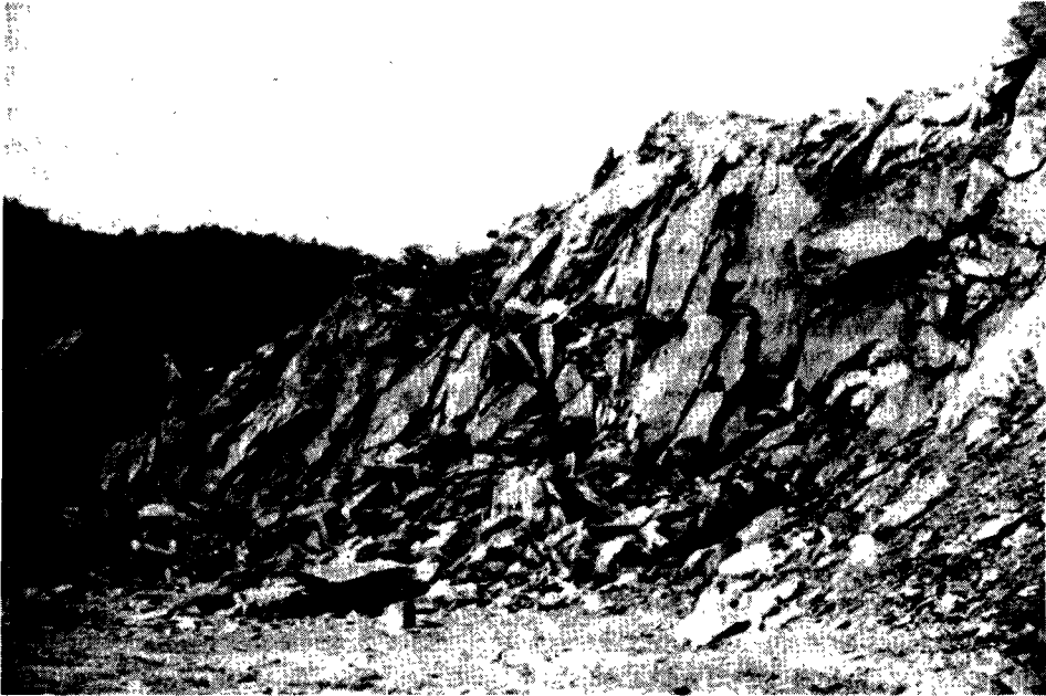
Figure 3.14. Schist being quarried in the spillway excavation at Kangaroo Creek Dam. Note the platy shapes of the rock fragments.
