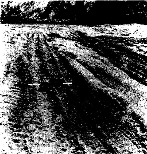
Figure 3.15. Slurry (Gravelly sandy silt) formed on the top of schist rockfill layer as a result of compaction by 4 passes of a 10-tonne vibrating roller (from Trudinger 1973).
