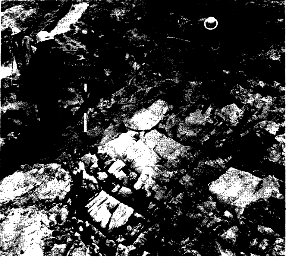
Figure 11.4. Cutoff foundation for Blowering Dam showing open joints being treated with pneumatically applied mortar, but no treatment for other joints (courtesy of Snowy Mountains Hydro-Electric Authority).
