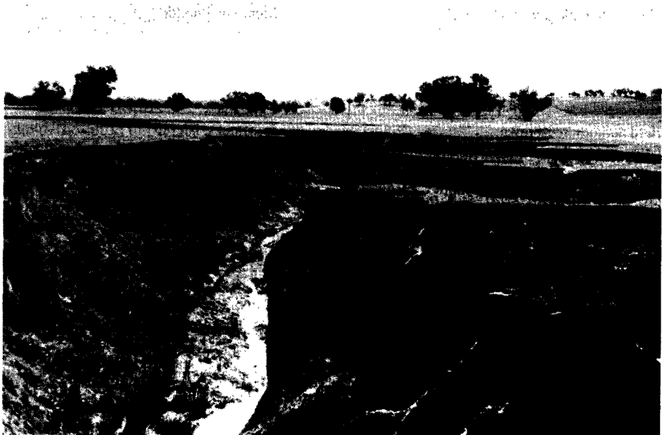
Figure 8.24. Deep erosion gullying in dispersive soils (Soil Conservation Service of NSW).
