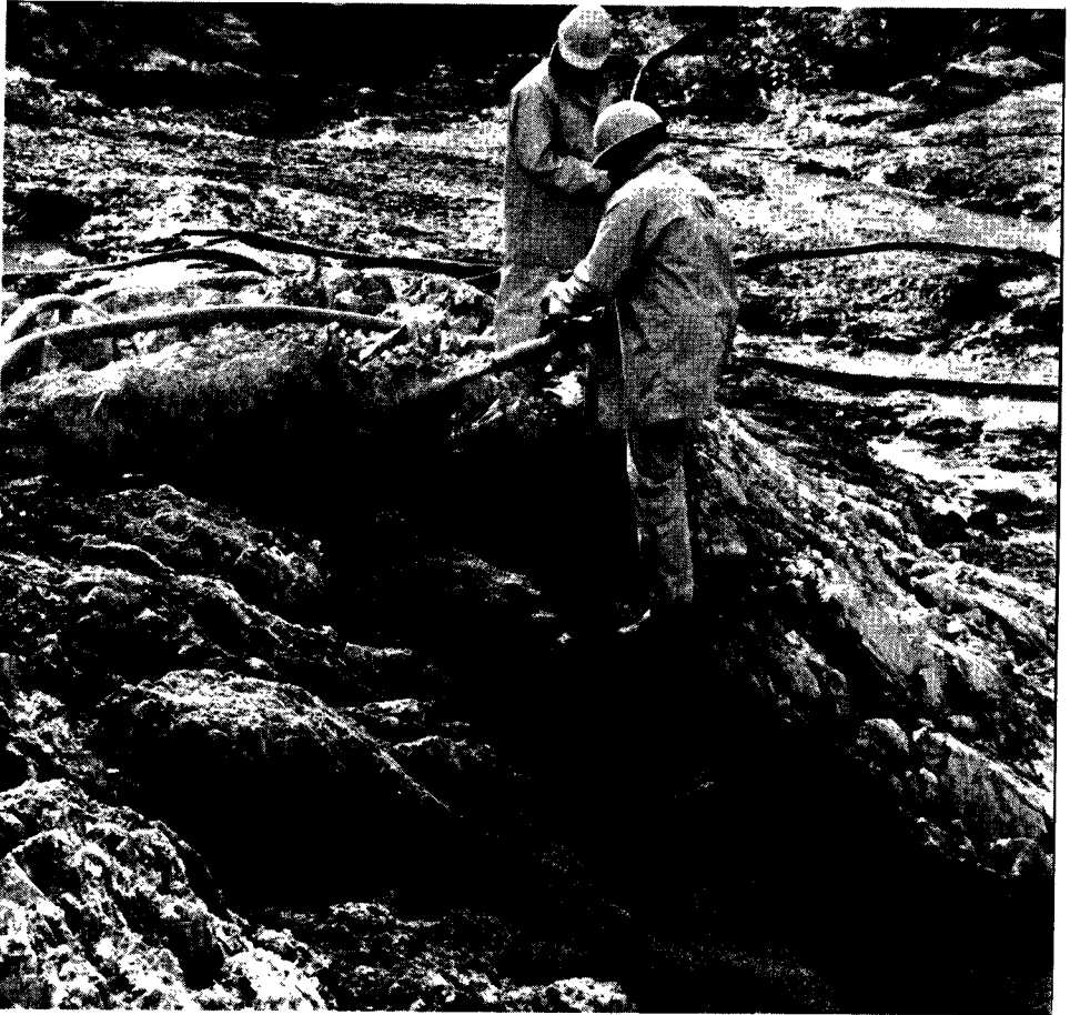
Figure 11.5. Application of pneumatically applied mortar on seams in the cutoff foundation of Blowering Dam (courtesy of Snowy Mountains Hydro-Electric Authority).
