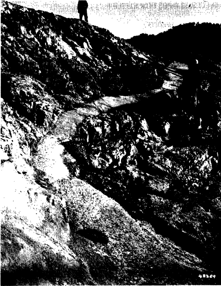
Figure 11.6. Left abutment of Blowering Dam after treatment of large fault zone and weathered seam (courtesy of Snowy Mountains Hydro-Electric Authority).
