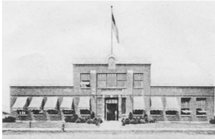
Austin No. 2 type building, a modern printing plant, of pleasing architectural appearance, built by Austin at Camden, N. J. Plate 199.
