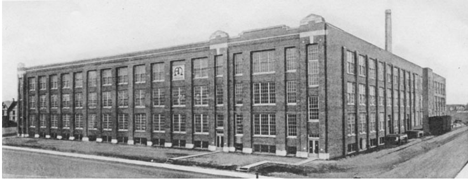
Austin No. 8 type building at Minneapolis with special architectural treatment, for large manufacturer of electrical equipment. Plate 249.
