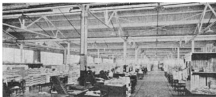
Austin No. 4 type building for large book publisher, Bloomfield, N. J. note evenly distributed daylighting. Plate 227.
