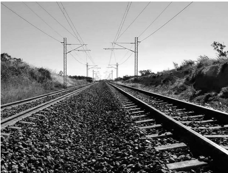
FIGURE 1.2 Duplicated track section on the Goonyella coal railway system.
