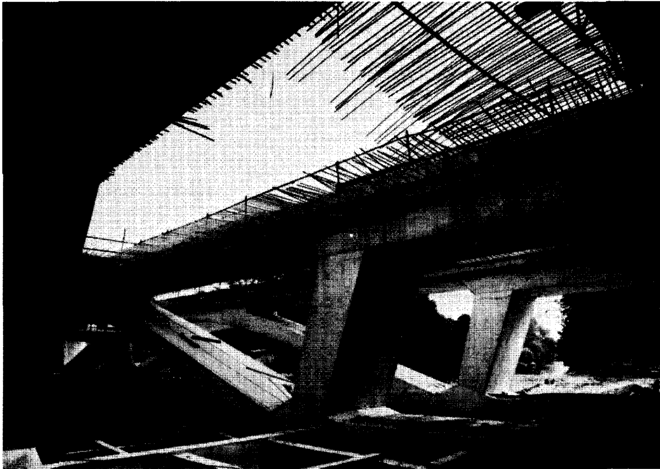
Prestressed concrete Runnymede Bridge over Thames River near Egham, Surrey, England. (Courtesy of Cement and Concrete Association.)
