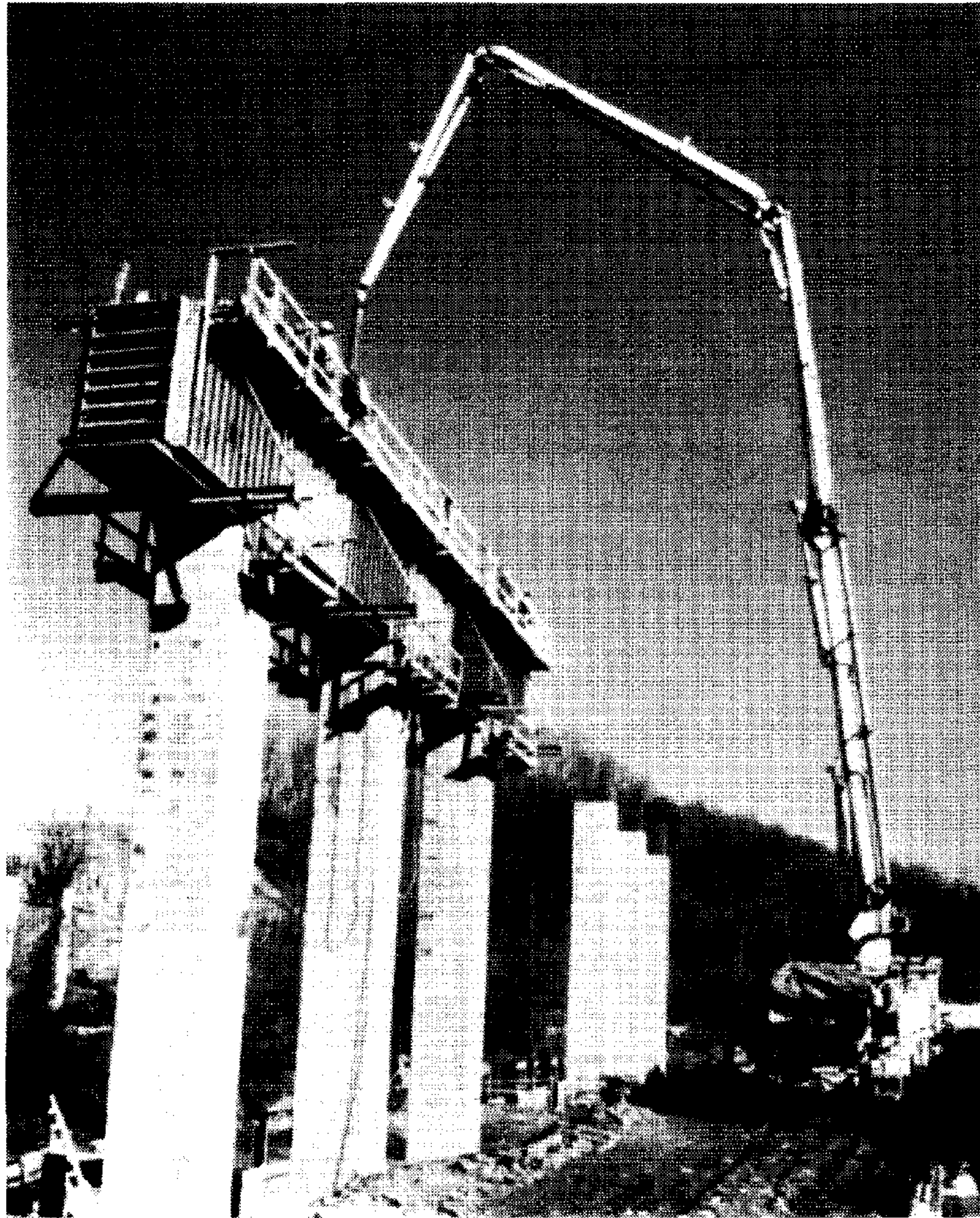
Pennsylvania Southern Expressway, Philadelphia, Pennsylvania. (Courtesy of Economy Forms Corporation.)
