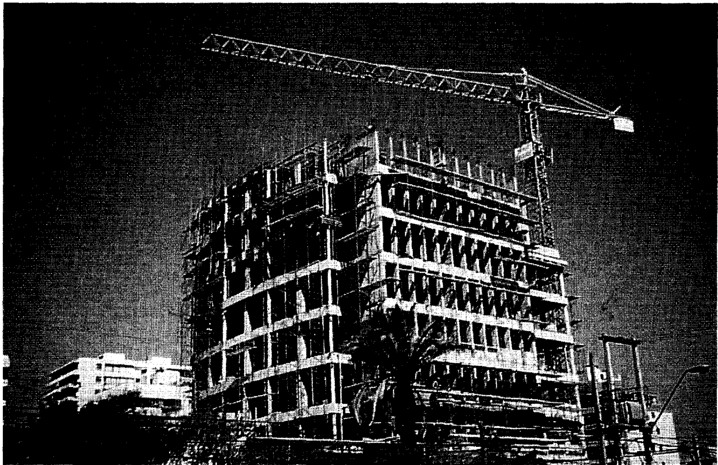
The 16-story Apoquindo Tower, Santiago, Chile. (Courtesy of Economy Forms Corporation.)
