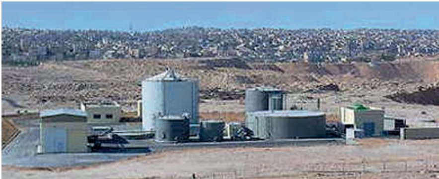
Figure 10.3. Biogas plant in Rusaifa/Jordan. Source: Al Husban 2006.
