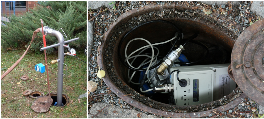
Fig. 1 On-situ continuous measurement of flow and Fig. 2 On-situ measurement of hydrodynamic pressure – underground hydrant hydrodynamic pressure
