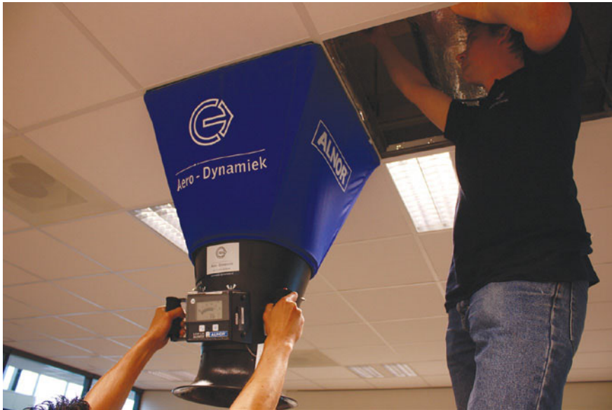
Figure 11.8 Testing, measuring and setting airflow
