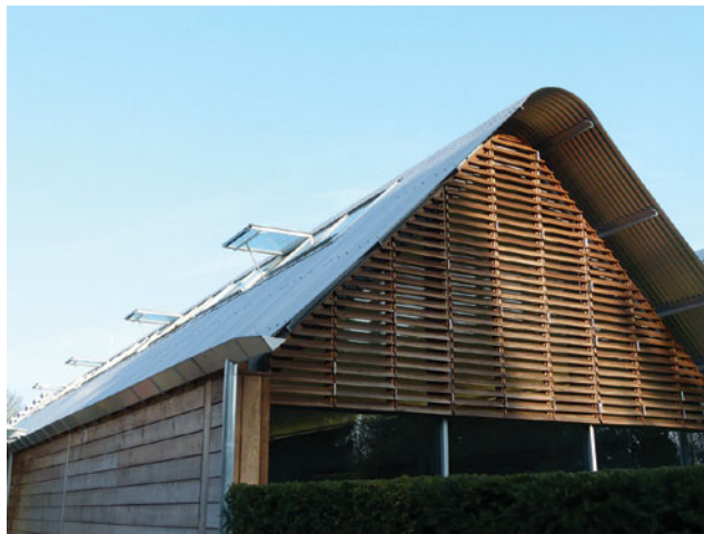
Figure 9.11 A good combination of high level natural cross flow ventilation and effective use of louvres to mitigate passive solar gain
