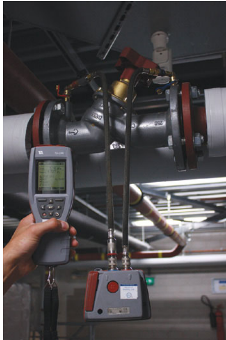
Figure 11.6 Commissioning – on-site validation and measurement of flow rates
