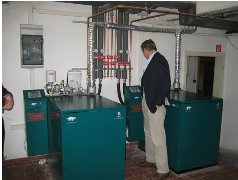
Figure 9.3 Combined heat and power
