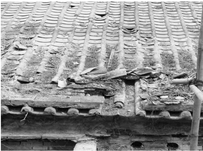
Fig. 13.7 Double-layer roof structure
