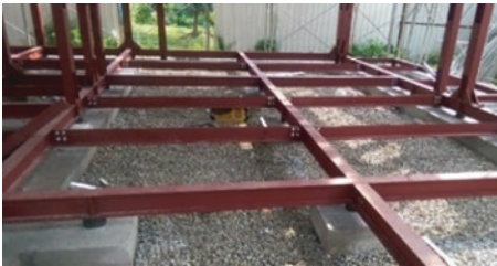
Fig. 14.12 Building the steel framework of the AG innovative composite structure
