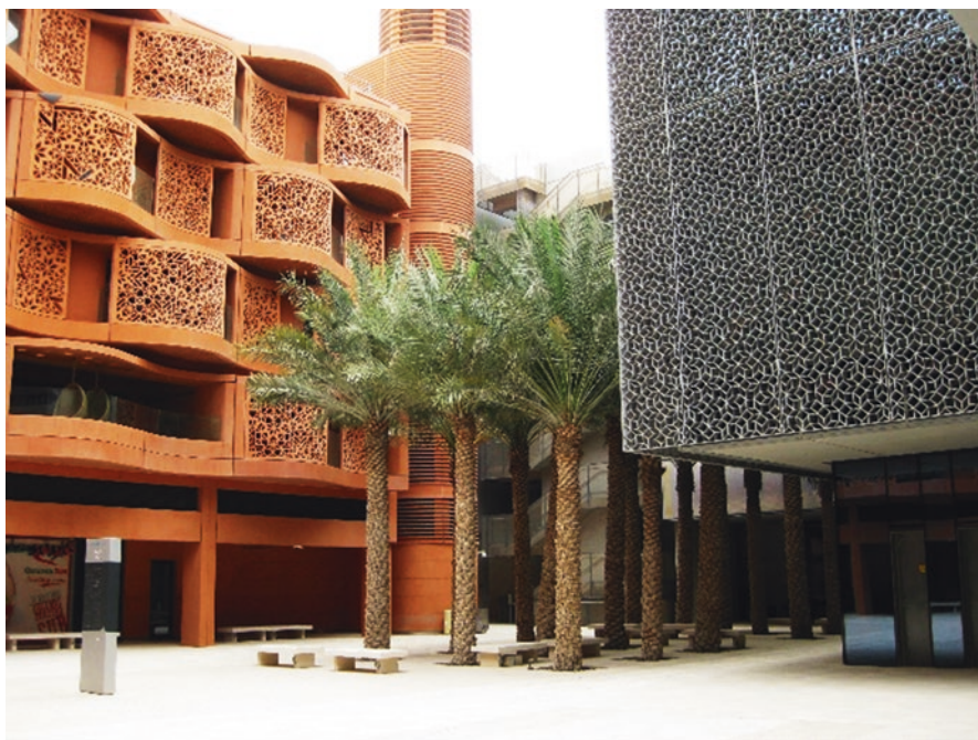
Fig. 15.3 Contemporary screens, Masdar City
