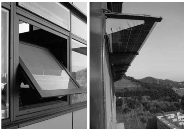
Fig. 4.11 Openable windows and outside sunshades
