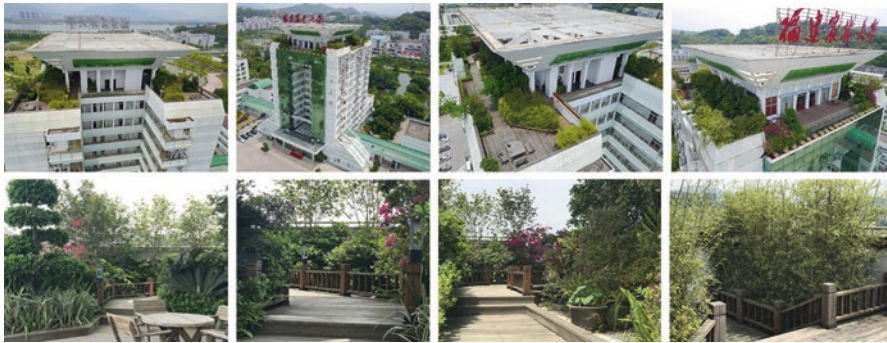
Fig. 9.3 Roof garden at the Fujian Agricultural and Forestry University
