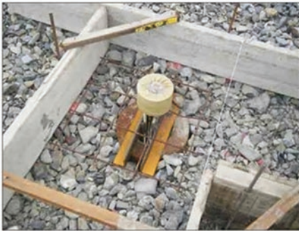
Grounded pile with damper
