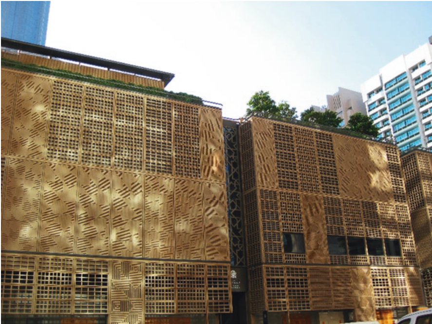
Fig. 15.4 Abu Dhabi Central Market: shading devices and roof garden
