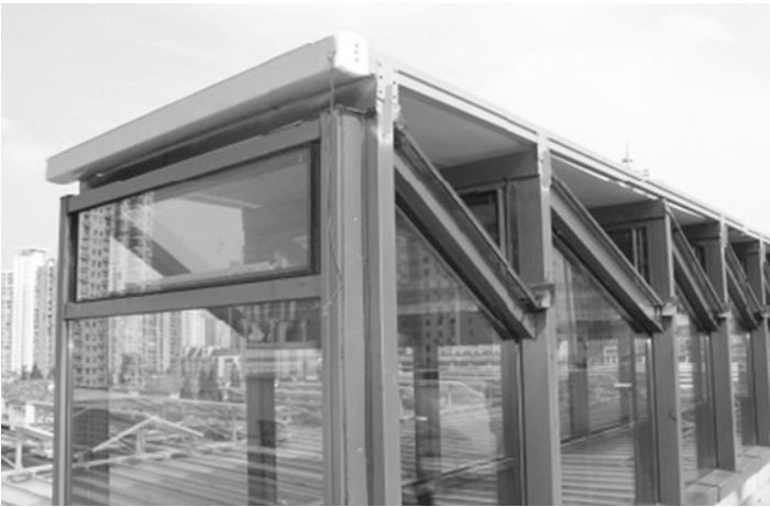
Fig. 4.19 Skylight of the building
