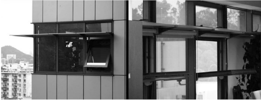
Fig. 4.12 Reflectors installed inside and outside windows for natural lighting
