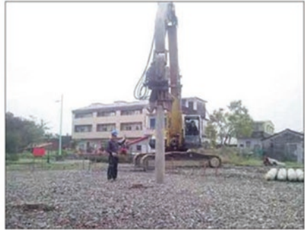
Hammering the foundation piles
