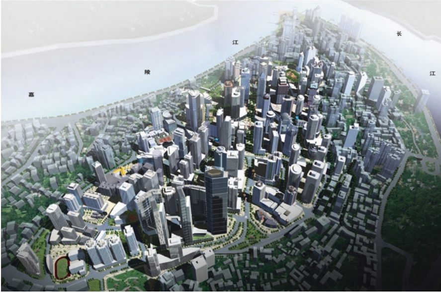
Fig. 6.1 Aerial view of the urban design of the core area in the Jiefangbei area, Chongqing
