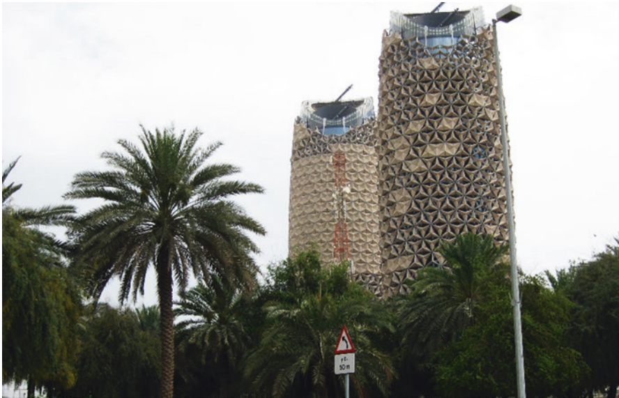
Fig. 15.6 Al-Bahr Towers, Abu Dhabi
