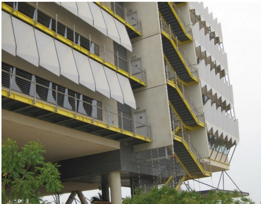
Fig. 15.5 Masdar: brise-soleil and pilotis creating shade and visual continuity
