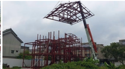
Fig. 14.12 Building the steel framework of the AG innovative composite structure
