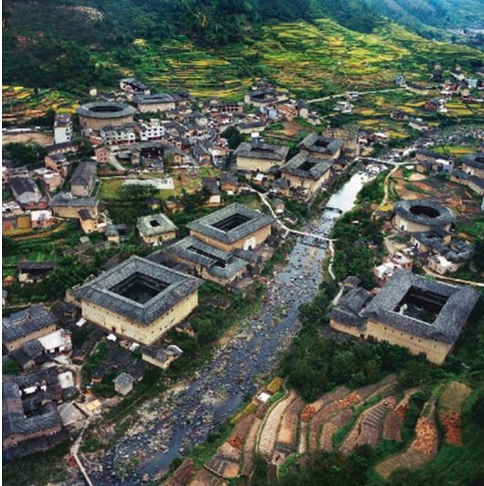
Fig. 12.2 Tulou (From: China Architecture & Building Press 2010)
