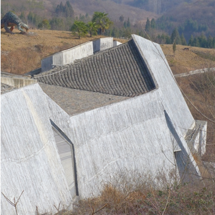
Fig. 13.3 Irregular concave side windows
