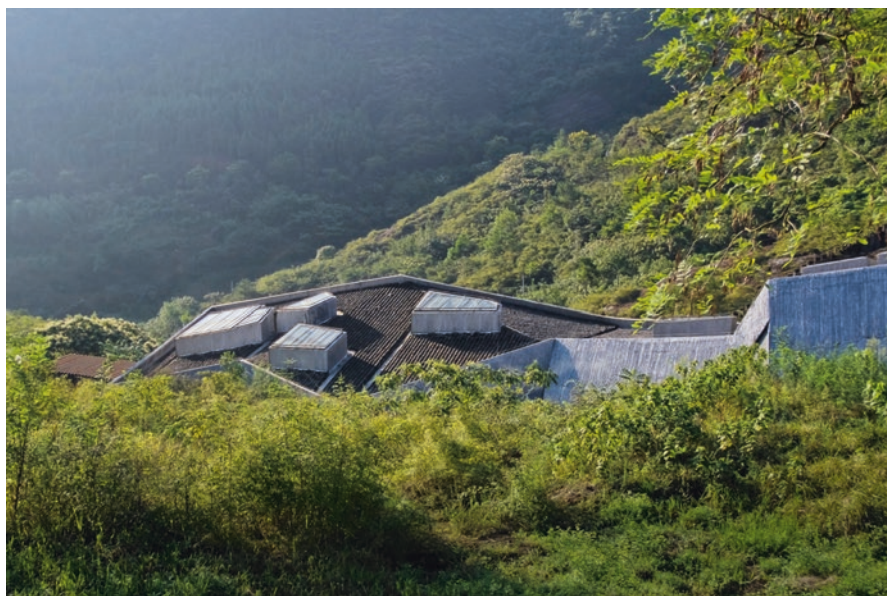
Fig. 13.9 New building with an old roof
