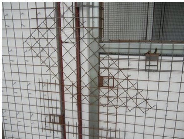
Fig. 14.2 Wall in the AGS1 composite building structure
