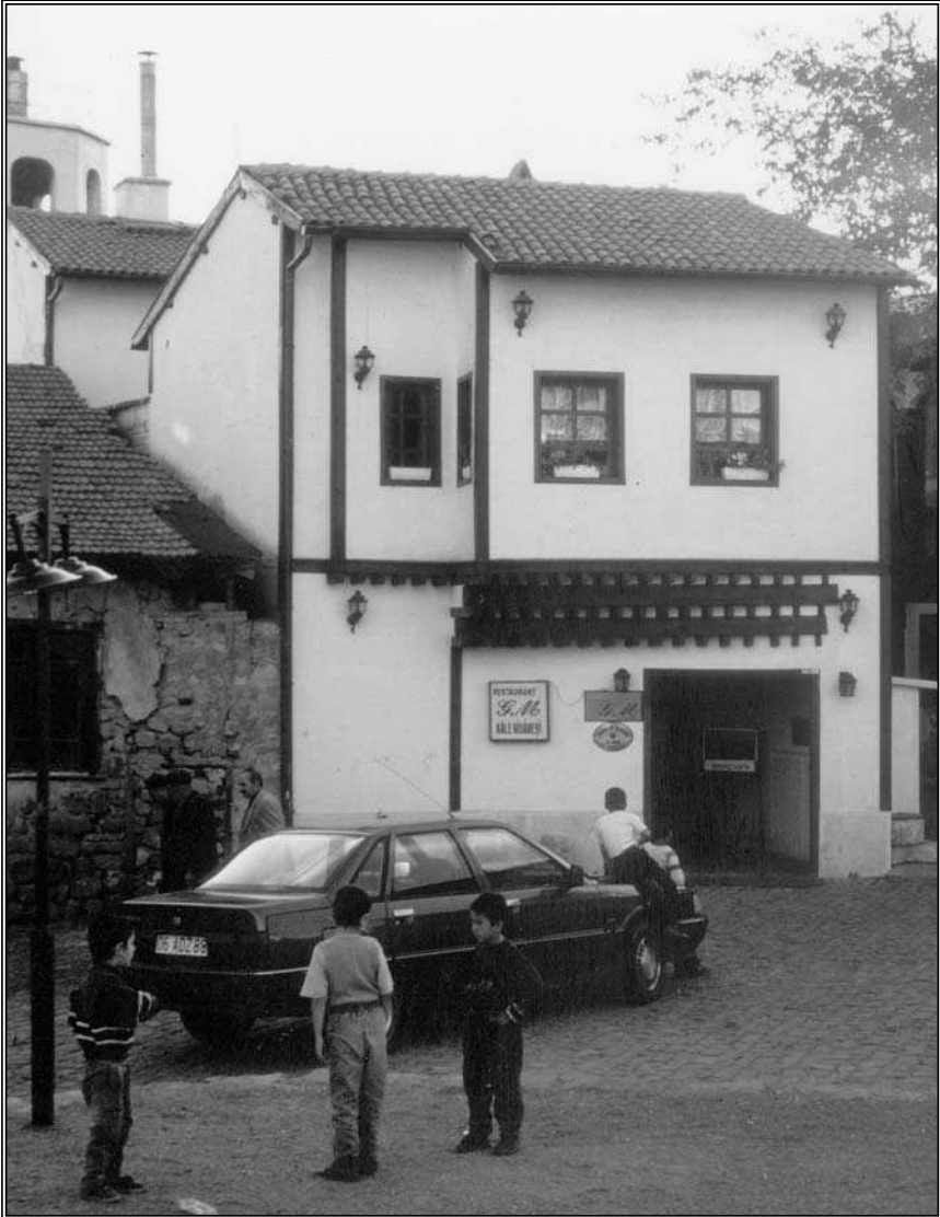
Figure 6.3 This traditional house in Ankara, Turkey, is a typical example of a commercial restoration, where the proportions of the ground floor have been altered to make way for the restaurant entrance.
