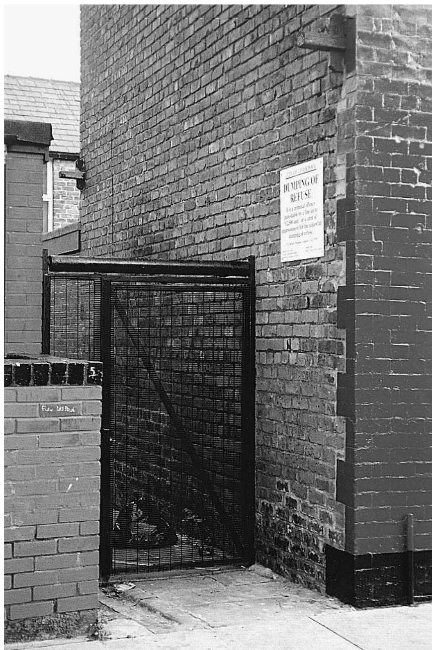
New alley-gate at the end of a terrace
