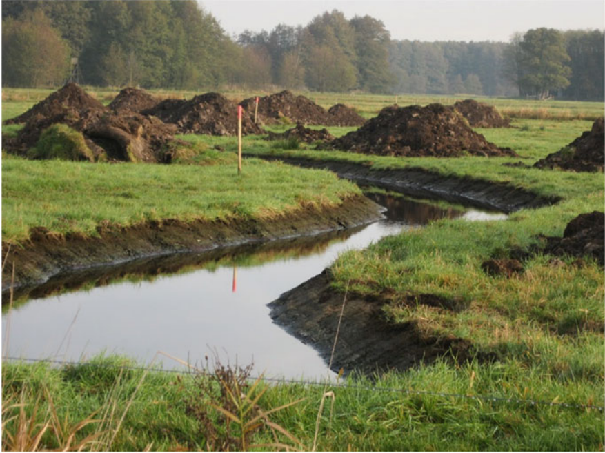
Fig. 9 Bringing the water back to the fen by building a new watercourse (2011)
