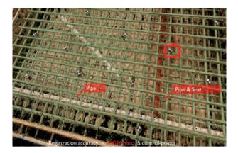
Figure 7.8: A 3D image-based point cloud model of a rebar cage. Using 15 control points, the up-to-scale point cloud model is transformed into the site coordinate system. © *MGF*
