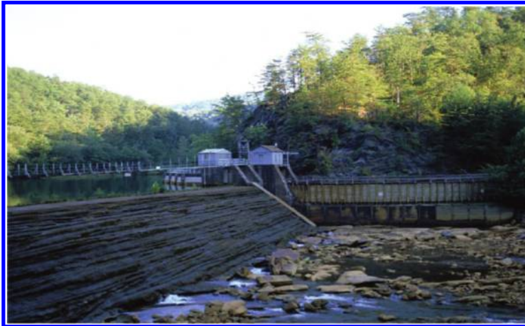
Figure 5. Ocoee Dam No. 2 after 27 years of service (provided by TVA).
