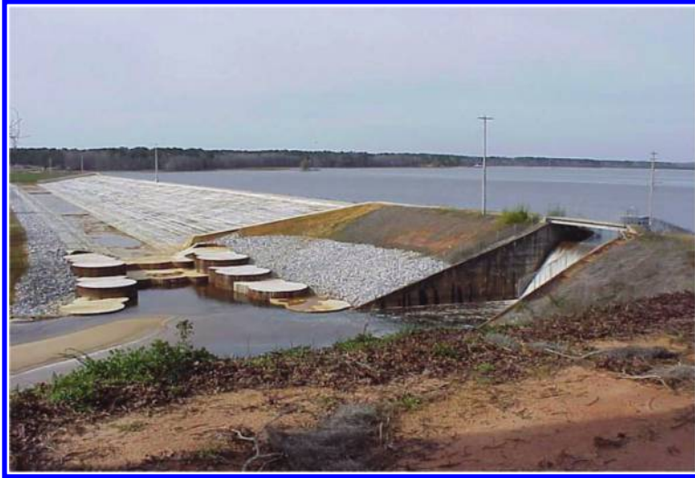
Figure 12. A view of principal and auxiliary spillways at Lake Tholocco Dam.
