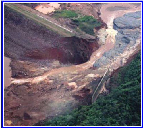
Figure 18. Algodoes Dam after failure.
