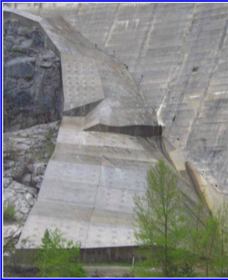
Figure 7. Concrete overtopping protection at downstream toe of dam (Reclamation).
