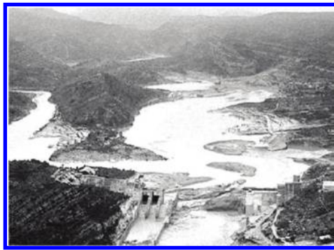
Figure 2. Image of the Tous dam after failure.
