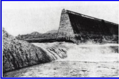
Figure 31. Khadakwasla Dam after failure.
