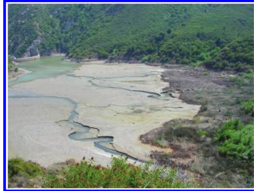
Figure 28. Silted up Matilija reservoir.
