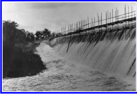
Figure 13. Muzuma Dam just before failure.
