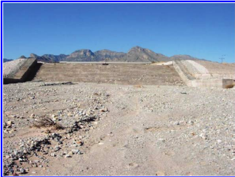
Figure 17. Red Rock RCC inflow spillway (February 2006).
