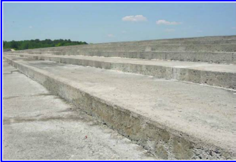
Figure 14. Excellent condition of RCC steps at Tholocco Lake Dam (May 2007).
