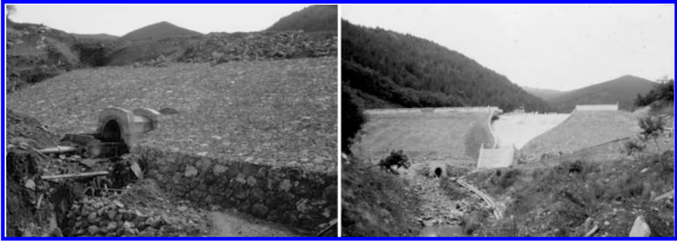
Figure 4. Llodio Dam. Left: upstream view. Right: downstream view.
