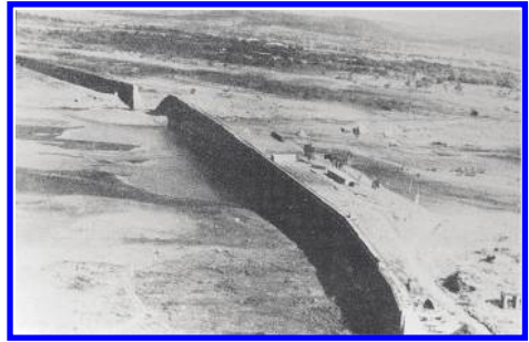
Figure 32. Kahadakwasla Dam after failure.
