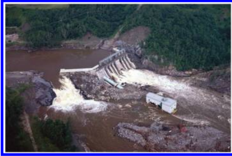
Figure 19. Ville de Jonquière Dam after failure.
