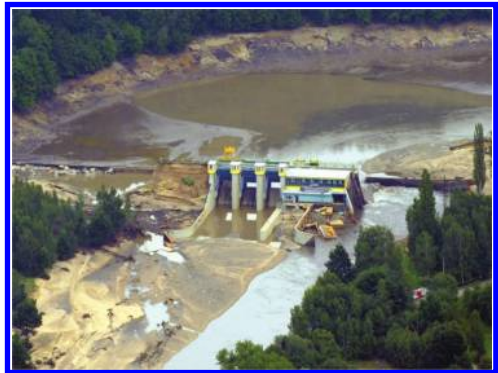
Figure 3. Niedow Dam after failure.
