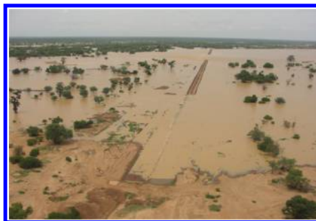
Figure 3. Liptougou dam protected against extreme floods by two spillways.
