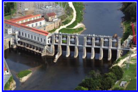
Figure 38. Tuileries Dam after gate failure.
