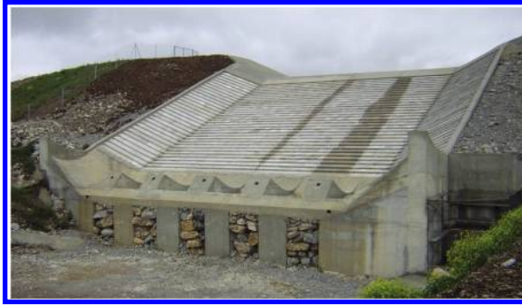
Figure 5. View of the spillway from downstream.
