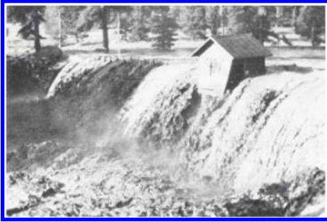
Figure 29. Cascade Dam failure sequence.
