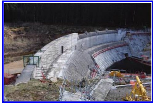
Figure 26. Des Plats Dam after rehabilitation.
