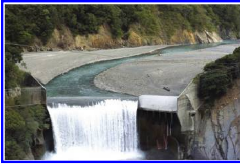
Figure 21. Baling Dam in November 2005.
