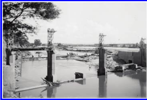
Figure 37. Yallourn Weir after failure.
