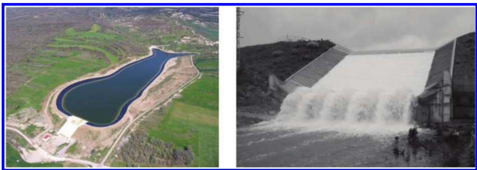
Figure 2. Left: Aerial view of Barriga dam (Source: Regional Authority of Castilla y León). Right: Spillway discharge (Source: José Manuel Ruiz, May 2008)
