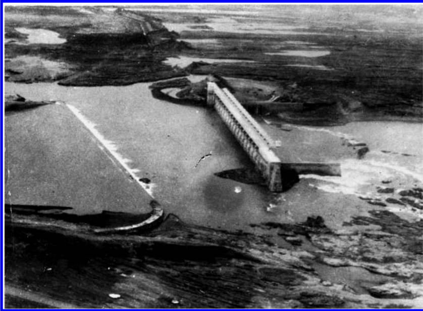
Figure 3. Machhu Dam II failure (photo credit: Gunvantbhai Sedani).
