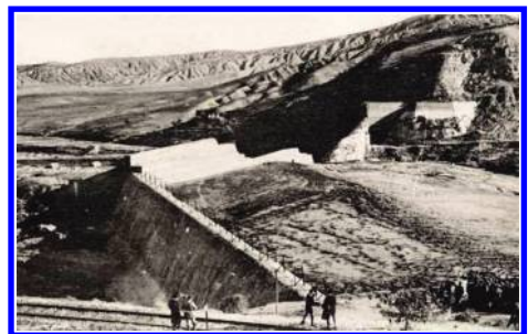
Figure 8. Habra Dam after its third failure.
