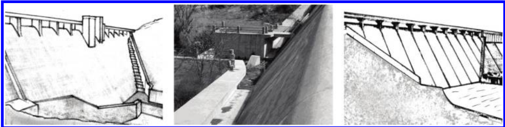
Figure 2. Three examples of dams with highly-converging chutes. Left: Nunome Dam (Japan), with RCC-stepped chutes. Center: Zapardiel de la Cañada Dam (Spain), with parabolic-floor chutes. Right: Torre Abraham Dam (Spain), in which the converging chutes were added after dam construction to increase the spillway capacity.
