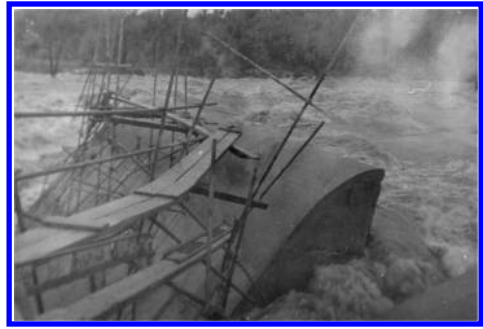
Figure 14. Muzuma Dam after failure.
