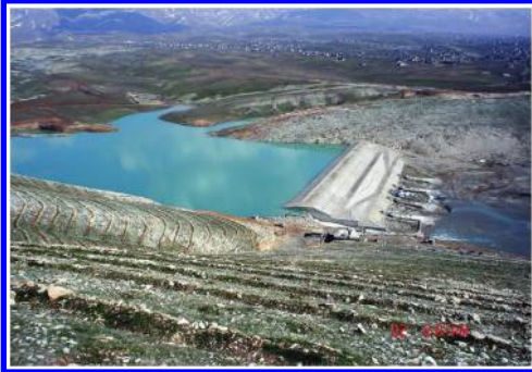
Figure 15. Chaq Chaq Dam in May 2005.
