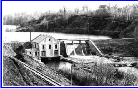
Figure 3. Fergus Falls Dam before failure.
