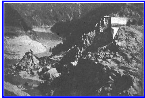
Figure 12. Sella Zerbino Dam after failure.
