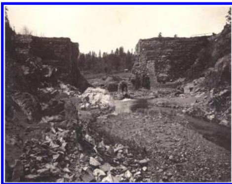
Figure 1. Lynx Creek Dam after failure.
