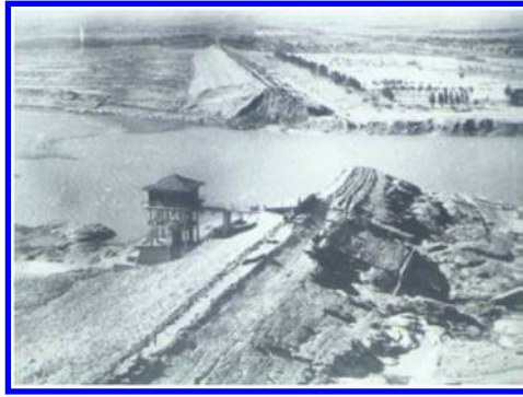
Figure 1. Image of Banqiao dam after the failure taken from (Banqiao 2010).
