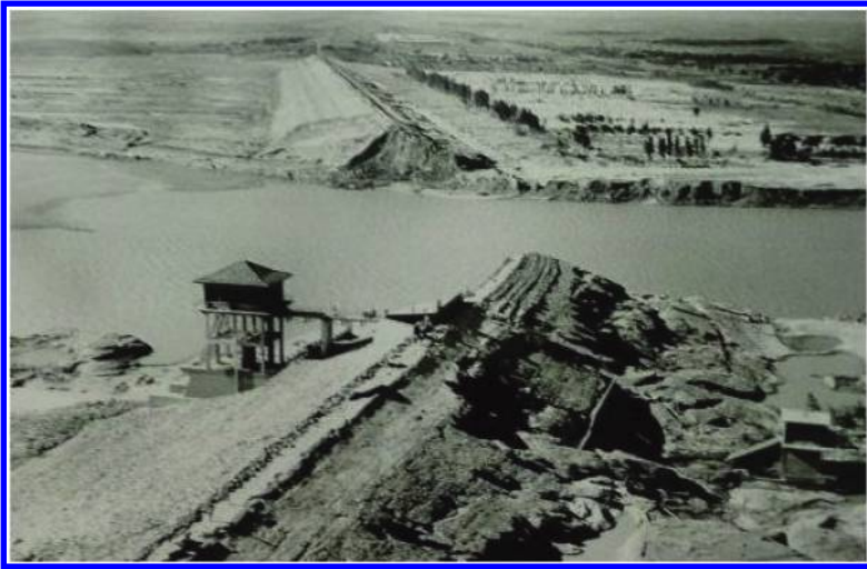
Figure 2. Banqiao Dam failure (photo credit: unknown).
