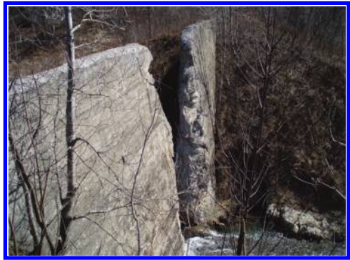
Figure 20. Ketner Dam core-wall today.
