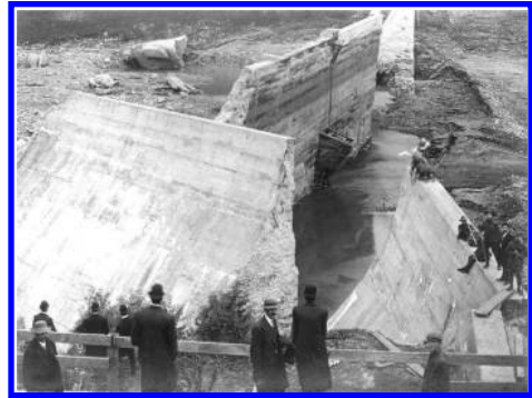
Figure 6. Bayless Dam after failure.
