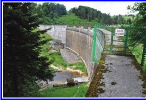
Figure 25. Des Plats Dam before reconstruction.
