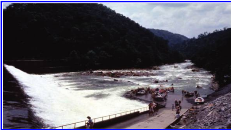
Figure 4. Close-up of Ocoee Dam No. 2 operating with rafters downstream.
