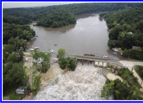
Figure 7. Lake Delhi Dam before failure.
