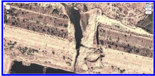
Figure 14. Detailed view of breach gap.
