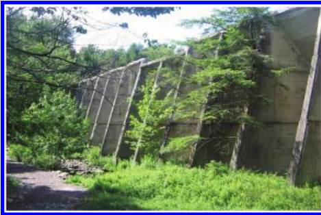
Figure 23. Lake Leigh Dam today.
