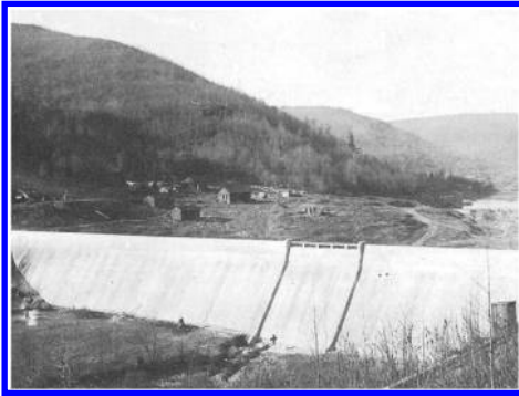
Figure 5. Bayless Dam before failure.
