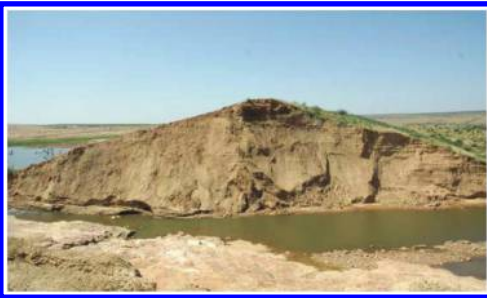
Figure 11. Homogeneous embankment at the breach.
