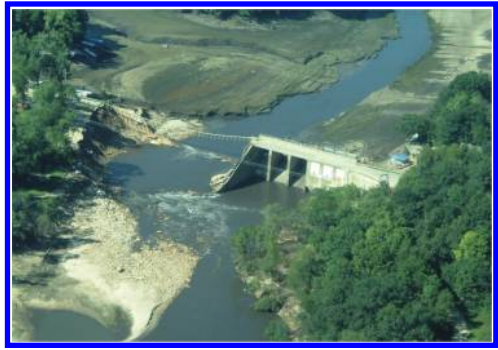
Figure 8. Lake Delhi Dam after failure.
