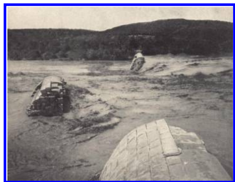
Figure 2. Mc. Donald Dam after failure.
