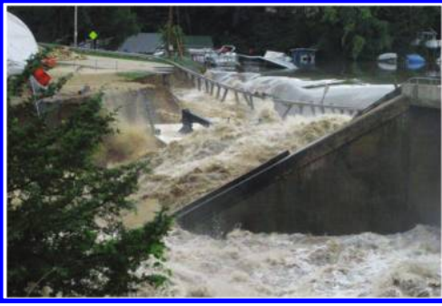
Figure 9. Breach sequence with core wall still in place.
