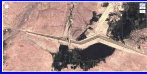
Figure 13. View of failed Gararda Dam.
