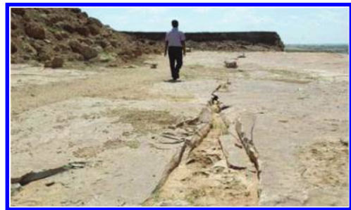
Figure 11. Homogeneous embankment at the breach.
