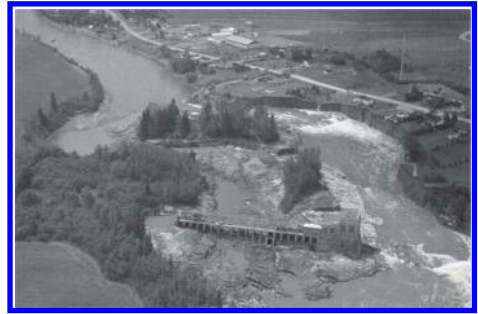
Figure 20. Chute-Garneau Dam after failure.
