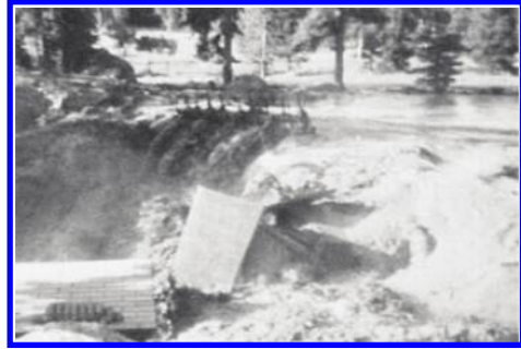
Figure 30. Cascade Dam failure sequence.
