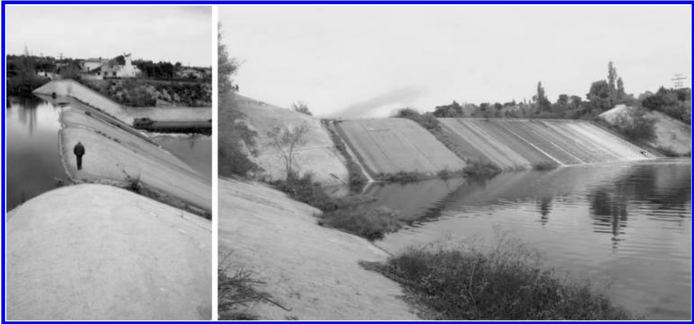
Figure 2. Molino de la Hoz Dam. Left: picture from the right abutment (with Mr. Alfonso Álvarez, designer of the dam, walking on the spillway). Right: picture from the downstream river bank.
