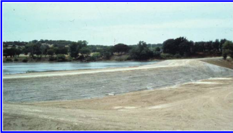
Figure 7. Brownwood Country Club Dam.
