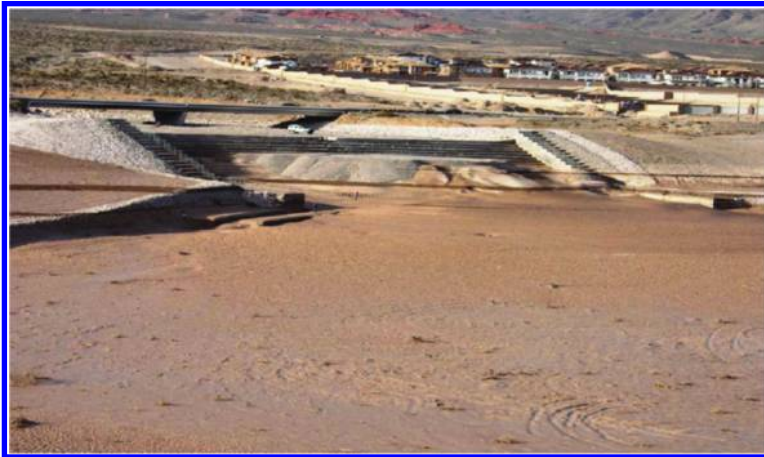
Figure 15. Red Rock RCC inflow spillway (January 2005). Note pile of sediment in stilling basin.
