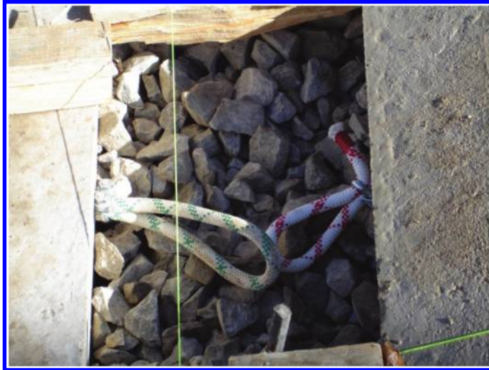
Figure 6. Bedding layer material and cable endings in longitudinal joint.
