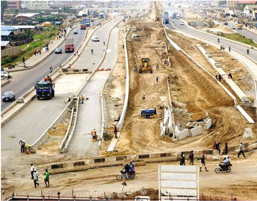
Fig. 8.6 Case Study 1 project site (ongoing work)
