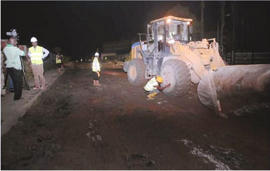
Fig. 8.8 Case Study 2 project site (work being undertaken at night)
