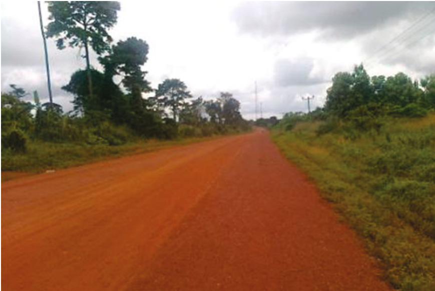
Fig. 8.10 Case Study 3 project site (delayed project)
