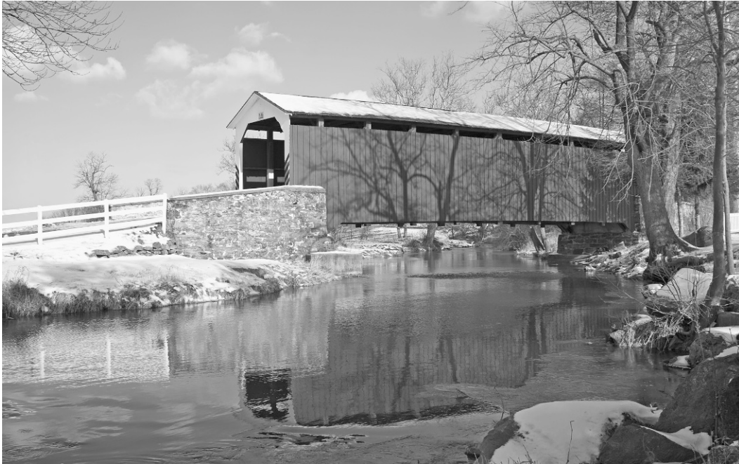
FIGURE 8-1 Historic structures, such as this old covered bridge, are an important part of the existing culture and should be protected. Image acquired from depositphotos.com.
