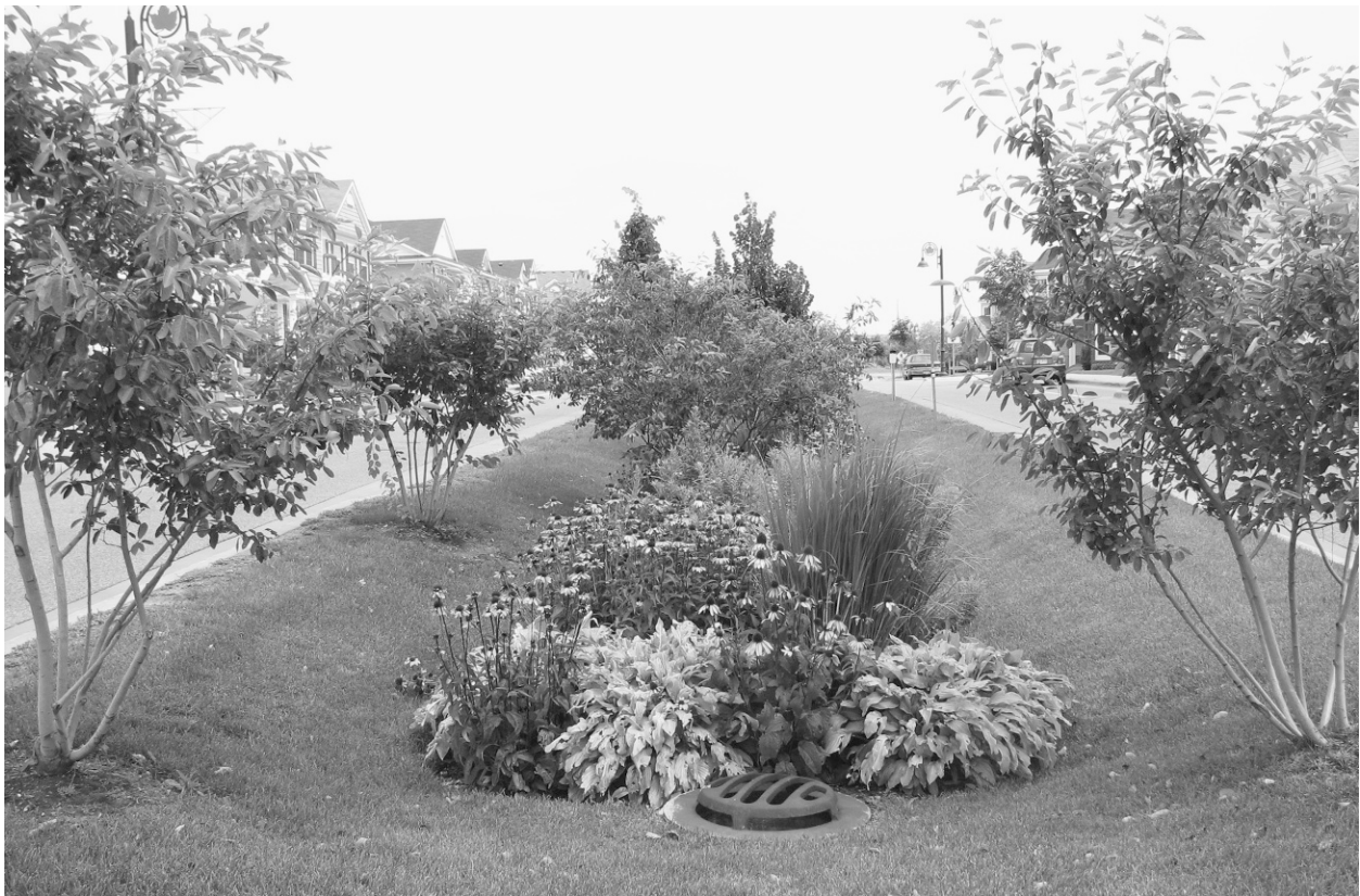
FIGURE 7-14 Rain gardens can be as shallow as four inches deep or as deep as twelve inches. Most rain gardens are simply depressions in the ground, with no need for special soil or pipes. Image courtesy of Jamie Csizmadia.
