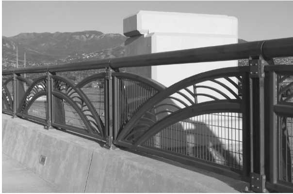
FIGURE 3-27 The ornamental railing on the Legacy Parkway in Utah is designed to enhance the parkway’s surrounding landscape. Photograph by Sharen Hauri, courtesy of National Scenic Byways Online ( www.byways.org ).
