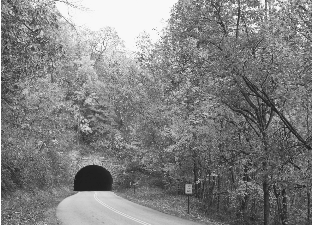
FIGURE 8-34 The Blue Ridge Parkway tunnels, a total of twenty-six, were designed to have a minimal impact on the land. Image courtesy of the Library of Congress-HABS/HAER.
