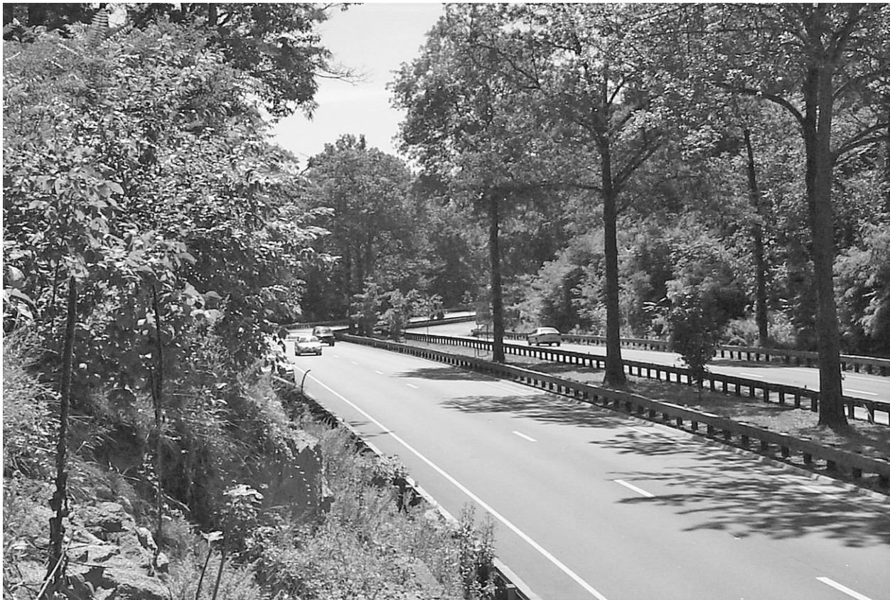
FIGURE 8-24 During construction of the Merritt Parkway in the 1930s, landscape architects attempted to save as many trees as possible from being cut down by creating gently rounding hills along the highway. Image courtesy of Connecticut Department of Transportation.
