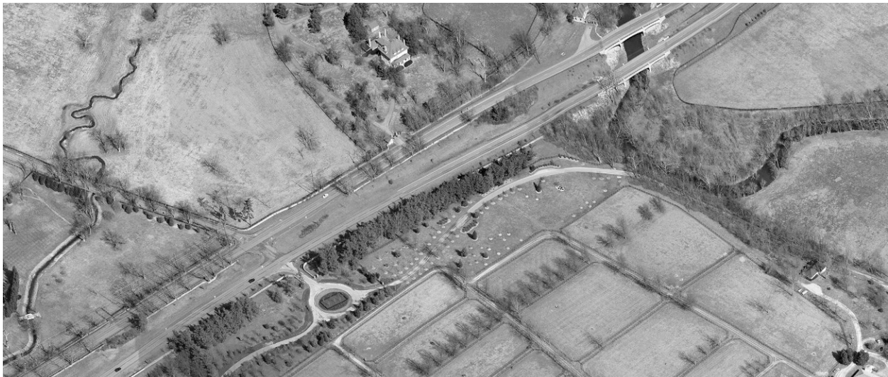
FIGURE 8-21 An aerial view of Paris Pike shows how the north- and southbound lanes move independently of each other, creating a median with variable widths. Image courtesy of J. Sipes.
