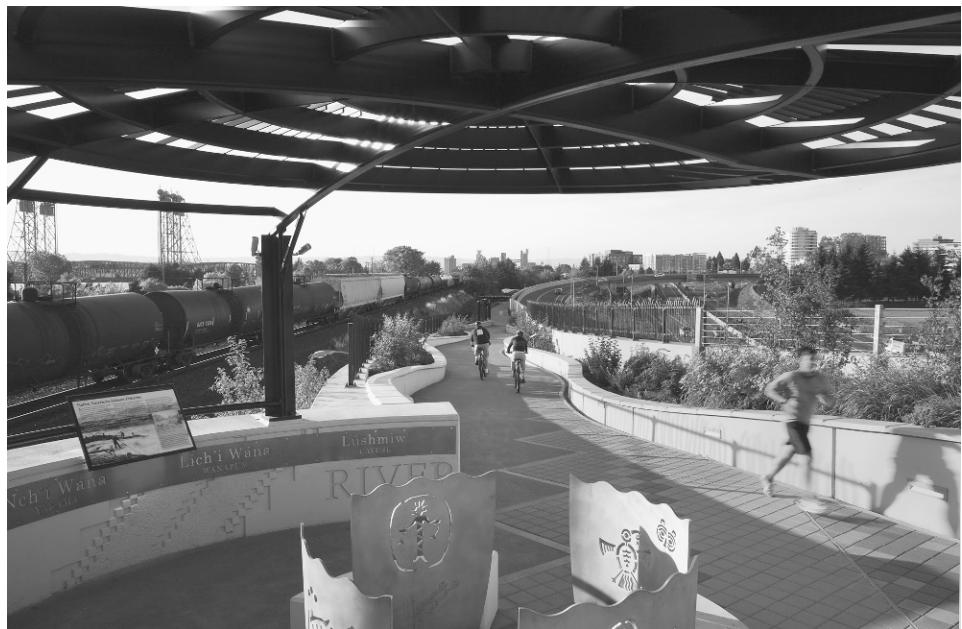
FIGURE 5-7 As bikers and pedestrians cross the Vancouver Land Bridge, they experience what is intended to be a natural extension of the landscape. Image courtesy of Jones & Jones.
