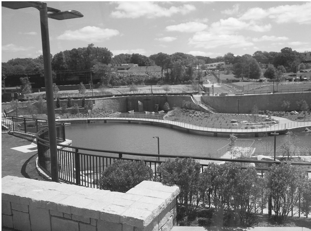
FIGURE 11-5 The seventeen-acre Fort Ward Park, which is one of the first projects constructed as part of the BeltLine, integrates stormwater detention as part of public open space. Image courtesy of EDAAW.
