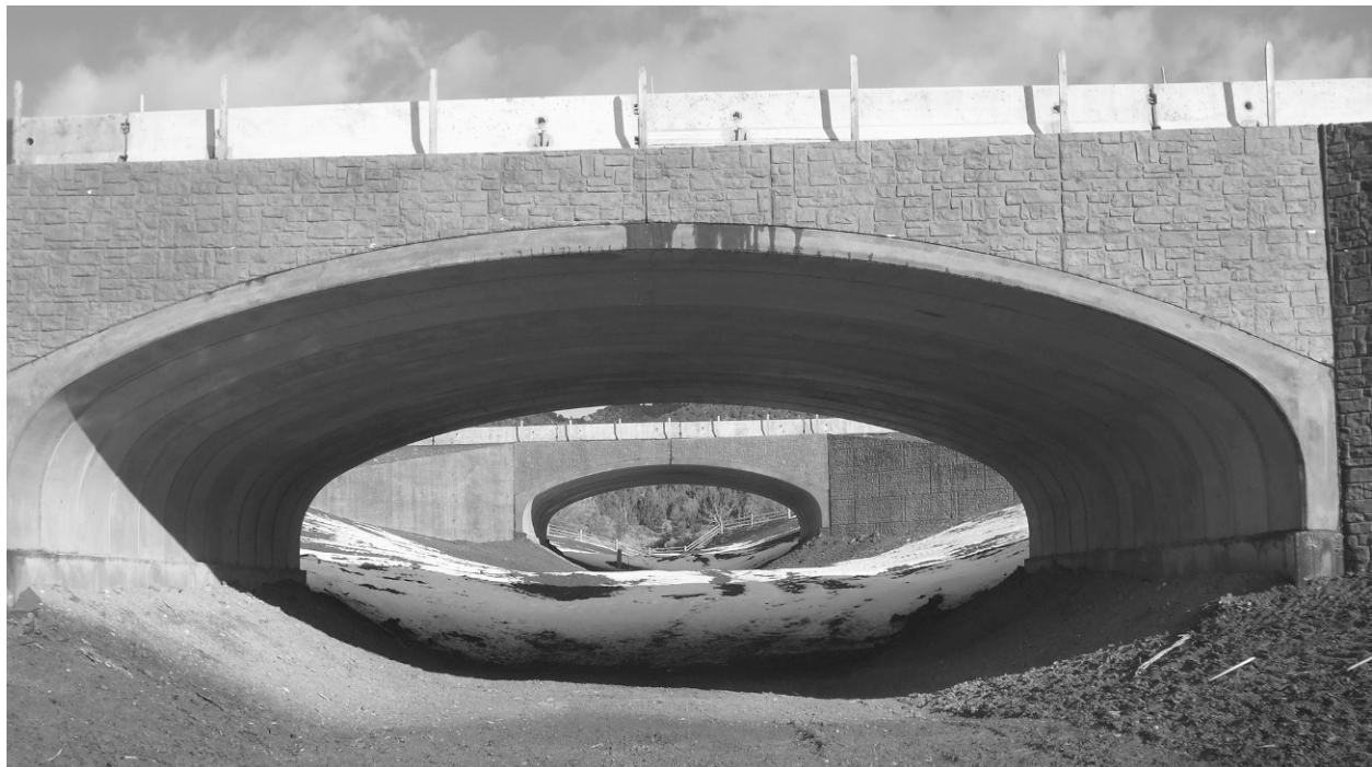
FIGURE 9-1 Wildlife crossings, such as these underpasses in Utah, have proven successful in increasing driver safety as well as animal survival. Image courtesy of Utah Department of Transportation.
