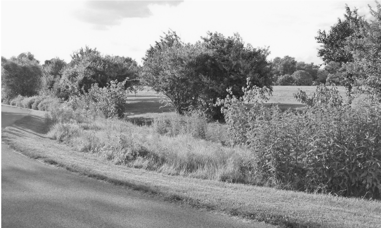
FIGURE 9-12 A bioretention basin is a landscaped depression that directs stormwater into an area where it can be treated by a number of physical, chemical, and biological processes. Image courtesy of EDAW.
