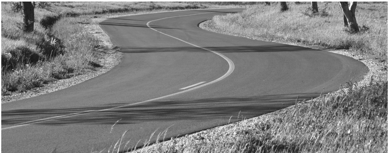
FIGURE 3-12 The gently curving road appears to be carved into the contours of the land, providing a gradual change to the driver, who is met with constantly changing views. Image acquired from depositphotos.com.
