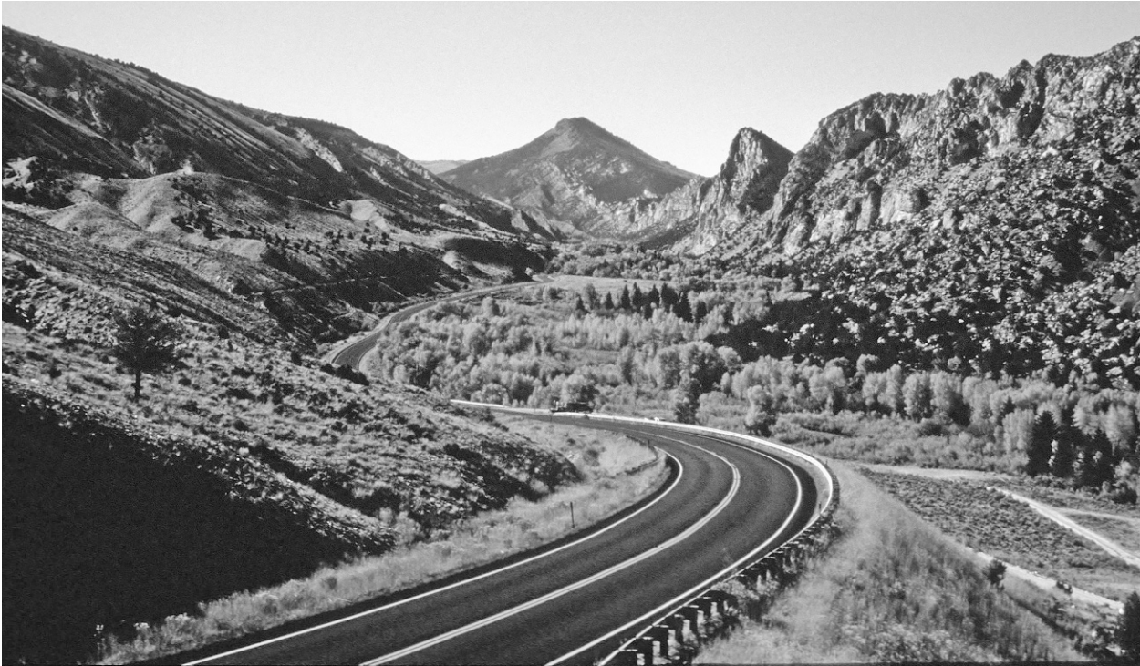
FIGURE 3-2 Looking along US Route 44 south of Manila, Utah, the road follows the base of the mountains to minimize cutting into the slope and stay out of the adjacent river valley. Image courtesy of National Scenic Byways Online ( www.byways.org ).
