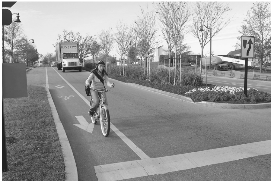
FIGURE 3-37 Bike lanes are a common part of all new roads constructed in Baldwin Park, California. Image courtesy of EDAW.
