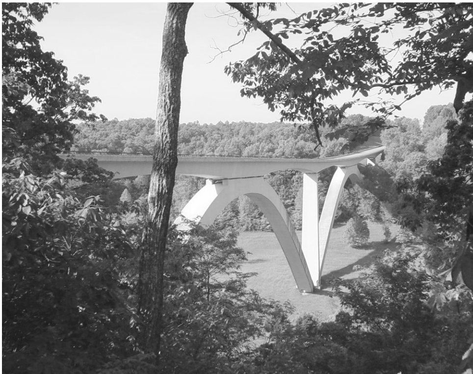
FIGURE 8-36 The Natchez Trace Parkway Bridge, located in Williamson County, Tennessee, is a 1,572-foot-long concrete double arch bridge spanning State Route 96 and a heavily wooded valley. Image courtesy of the National Park Service.
