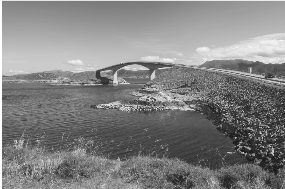
FIGURE 12-22 Norway's Storseisundet Bridge, located along "The Road to Nowhere," is the longest of the eight bridges that make up the Atlantic Road. Image courtesy of Wikipedia Commons.
