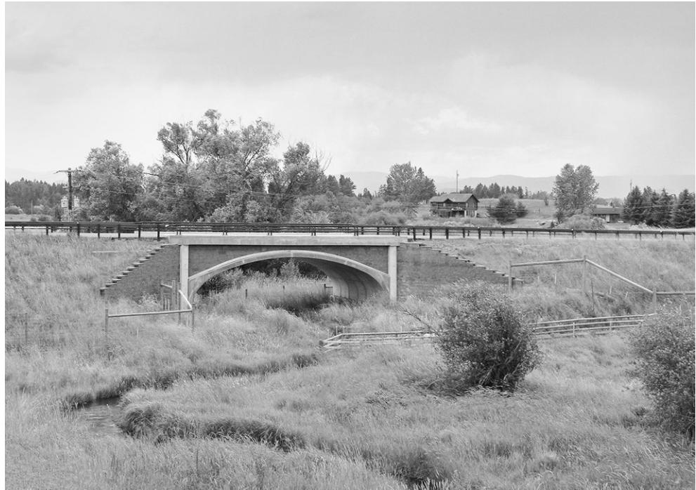
FIGURE 9-23 This bridge structure is wide enough to allow the creek and its adjacent landscape banks to connect from one side of the road to the other. Image courtesy of Jones & Jones.
