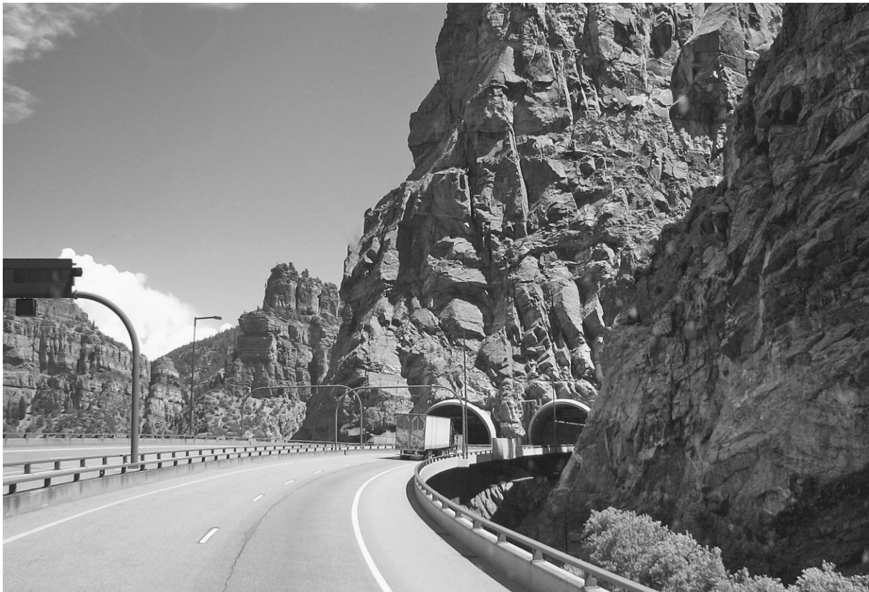
FIGURE 8-18 Approaching the entrance to the Glenwood Hanging Tunnel along I-70 in Colorado, viaducts take I-70 directly into the tunnel portals. Image courtesy of Wikipedia Commons.
