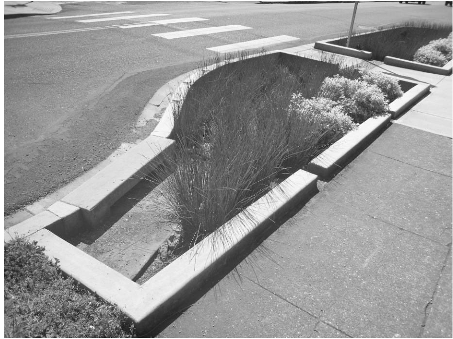
FIGURE 9-11 This bio-swale in Portland, Oregon, is designed to remove silt and pollution from surface and runoff water. Image courtesy of Kevin Robert Perry, City of Portland.
