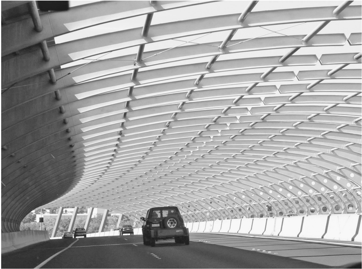
FIGURE 12-1 The Sound Tube that is part of the Tullamarine Freeway in Melbourne, Victoria, Australia, is used to reduce noise pollution to neighboring residential development. Image courtesy of Wikipedia Commons.
