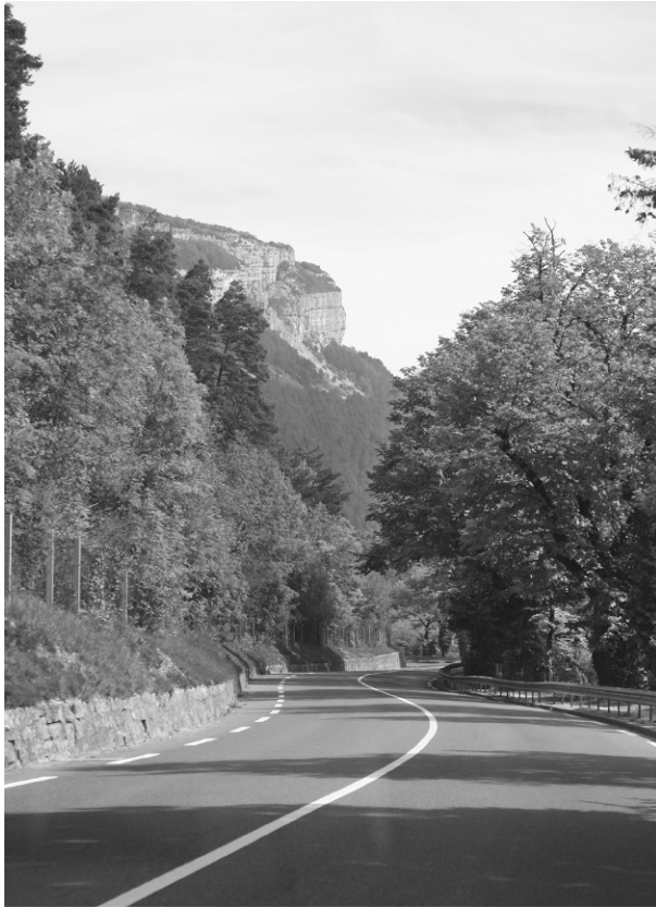
FIGURE 8-11 A stone retaining wall along the side of the road minimizes impacts to adjacent natural resources. Image acquired from depositphotos.com.
