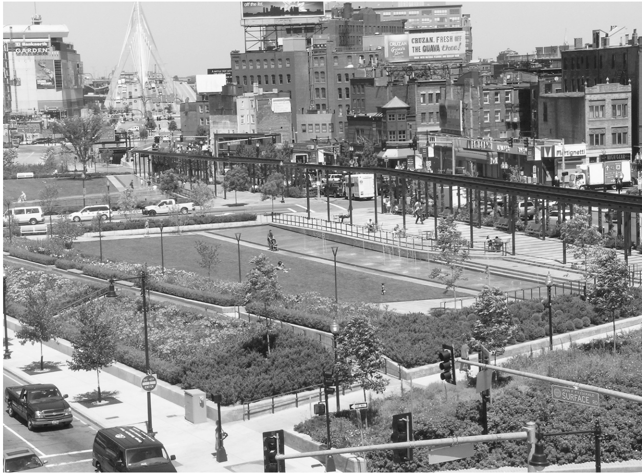
FIGURE 6-13 Boston's Big Dig reconstruction replaced part of the highway with a mile-long green space, including benches, fountains, and trees. Image courtesy of Wikipedia Commons.
