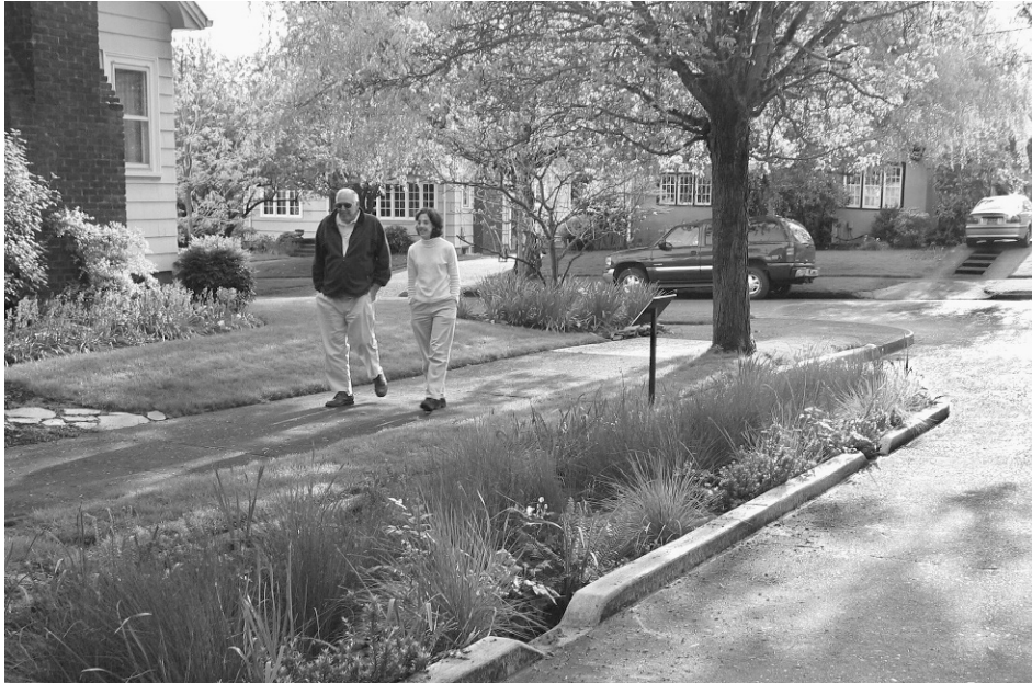
FIGURE 6-7 The Northeast Siskiyou Green Street curb extensions include a series of miniature dams. Water cascades from one “cell” to another. The system can manage 225,000 gallons of stormwater runoff per year. Image courtesy of Kevin Robert Perry, City of Portland.
