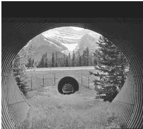
FIGURE 9-21 Using natural vegetation for the floor of the wildlife crossings can help make the underpasses more welcoming and more appealing for animals to use. Image courtesy of Jones & Jones.
