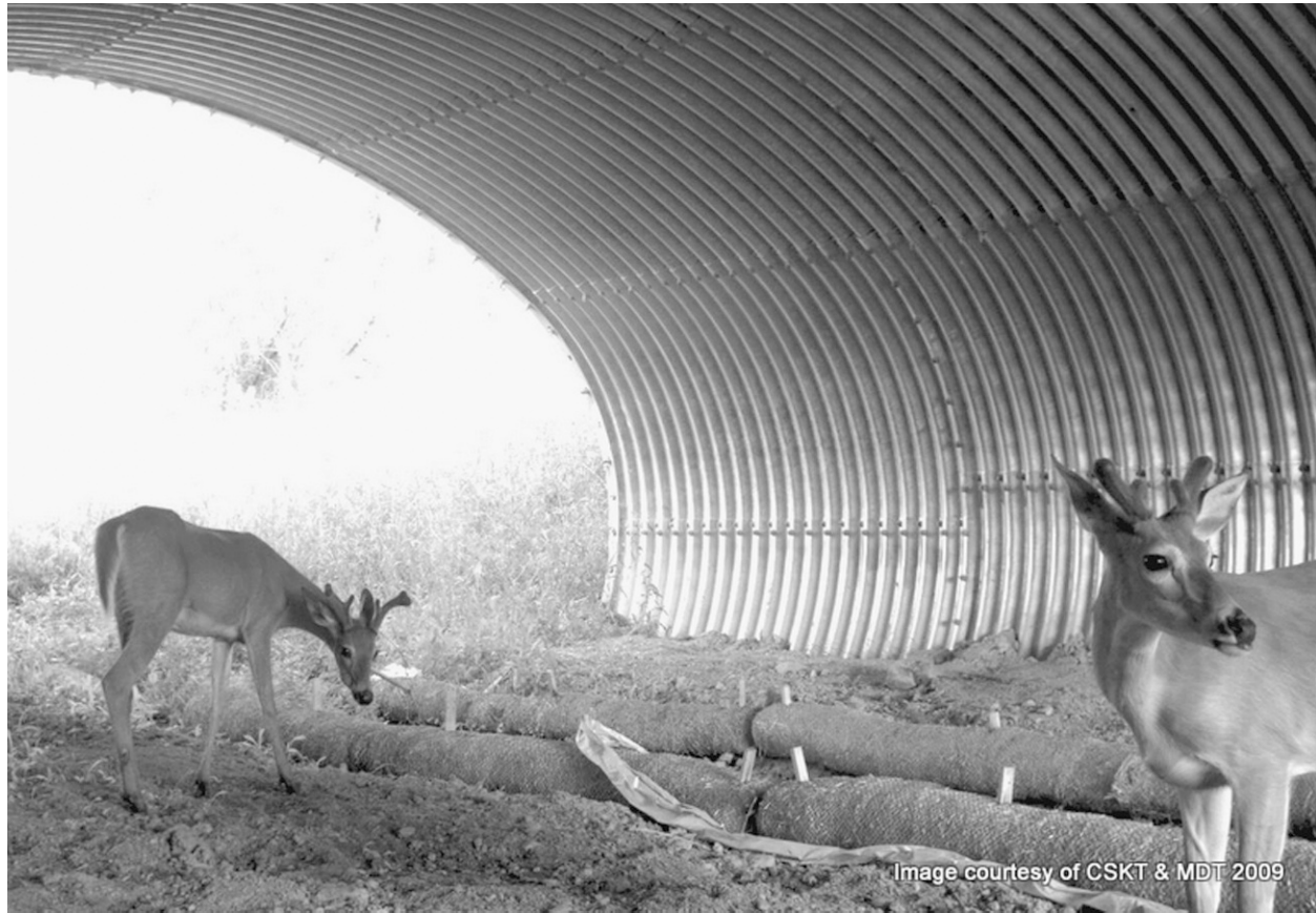
FIGURE 9-5 Deer can safely cross US Highway 93 that might otherwise interfere with their normal migration route. It is important to make the tunnels as wide as possible with a dirt and rock floor. Image courtesy of Montana Department of Transportation.
