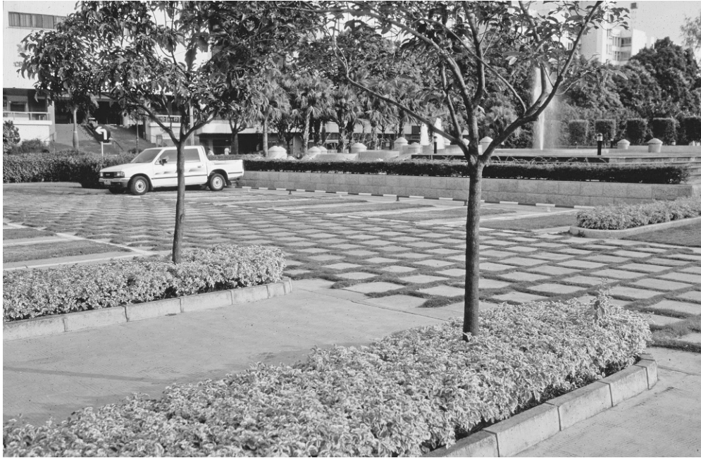
FIGURE 3-43 Using a green approach to parking areas, such as this one in Shekou, China, allows rainwater to drain through the pavement, thus reducing pollution. Image courtesy of EDAW.
