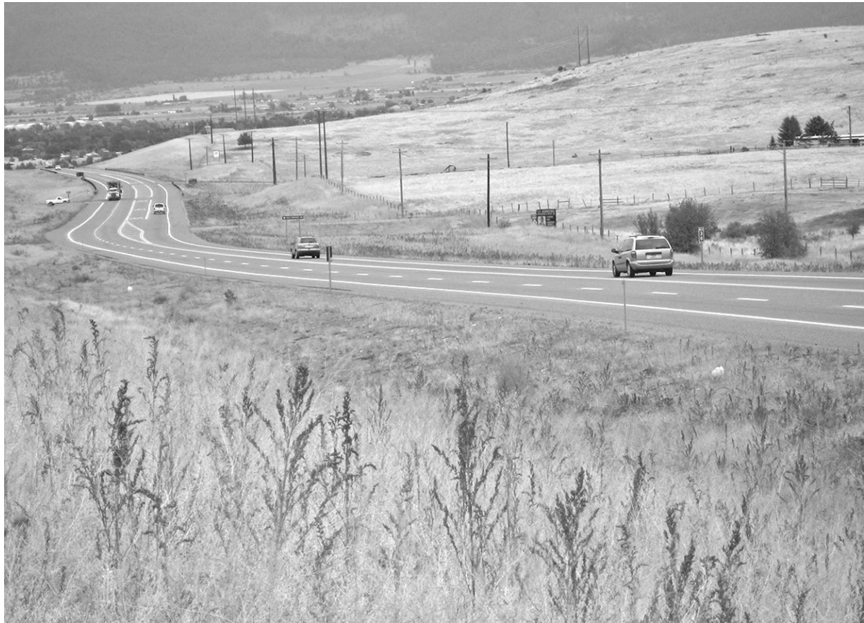
FIGURE 9-20 US 93 enters Montana from Idaho, continues north through Flathead National Forest, then reaches its end at the Canadian border. Image courtesy of Jones & Jones.
