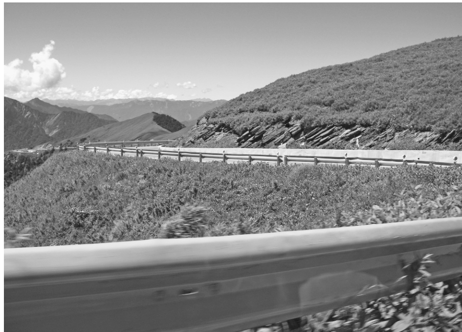
FIGURE 3-22 The Hehuan Road leads to the top of Hehuan Mountain in central Taiwan. Colorful red and yellow guardrails are used to make the narrow, winding road safer, while also adding visual interest. Image courtesy of AECOM.
