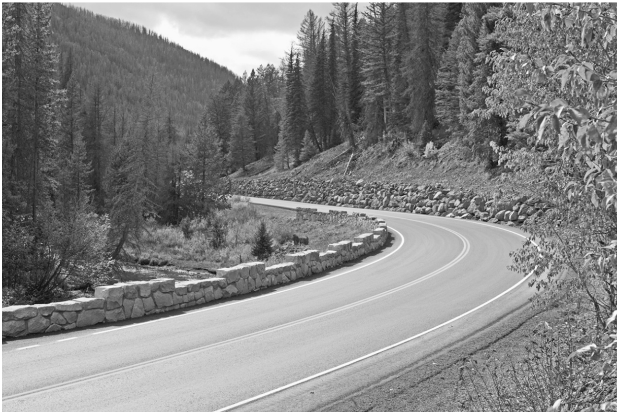
FIGURE 9-31 The east entrance to Yellowstone National Park climbs over Sylvan Pass and descends to Yellowstone Lake. Image courtesy of FHWA.
