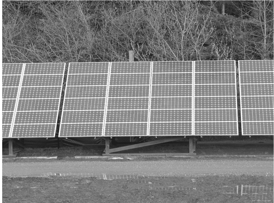
FIGURE 12-11 The 594 solar panels located with the right-of-way of the Oregon Solar highway produce nearly 130,000 kilowatt hours of electricity annually. Image courtesy of Oregon Department of Transportation.
