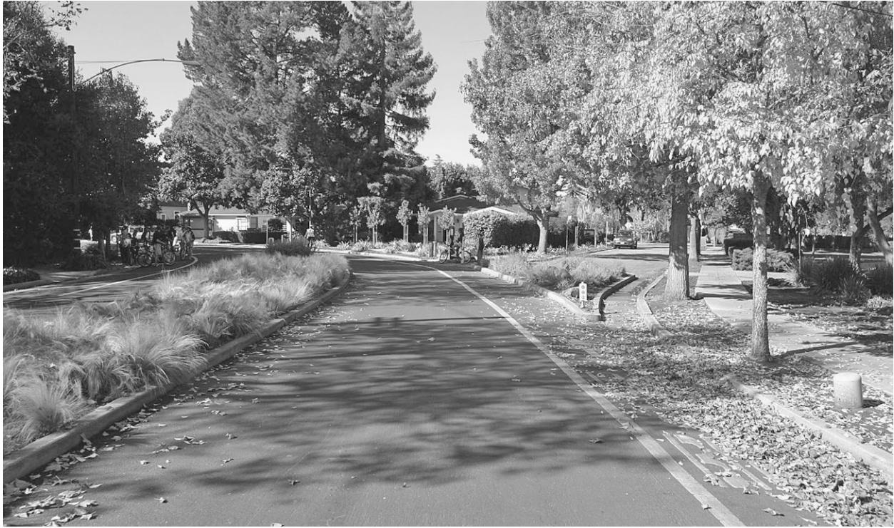
FIGURE 7-7 Planted medians, narrow travel lanes, and adjacent bike lanes help reduce the impact of roadways. Image courtesy of EDAAW.
