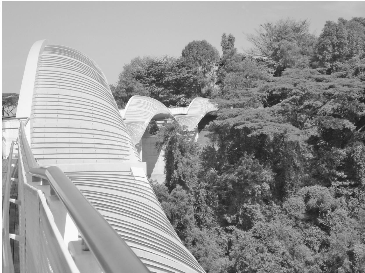
FIGURE 12-14 The Henderson Waves Bridge in Singapore is designed with seven undulating curved steel “ribs” that alternately rise over and under its deck. The unique waveform of the bridge gives it a distinct look. Image courtesy of Wikipedia Commons.
