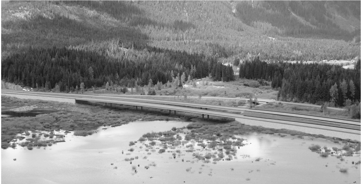
FIGURE 9-3 The wildlife underpass at Gold Creek in Washington State not only benefits the local terrestrial wildlife, but also benefits the animals living in the creek. Image courtesy of Washington State Department of Transportation.
