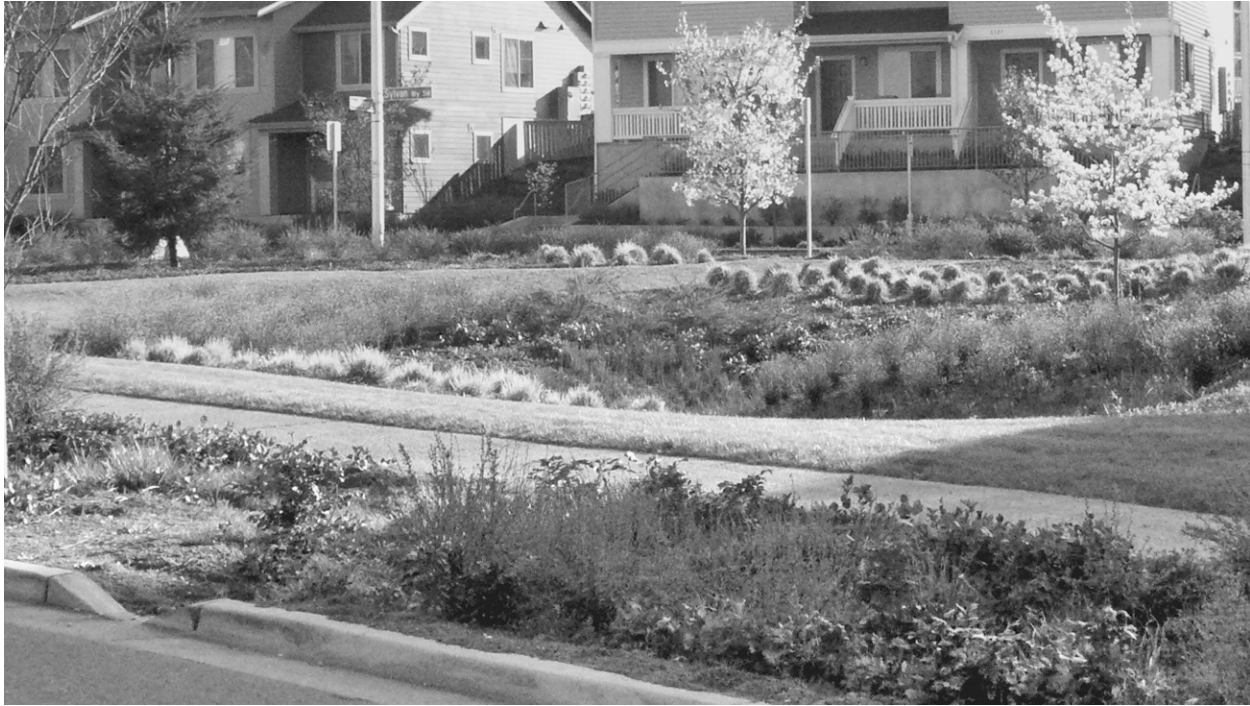
FIGURE 7-16 One example of a sustainable feature in High Point's redeveloped community is the use of rain gardens. This design allows more stormwater to soak into the ground, thereby reducing pollution. Image courtesy of Wikipedia Commons.
