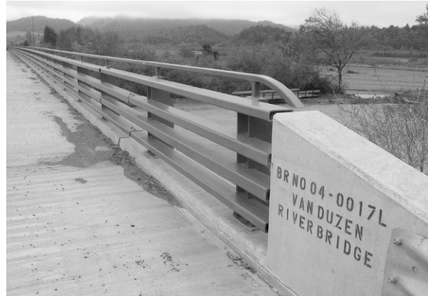
FIGURE 3-28 Open-spandrel bridges, like the Van Duzen River Bridge in Humboldt County, California, are designed to leave more areas of the rail open. Image courtesy of Dr. Ronald K. Faller, from Online Guide To Bridge Railings ( guides.roadsafellc.com/bridgeRailGuide/index.php ).
