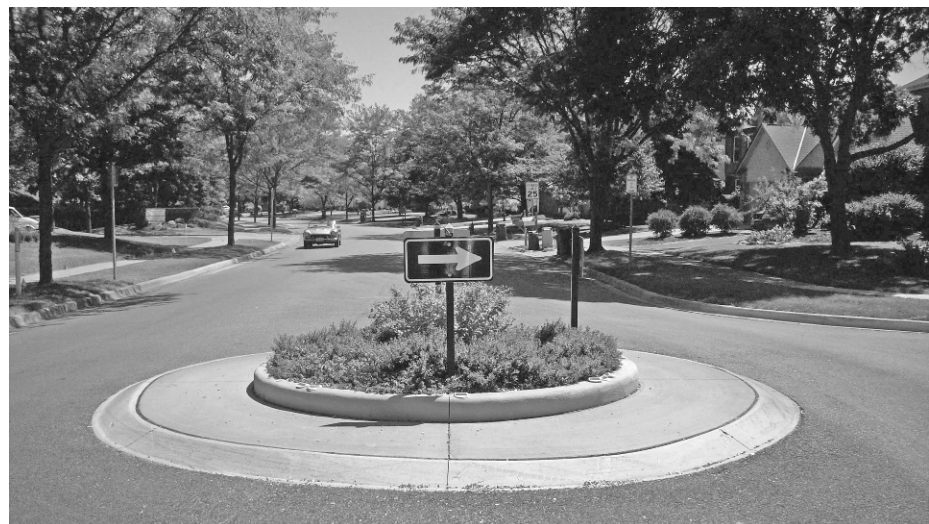
FIGURE 3-15 This traffic circle in Dublin, Ohio, was successful in both decreasing the average speed of traffic and decreasing the volume of traffic along Tara Hill Drive. Image courtesy of Heather Bowden.
