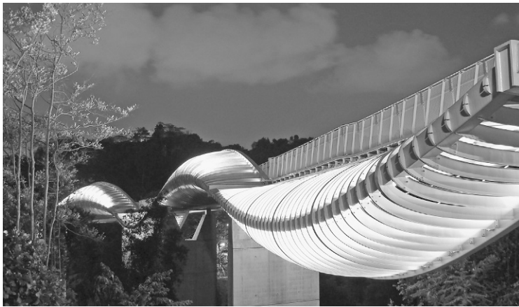
FIGURE 12-15 The lighting for the Henderson Waves Bridge helps enhance the visual character of the bridge at night. Image courtesy of Wikipedia Commons.
