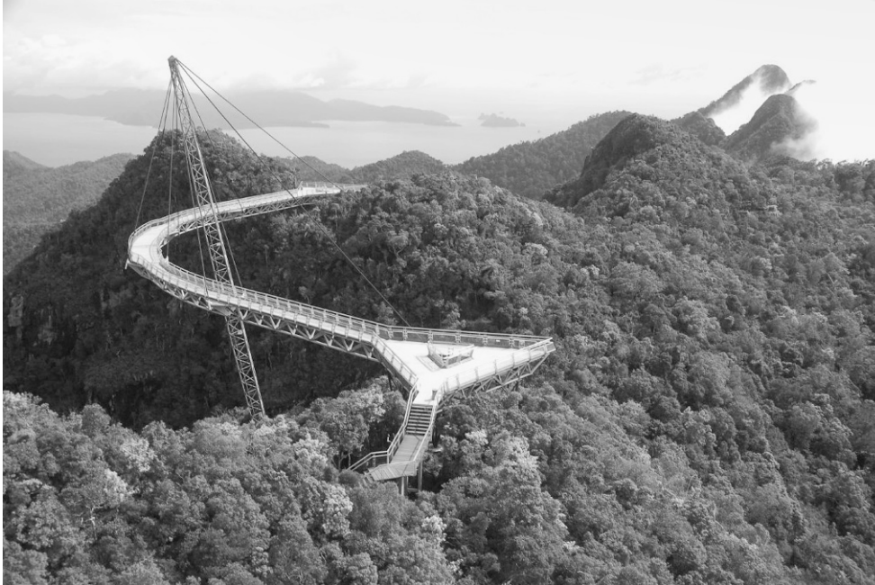
FIGURE 10-2 Langkawi Sky Bridge is a curved pedestrian cable-stayed bridge in Malaysia. It is located 2,297 feet above sea level at the peak of Gunung Mat Chinchang. Image courtesy of Wikipedia Commons.
