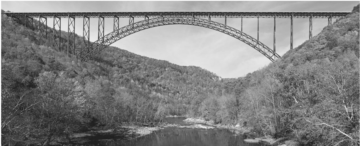
FIGURE 10-8 The New River Gorge Bridge is the fifth highest vehicle bridge in the world, sitting 876 feet above the New River. Image courtesy of Wikipedia Commons.
