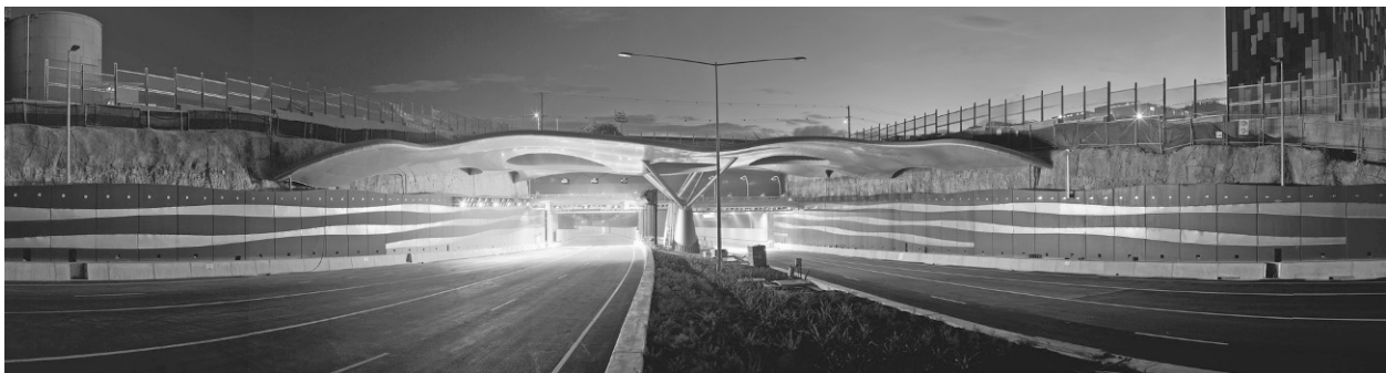
FIGURE 12-17 The CLEM7 Tunnel at dusk, Brisbane, Australia. Image courtesy of RiverCity Motorway.
