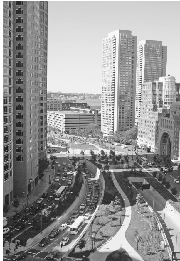
FIGURE 6-12 The Big Dig was a project in Boston that rerouted I-93 into a 3.5-mile tunnel. The project was created in response to Boston's heavily congested streets. Image courtesy of Wikipedia Commons.
