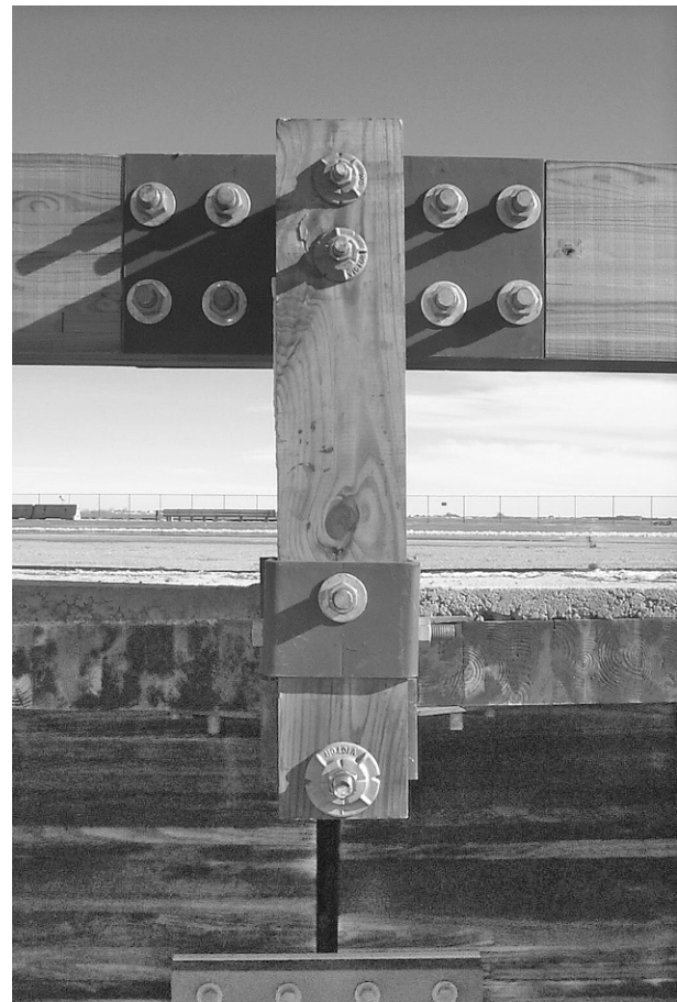
FIGURE 3-26 Glulam Timber is ideal for creating bridges and waterfront structures. Its ability to absorb impact forces from traffic makes it frequently used for highway and railway bridges. Image courtesy of Dr. Ronald K. Faller, from Online Guide To Bridge Railings ( guides.roadsafellc.com/bridgeRailGuide/index.php ).
