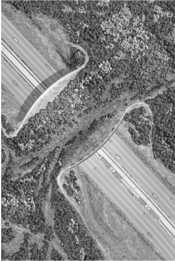
FIGURE 9-32 Olin Partnership’s Wild (X)ing includes a bridge with a concave shape with the lowest point in the center of the crossing. Image courtesy of Olin Partnership.
