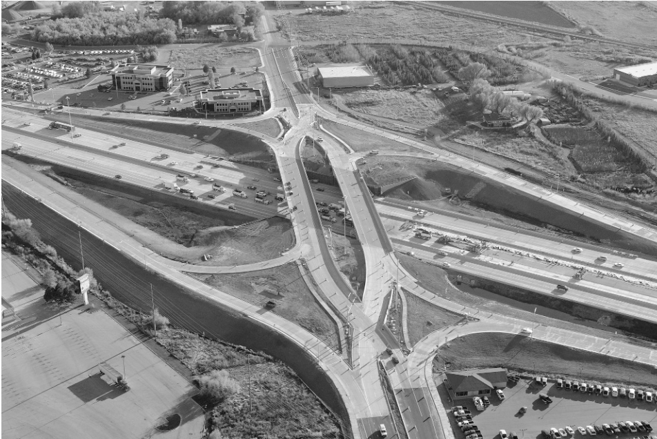
FIGURE 3-18 This diverging diamond interchange is part of Utah Department of Transportation's I-15 Corridor Expansion Project. Image courtesy of Utah Department of Transportation.
