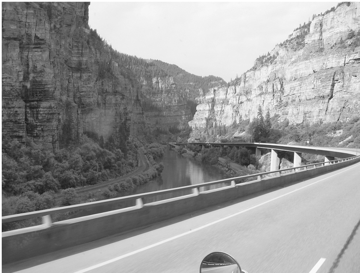
FIGURE 8-19 The westbound road to Hanging Lake Tunnel, along Glenwood Canyon, is positioned on a high viaduct, providing travelers with a good view. Image courtesy of Wikipedia Commons.
