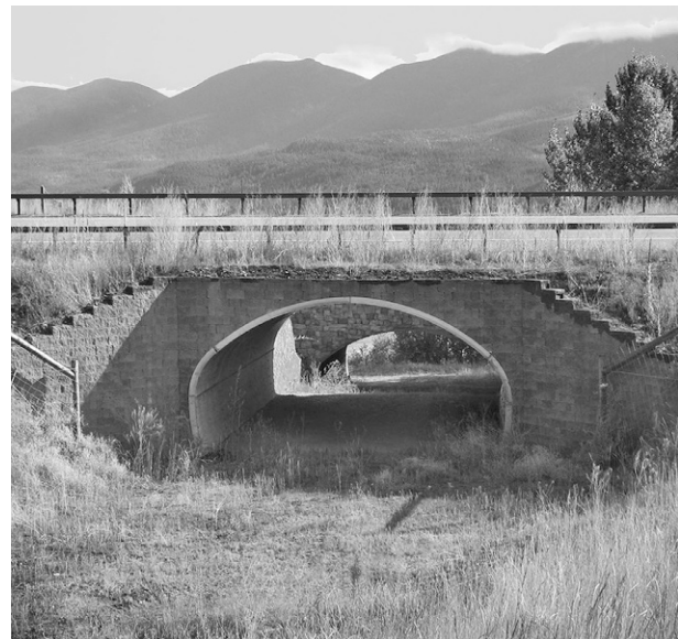
FIGURE 9-22 It is sometimes helpful to use fencing to guide the animals toward the opening of the wildlife crossings. Image courtesy of Jones & Jones.
