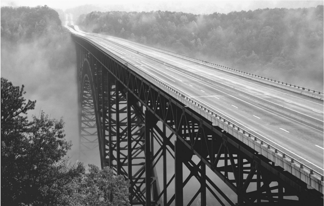
FIGURE 2-1 The New River Gorge Bridge in Fayetteville, West Virginia, was completed in 1978. One of the largest arch bridges in the world, it is an icon and symbol of pride to the people of West Virginia. Photograph by Steve Shaluta, courtesy of National Scenic Byways Online ( www.byways.org ).
