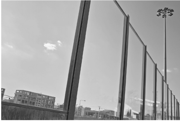
FIGURE 3-20 One major problem with sound walls is that they visually block views and create an enclosed corridor. One solution is to use Plexiglas sound walls that still provide the functionality without creating a visual barrier. Image acquired from depositphotos.com.
