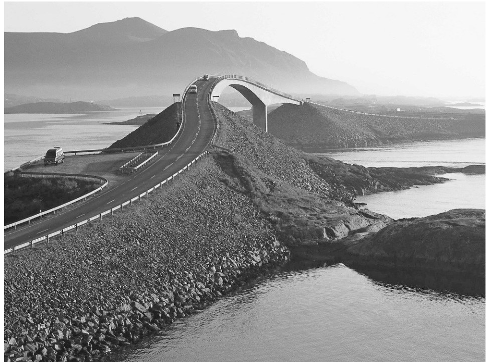
FIGURE 12-23 The Storseisundet Bridge is built so that, as you approach certain angles, it looks as if you may plummet off its seventy-five-foot height. Image courtesy of Wikipedia Commons.
