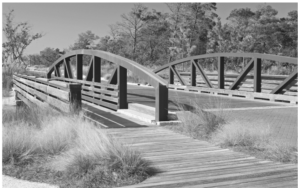
FIGURE 3-33 At the Watersound development in Florida, emphasis is on walkability. Bridges and walkways are constructed at a pedestrian scale. Image courtesy of EDAW.
