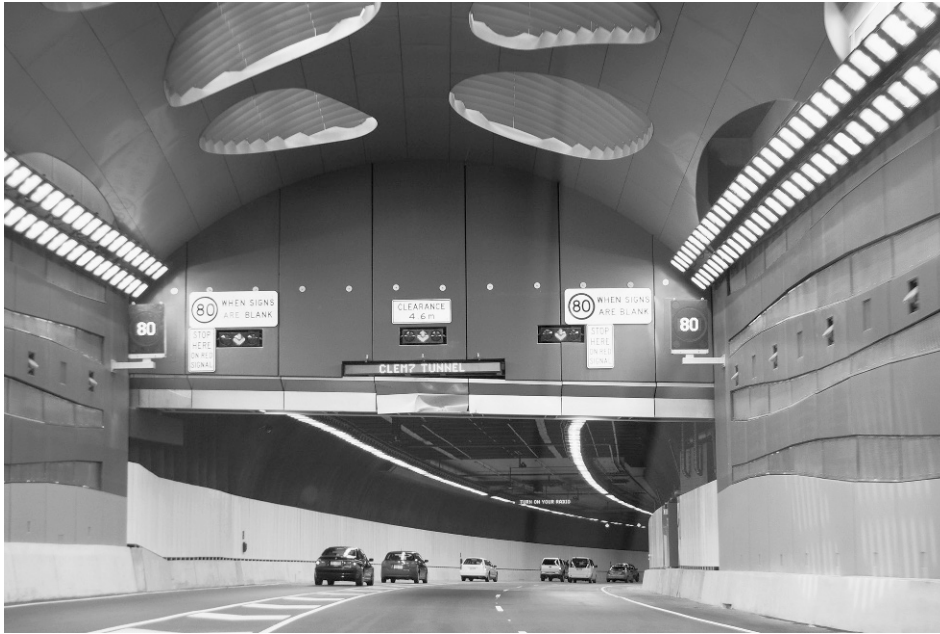
FIGURE 12-18 The CLEM7 Tunnel, built 197 feet below the Brisbane River, uses state-of-the-art monitoring to ensure the safety of passengers. Image courtesy of Shannon Walker.
