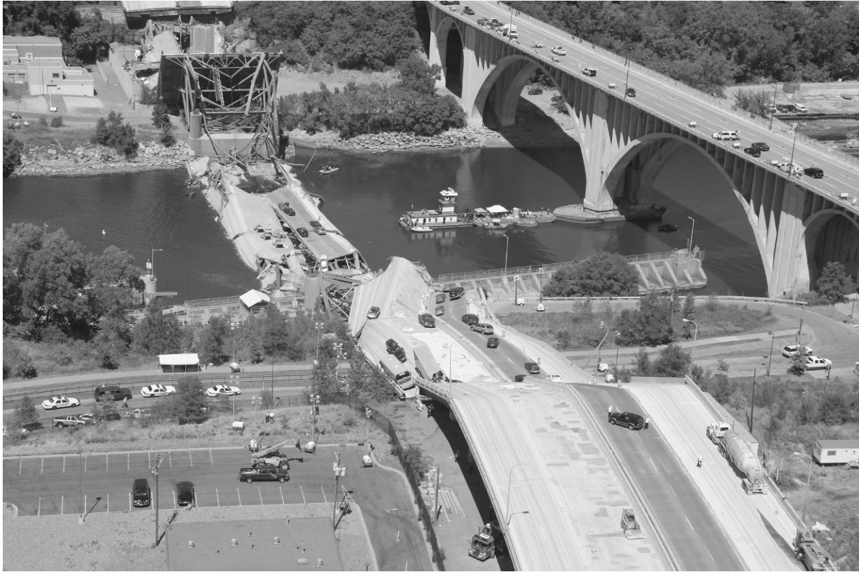
FIGURE 1-5 The collapse of the I-35W Mississippi River Bridge in 2007 was a wake-up call about the need to maintain highway infrastructure in this country. Image courtesy of Minnesota Department of Transportation.
