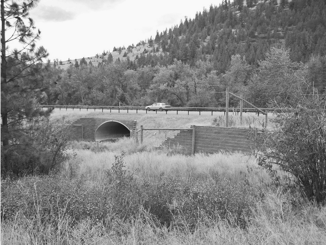
FIGURE 9-6 Natural vegetation near the opening of a wildlife crossing will give animals the security of their preferred environment and can work as a guide to motivate them to use the crossing. Image courtesy of Jones & Jones.
