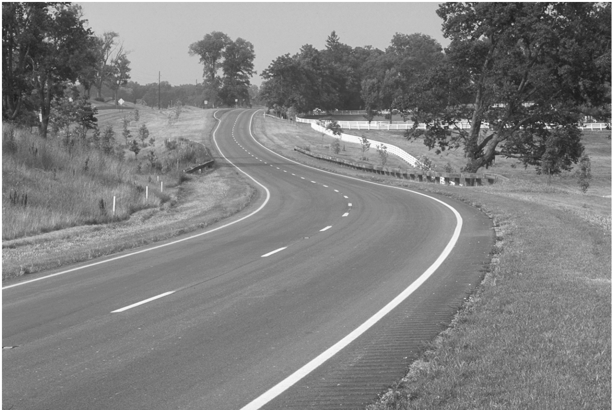
FIGURE 8-20 Care was taken during the widening project of Paris Pike in 1997 to preserve the existing rock walls and entryways and to let the highway flow with the contours of the landscape. Image courtesy of Jones & Jones.
