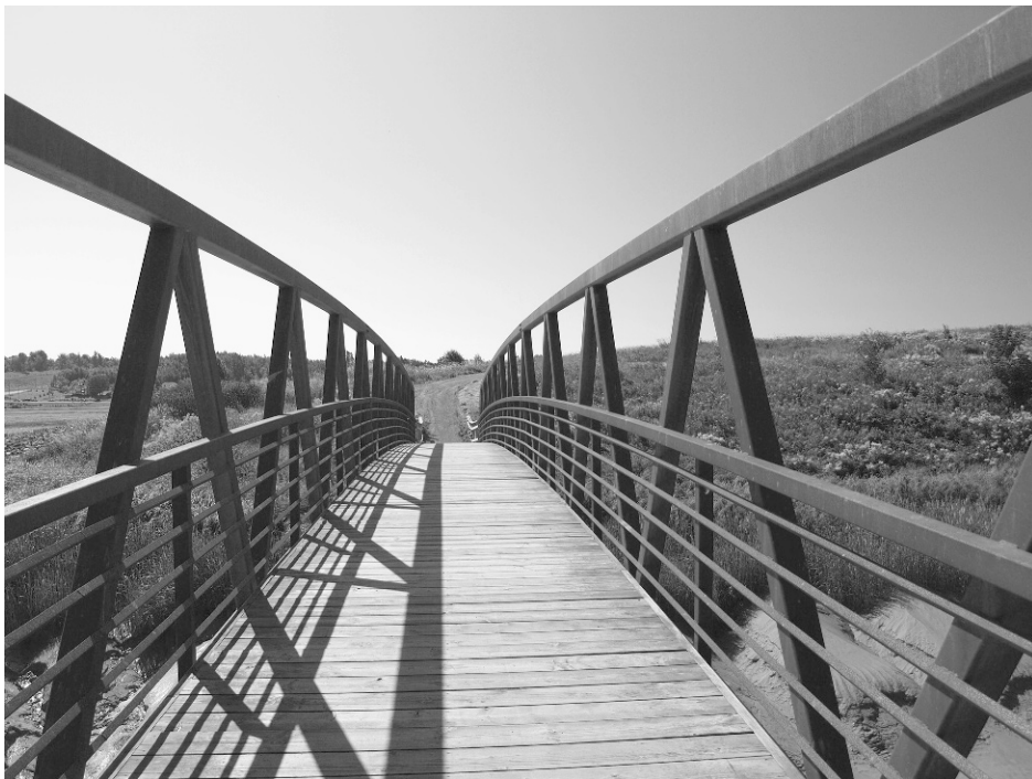
FIGURE 4-5 Simple corten steel pedestrian bridges are an inexpensive way to enhance connectivity to trails and recreation opportunities. Image acquired from depositphotos.com .
