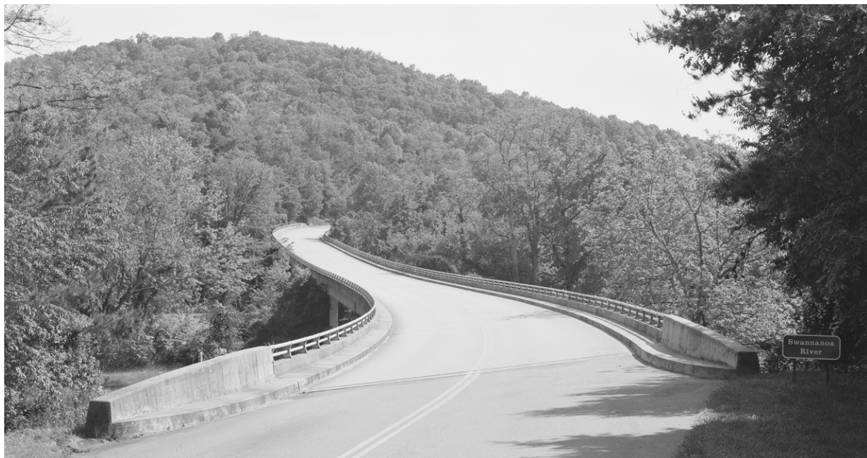
FIGURE 3-5 The Swannanoa River Bridge is a concrete box girder bridge that was built in 1966. Located in North Carolina, it crosses the Swannanoa River and Interstate 40. Image courtesy of the Library of Congress-HABS/HAER.
