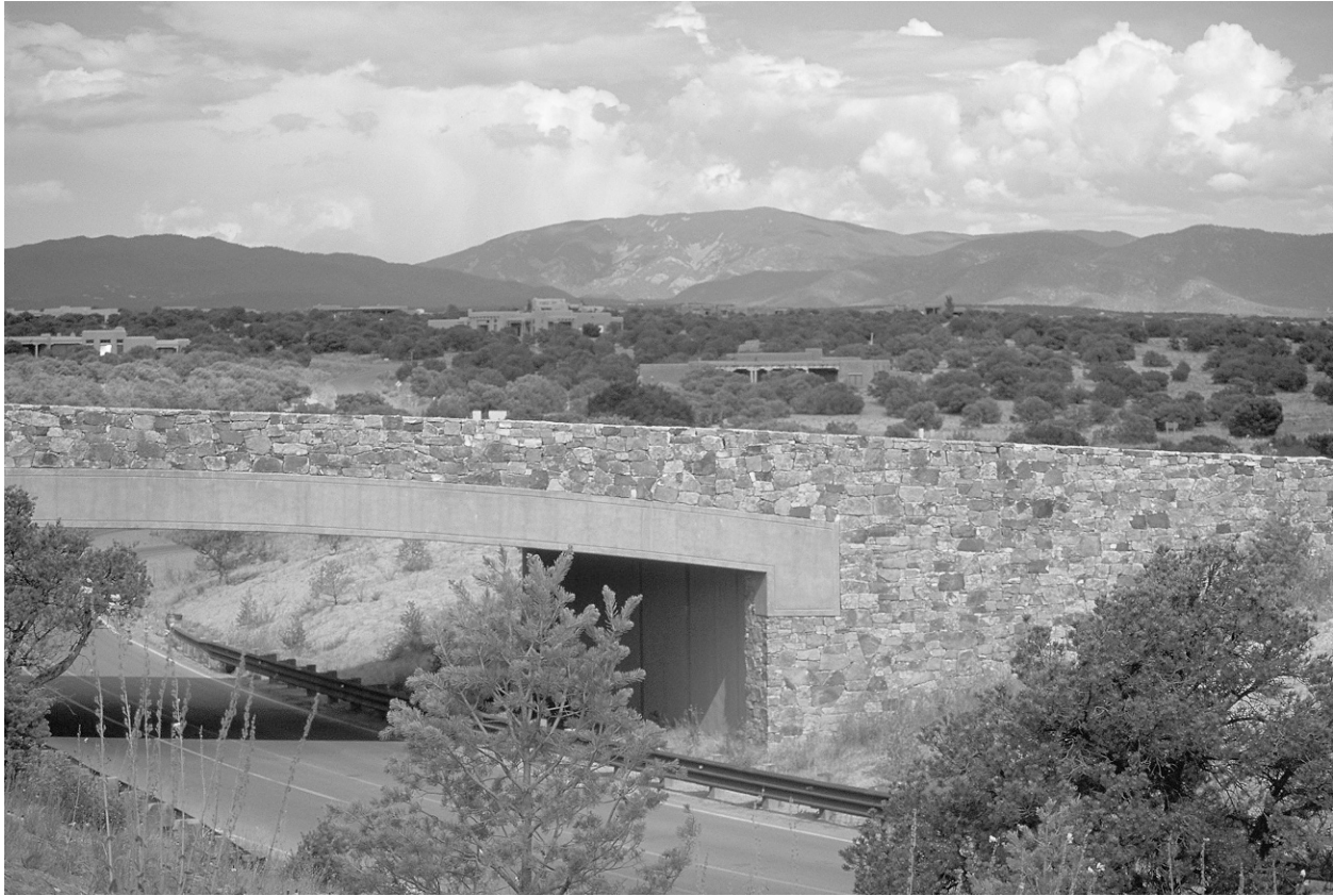
FIGURE 2-3 This bridge in New Mexico uses native stones, a low horizontal design, and subdued brown and tan colors to help visually integrate into the surrounding landscape. Image courtesy of EDAW.
