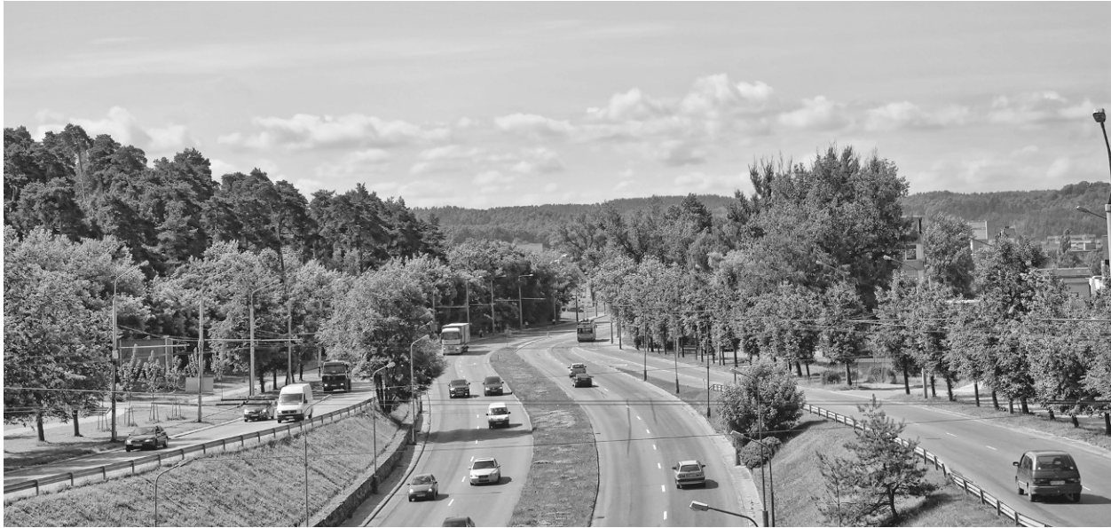
FIGURE 1-1 Using landscape medians, preserving existing vegetation, and planting new trees helps reduce the visual impact of roadways. Image acquired from depositphotos.com.
