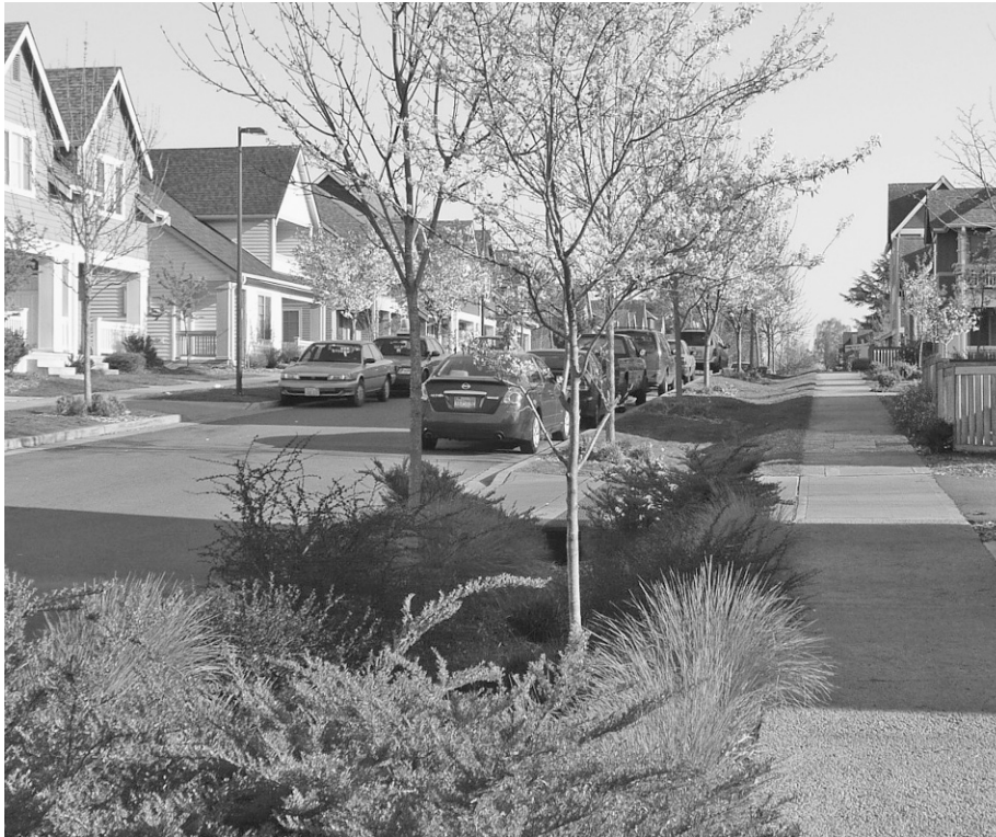
FIGURE 7-15 The redevelopment of High Point in Seattle features the only porous pavement in Washington State. Image courtesy of Wikipedia Commons.
