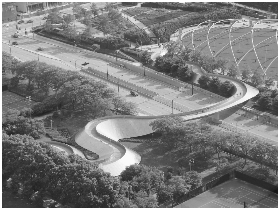
FIGURE 3-30 The BP Pedestrian Bridge in Chicago is a 925-foot bridge that connects Millennium Park to Daley Bicentennial Plaza. Designed by Frank Gehry, the bridge has won awards for its use of sheet metal and is known for its style and aesthetics. Image courtesy of Wikipedia Commons.
