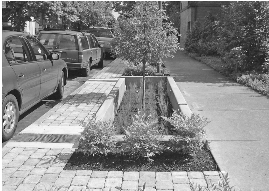
FIGURE 3-42 A bioswale, like this one along 12th Avenue in Portland, Oregon, is used to reduce runoff volumes by slowing down water through vegetation. Image courtesy of Kevin Robert Perry, City of Portland.
