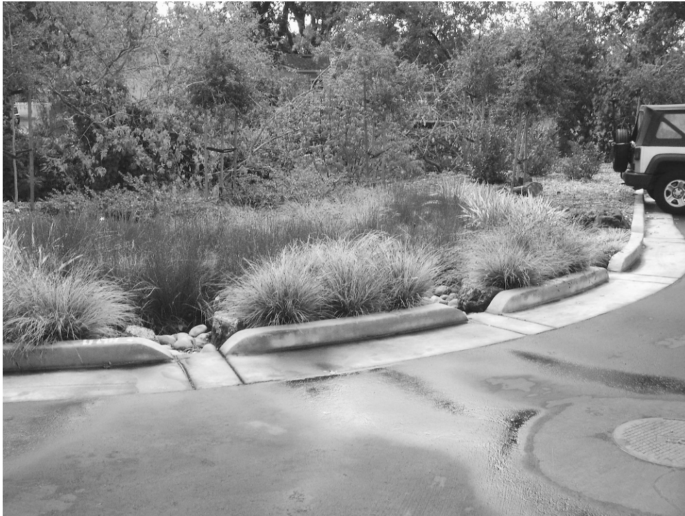
FIGURE 3-8 Rain gardens, like this one in Portland, Oregon, are used for stormwater management. They allow rainwater to soak into the ground instead of running into storm drains or surface water. Image courtesy of the City of Portland.
