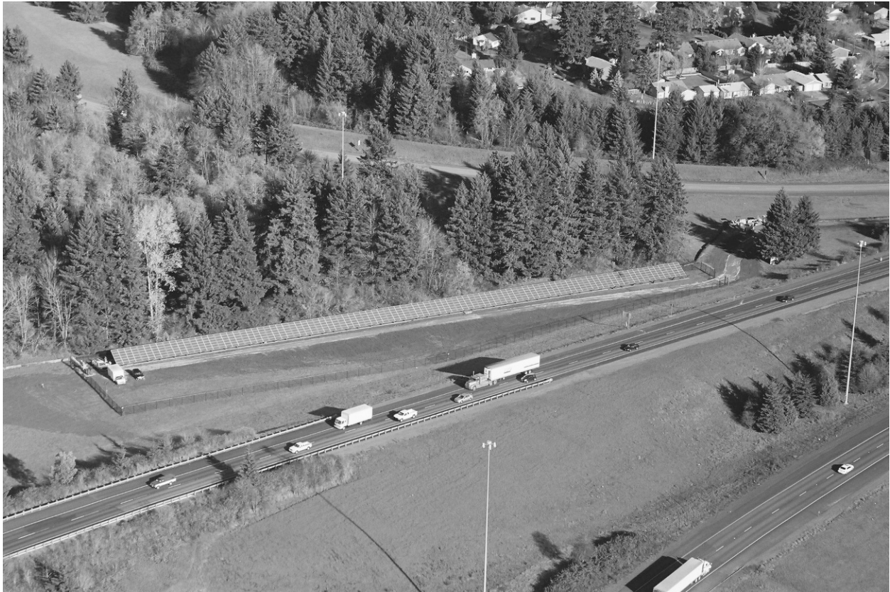
FIGURE 12-10 The solar panels run parallel to the highway near the interchange of I-5 and I-205, and are located so their visual impact is limited. Image courtesy of Oregon Department of Transportation.
