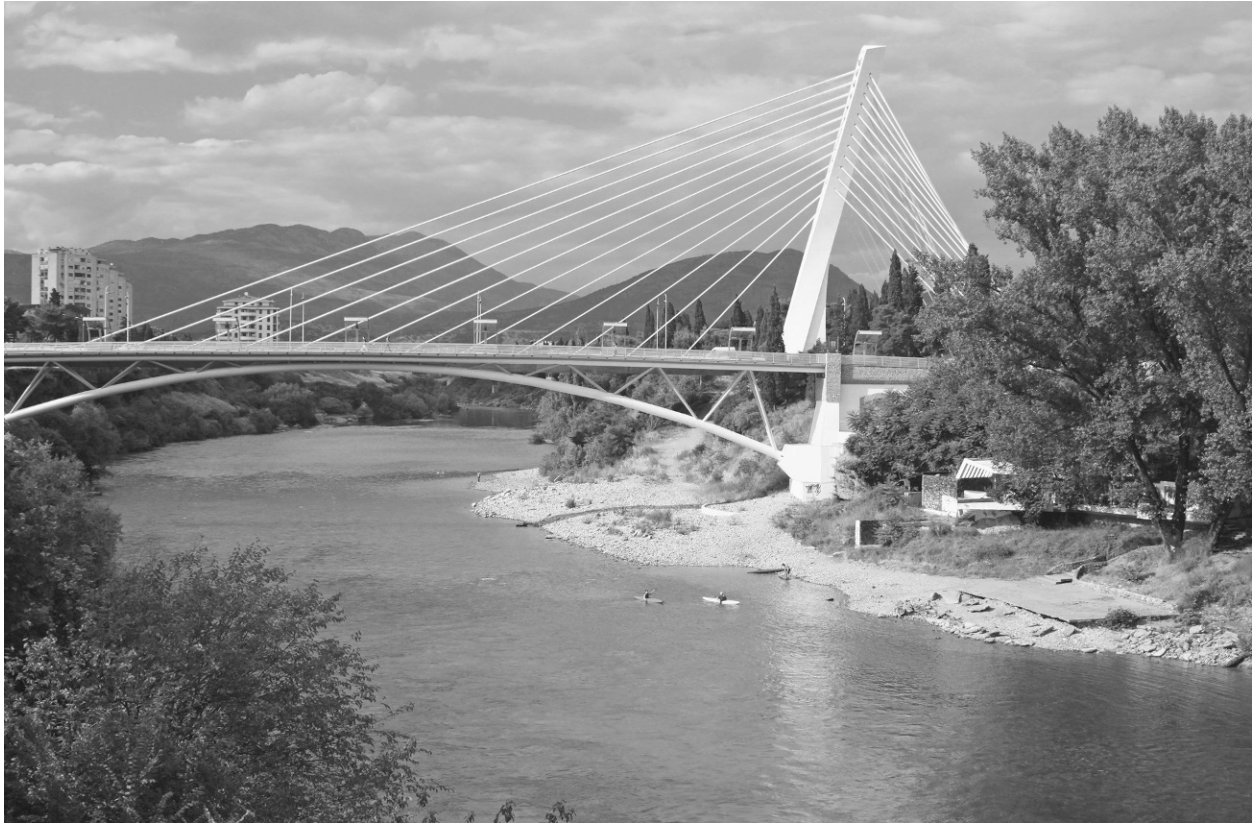
FIGURE 3-25 The Millennium Bridge is a cable-stayed bridge that spans the Moraca River in Podgorica, Montenegro. Image acquired from depositphotos.com.
