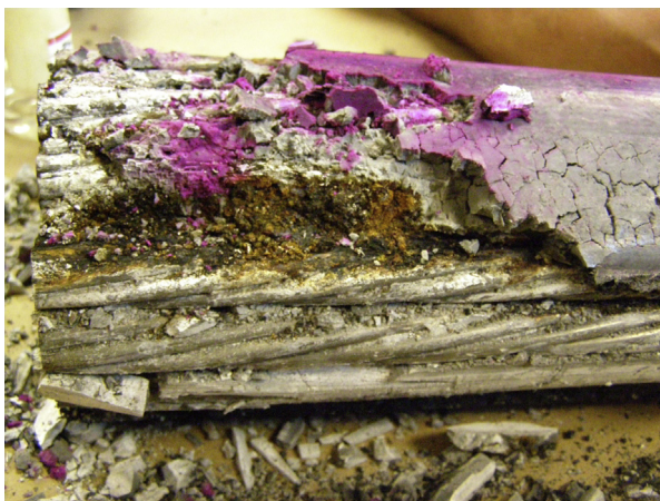
Figure 3.5 Corrosion of a strand embedded in deficient grout. Pink color shows the pH indicator (phenolphthalein) sprayed on the grout surface.
