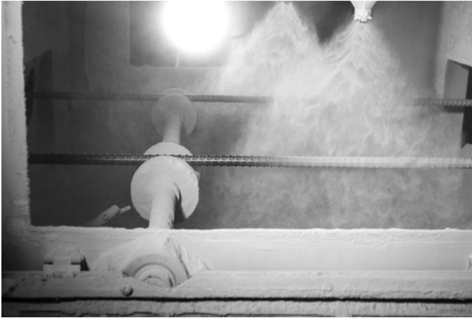
Figure 5.1 Epoxy powder being applied to cleaned and heated reinforcing steel. From Western Coating Inc.
