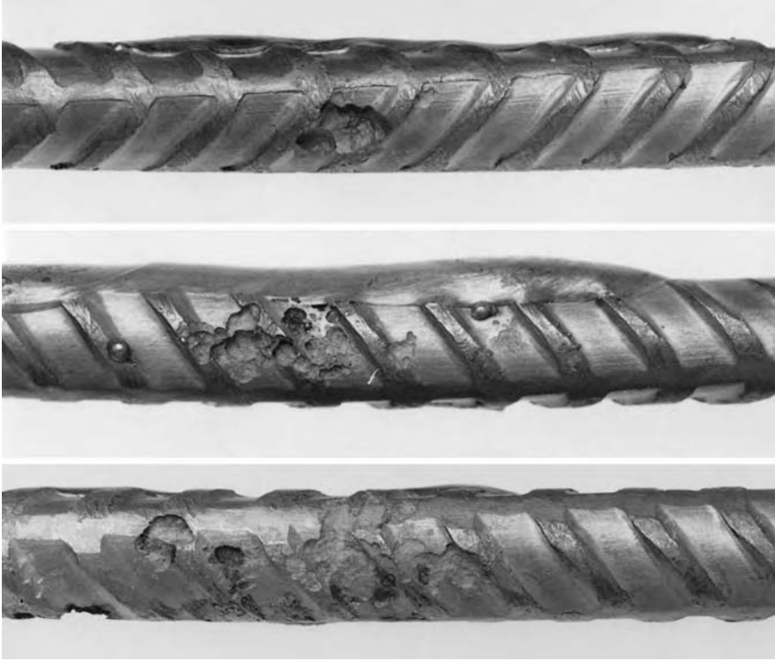
5.7 Corrosion of deformed reinforcing bars in concrete (2 years; 2.5 M.-% Cl - ).
