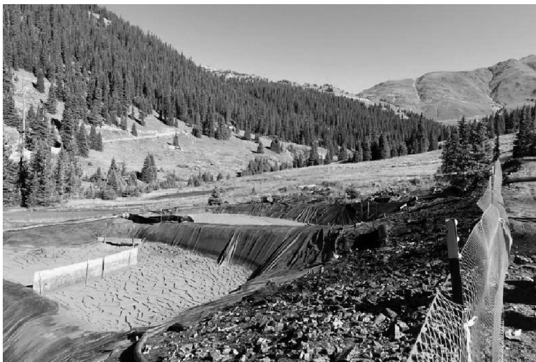
FIGURE 8.5 Settling ponds used to precipitate iron oxide and other suspended materials from nearby Red and Bonita mines drainage are shown in this August 14, 2015, photograph. (From USEPA, Emergency Response to August 2015 Release from Gold King Mine , U.S. Environmental Protection Agency, Washington, DC, 2016, http://epa.gov/goldkingmine . Photograph by Eric Vance/EPA.)
