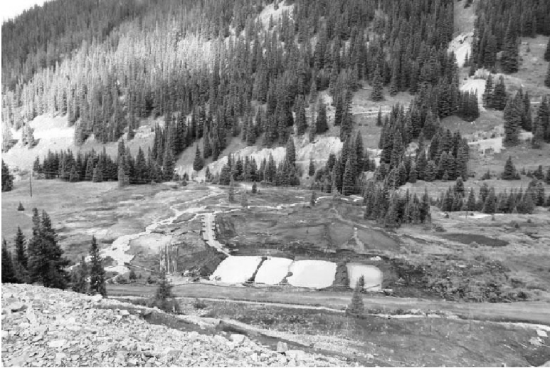
FIGURE 8.3 Treatment ponds built close to the Gold King Mine. When water leaves the mines, these ponds slow it down and allow pH adjustment to be made while letting contaminants settle to bottom. (From USEPA, Emergency Response to August 2015 Release from Gold King Mine , U.S. Environmental Protection Agency, Washington, DC, 2016, http://epa.gov/goldkingmine .)
