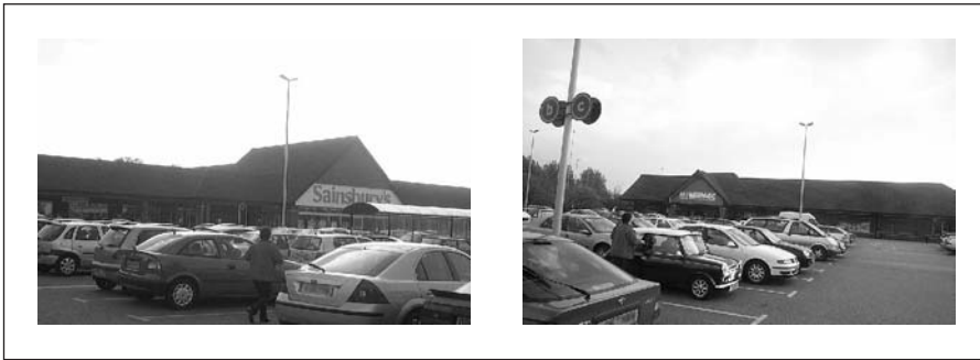
Figure 12.3 ● A typical example of creating the appearance of a pitched roof on a flat-roofed building.
