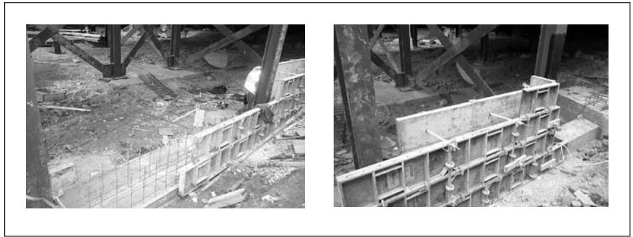
Figure 7.12 ● Creating concrete walls using formwork.
