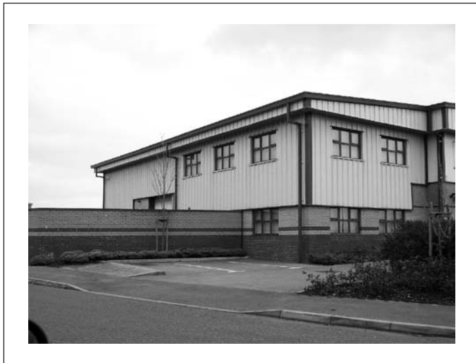
Figure 10.19 ● A building in which brickwork cladding has been used at the lower level and coated aluminium cladding for the upper level.
