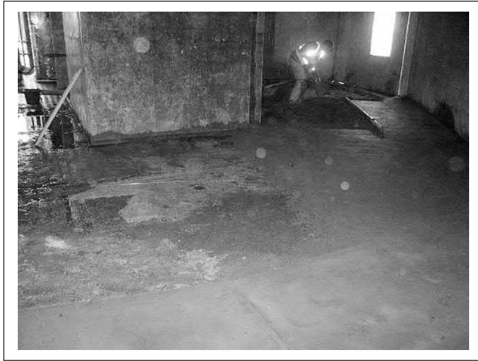
Figure 11.22 ● The screeding operation being undertaken.
