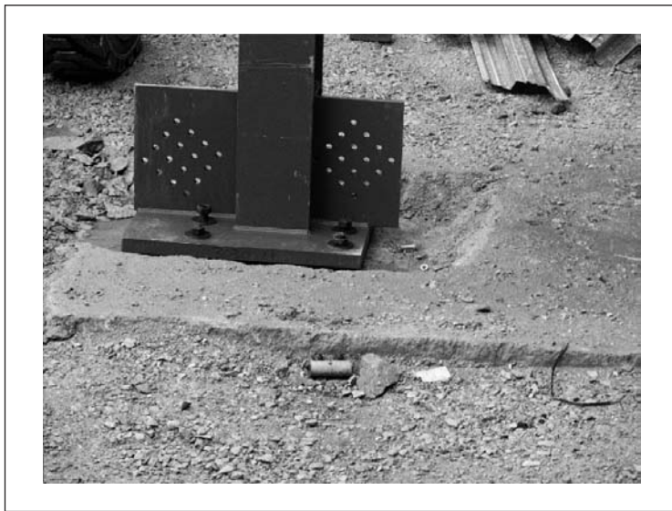
Figure 7.24 ● Reducing the level of a pad foundation by breaking out concrete.
