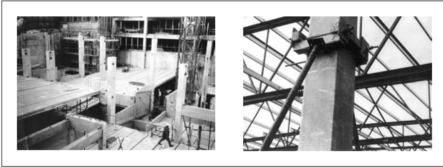
Figure 7.17 ● Erecting a precast concrete frame.
