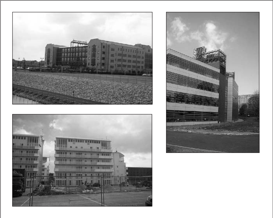
Figure 1.3 ● Modern, sophisticated buildings require careful design of structure fabric and services to ensure that they meet user requirements.
