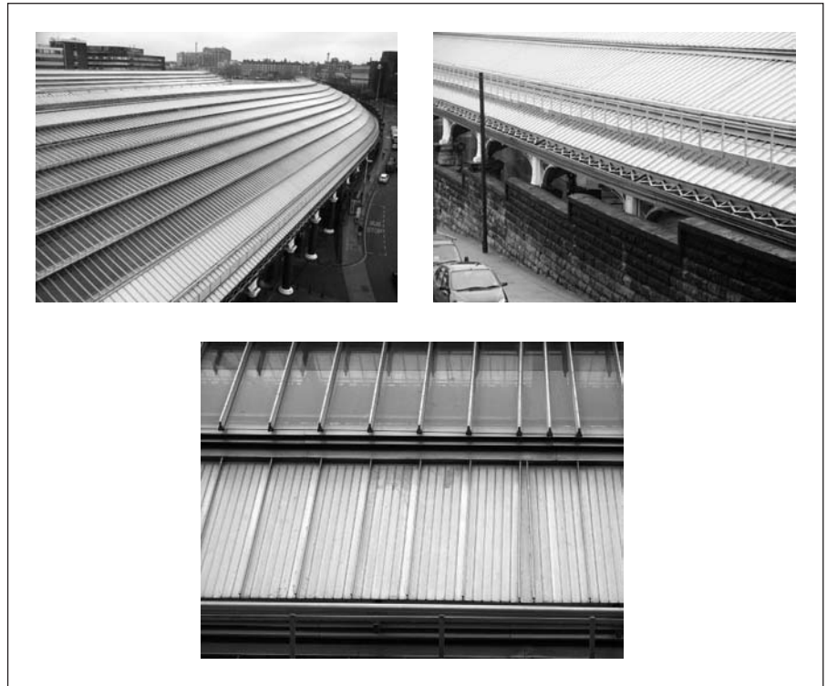
Figure 12.20 ● Soft metal roof covering.
