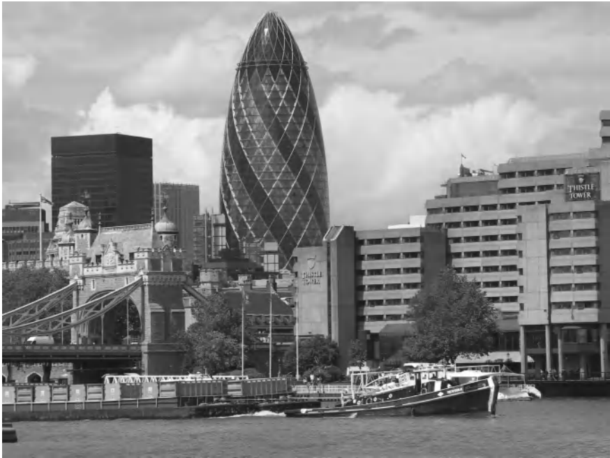
Figure 6.4 The building commissioned by Swiss Re at 30 St Mary Axe, London. Image courtesy of Stephen Pryke.
