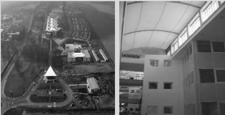
Figure 15.1 The ANSR external view and inside of office facility [5].
