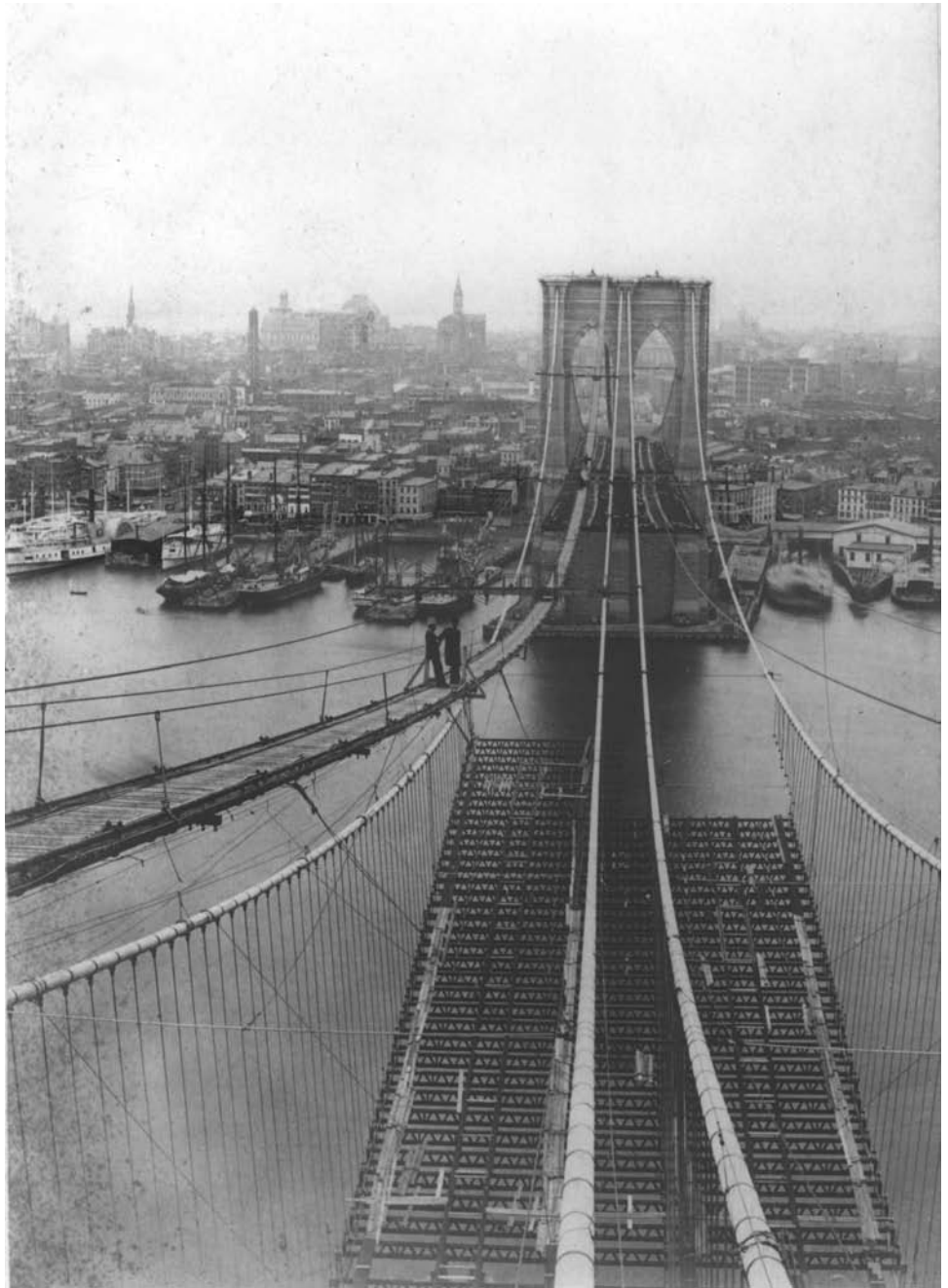
Figure 1.4 Brooklyn Bridge under construction 1881. (Museum of the City of New York, Print Archives, Gift of the Essex Institute)
