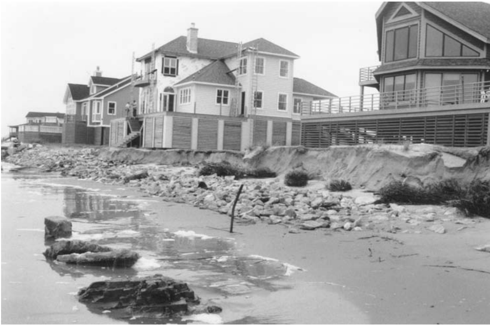
FIGURE 12-2 Reconstruction of expensive homes on eroding barrier beach at Isle of Palms, South Carolina, after Hurricane Hugo in 1989. The middle house is under construction. ( Photo by author. )
