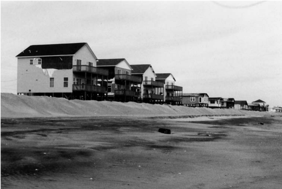
FIGURE 7-3 Buildings threatened by coastal erosion, North Carolina. (Photo by author.) Also see Figure 12-2.
