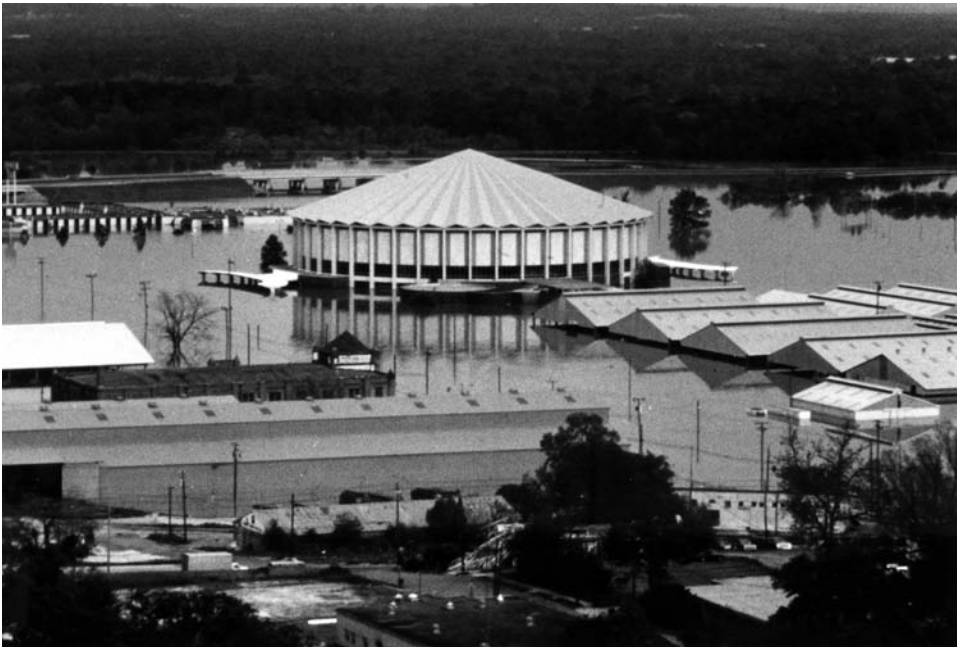
FIGURE 12-5 The 1979 Pearl River flood at Jackson, Mississippi. State Coliseum and industrial and commercial buildings built in area protected by Corps of Engineers flood control project were inundated. (Photo by author.)
