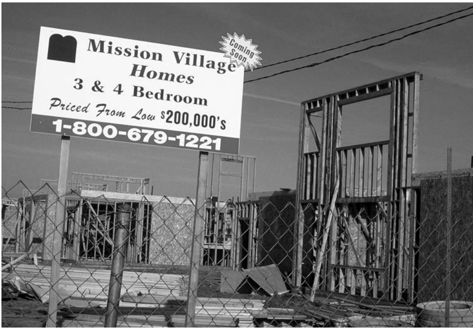
FIGURE 6-9 “Affordable” new housing under construction in Riverside, California, 2002. (Photo by author.)
