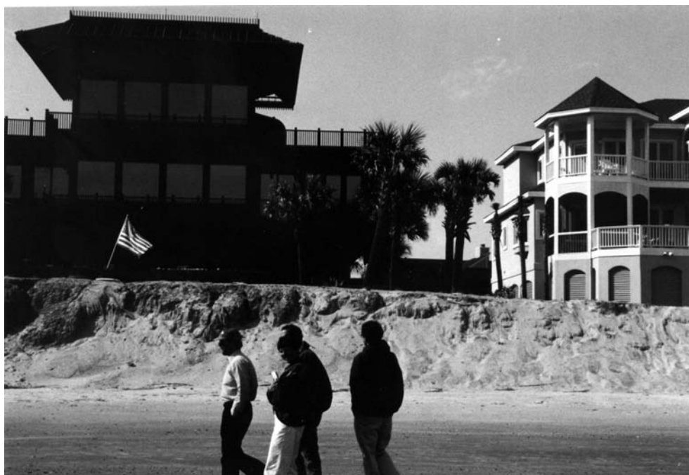
FIGURE 10-1 The site of the Lucas v. South Carolina Coastal Council case. The state's defeat in the U.S. Supreme Court eventually led to the construction of the house on the right on one of the Lucas lots. The beach scarp indicates that the inlet is shifting toward the houses again. (Photo by author.)
