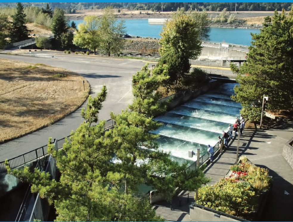
Fish ladders, like this one at the Bonneville Dam in Oregon, are built to help fish travel across dams.
