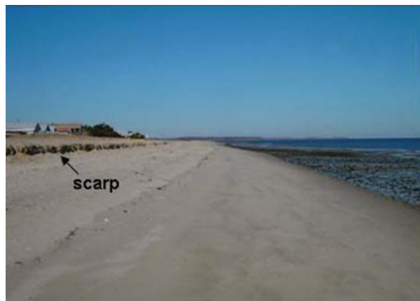
Fig. 5 View of Bowers Beach, DE, showing the development of a scarp on the foreshore after beach nourishment
