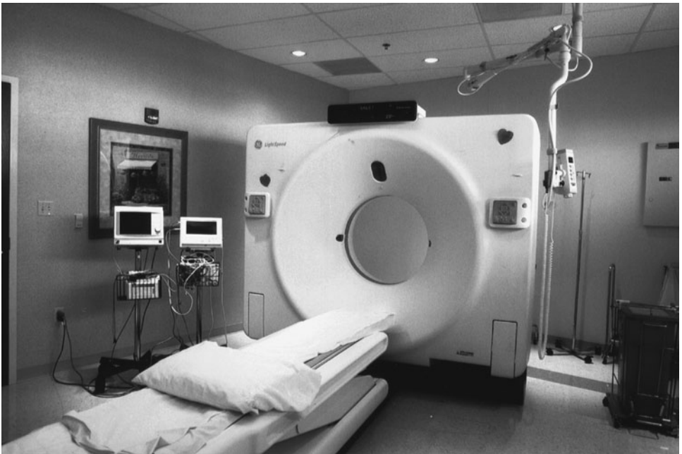
Figure 10-16. Computed axial tomography, CT, scanner. (Reproduced with permission of the National Council on Radiation Protection and Measurements from Structural Shielding Design for Medical X-Ray Imaging Facilities . Bethesda, MD: National Council on Radiation Protection & Measurement; 2004. NCRP Report 147.)
