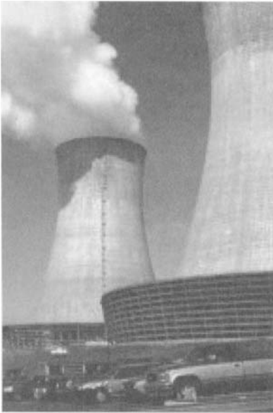
Figure 8.9 Natural-draft cooling towers in a nuclear power plant. The packing occupies only the bottom section; the rest of the tower acts as a chimney to create the flow of air. (Courtesy of Michael Rennhack, NukeWorker.com.)
