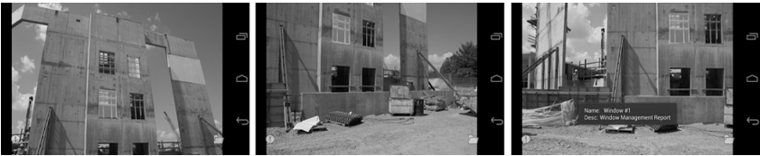
Figure 6. On-site localization results using Android smartphones. Cyber information is precisely overlaid in all different viewpoints.
