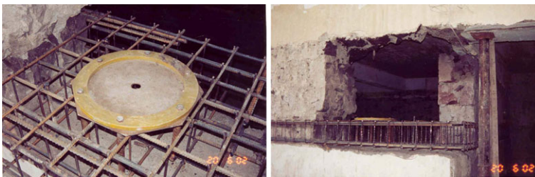
Fig. 9 The views of the lower reinforcement frames of the lower pedestal installed in the opening together with the isolator socket
