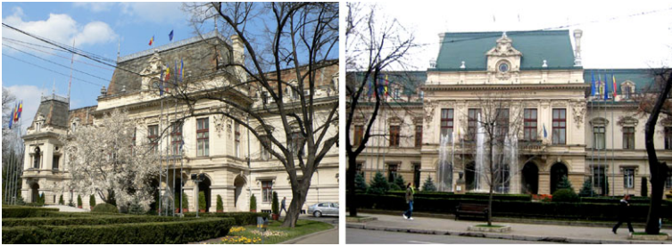
Fig. 15 Views of the Iasi City Hall building
