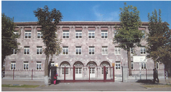
Fig. 5 General view of the retrofitted by base isolation 3-story school building
