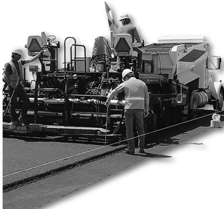
Figure 23.14 A string line guiding a paver. (Courtesy Topcon Positioning Systems.)
