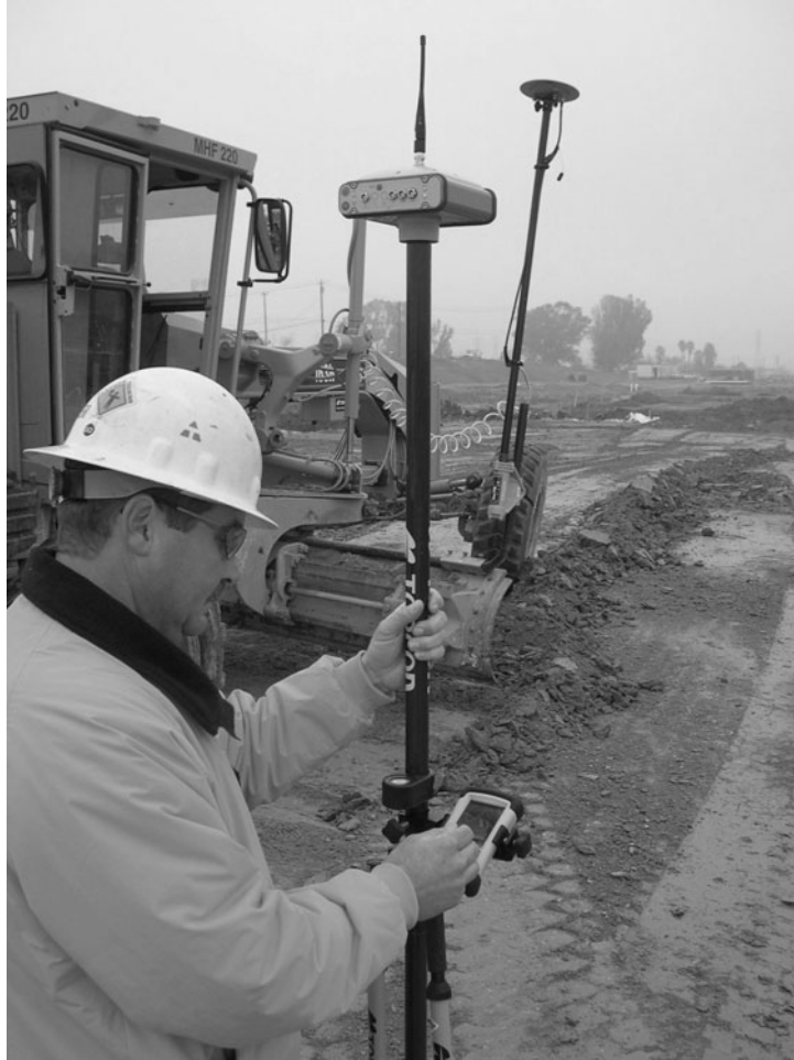
Figure 15.7 GNSS antenna mounted on a grader blade. (Courtesy Topcon Positioning Systems, Inc.).
