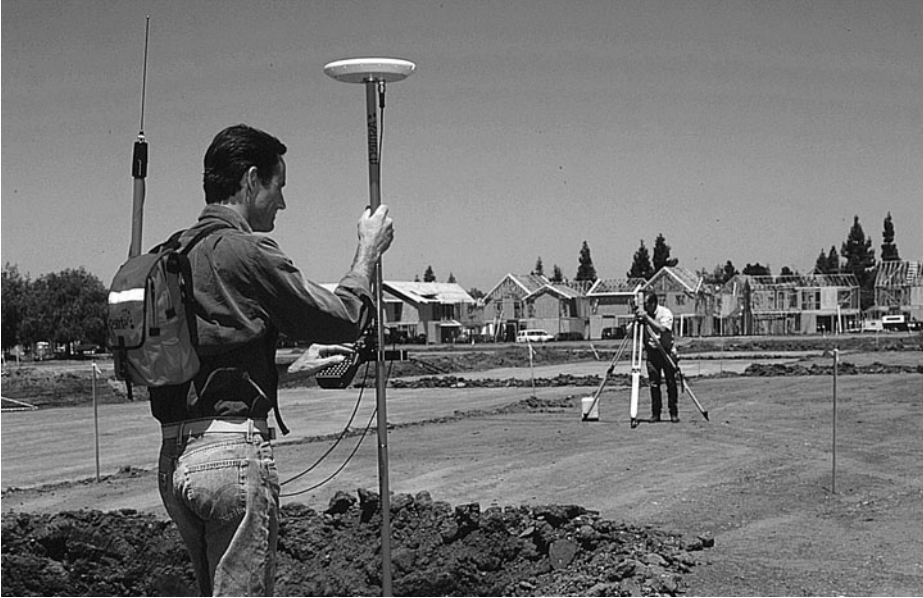
Figure 14.1 GPS receiver being used in construction stakeout. (Courtesy of Ashtech, LLC.)
