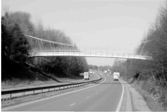
Figure 4 A30 Halgavor Bridge – After completion
