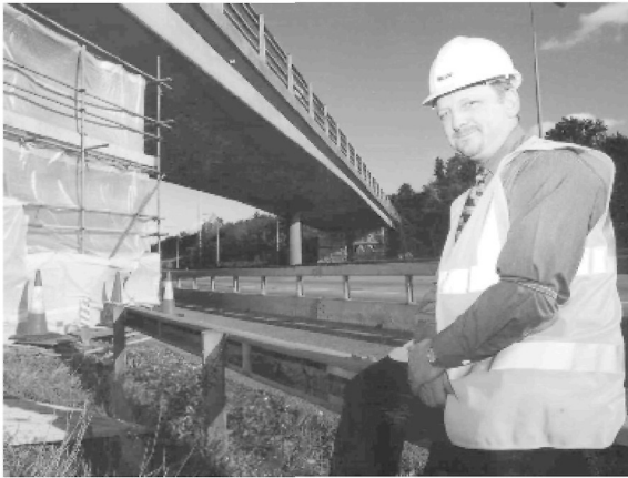
Figure 2 M11 Coopersale Bridge – Column wrapping
