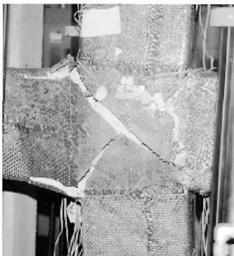
Figure 1 Failure mode of wrapped beam-column joint
