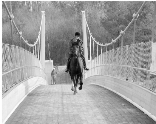
Figure 5 A30 Halgavor Bridge – In use
