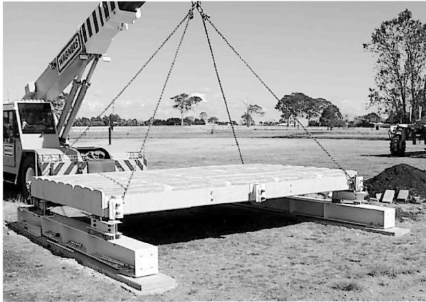
Figure 12 5m test bridge being lifted into place
