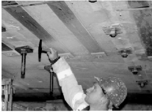
Figure 1 M60 Barnes Bridge - Hammer testing composites
