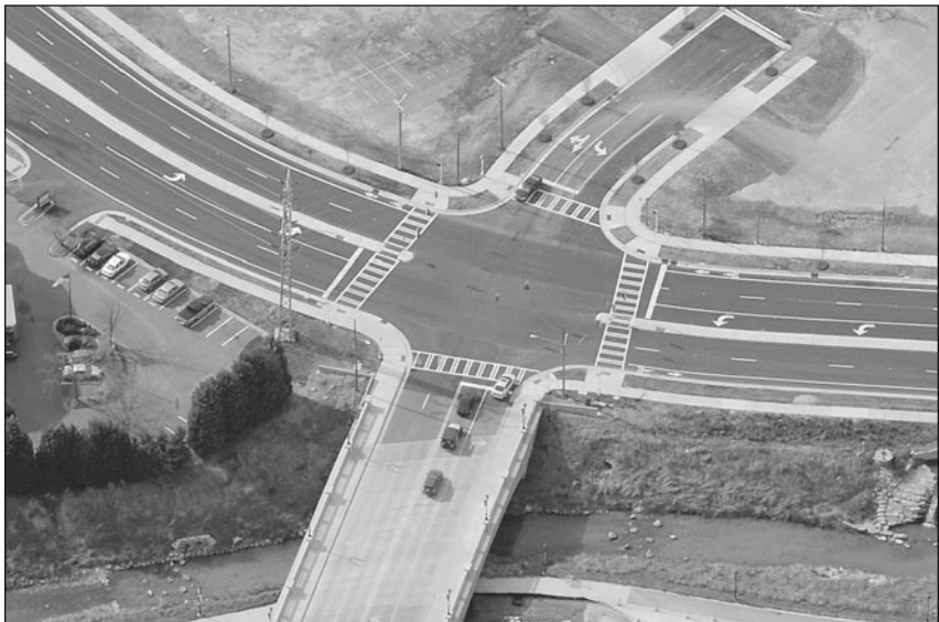
Pedestrian and bicycle safety improvements at an expanded intersection in Charlotte. (Photos courtesy Mecklenburg County and Pictometry International.)
