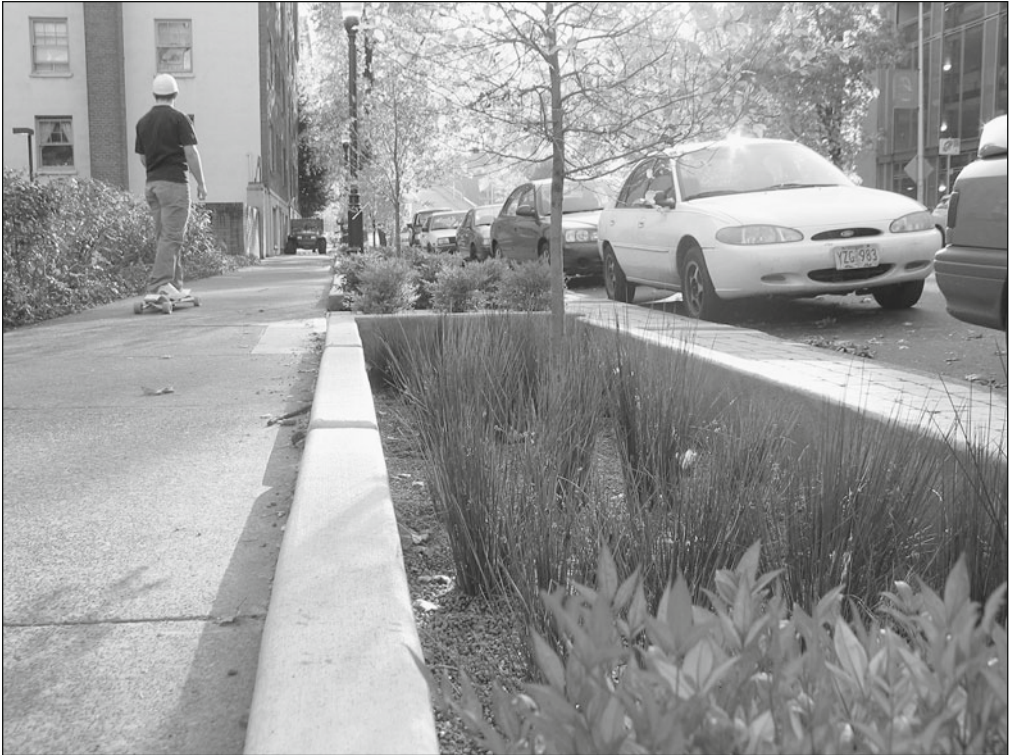
Many communities are combining complete streets initiatives with “greening” their streets to better handle storm water runoff. (Photo courtesy Kevin Robert Perry.)
