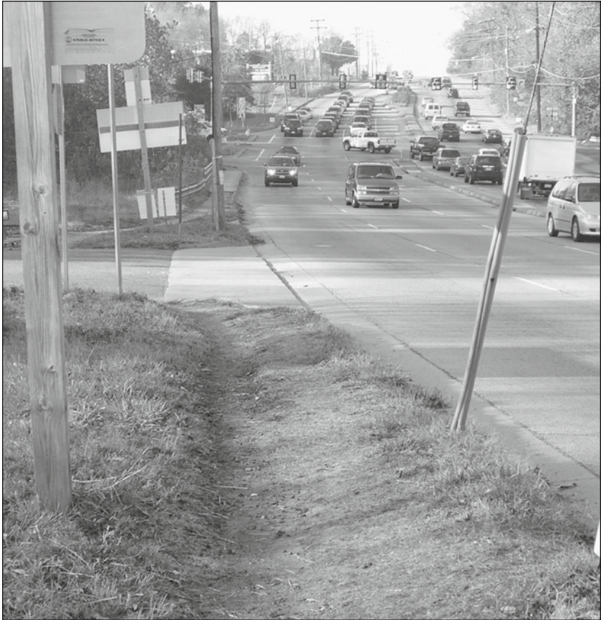
A “goat track” on Route 1 in northern Virginia is evidence that people walk along this road. (Photo by Barbara McCann.)
