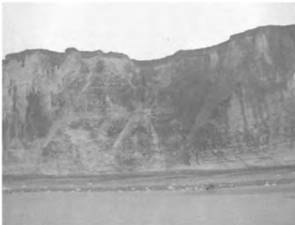
Veules-les-Roses, Newhaven Chalk, steeply inclined conjugate joints (pyramidal structure)
