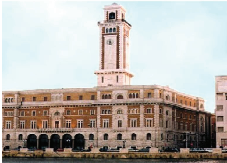
Fig. 1. View of the Provincial Administration Building of Bari (a) and of the investigated tower (b)
