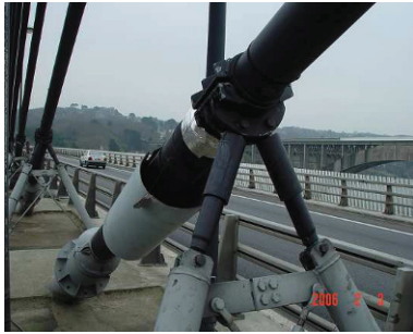
Fig. 1 Dampers device of Iroise Bridge (FR)
