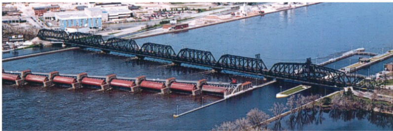
Fig. 1 Government Bridge at the Rock Island Arsenal with Davenport, IA in the upper left (Spans are numbered from right to left)
