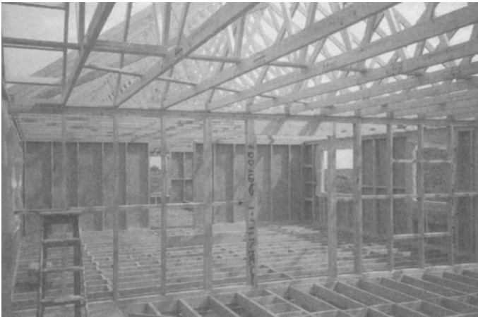
Figure 10.6 Timber-framed house construction (Photograph courtesy of Mr Mark Inglis)
