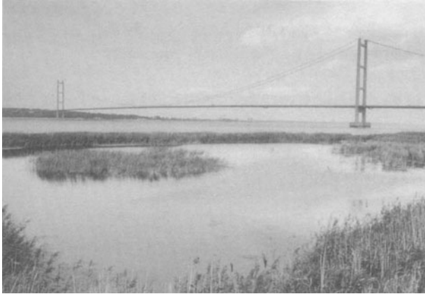
Figure 1.3 Humber suspension bridge (Courtesy of F. Sawko)
