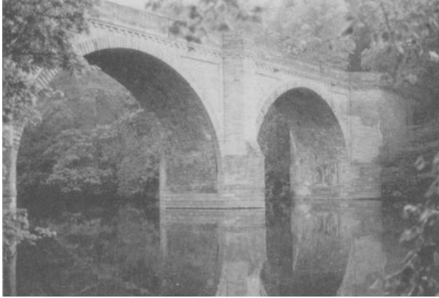
Figure 1.1 Masonry arch bridge (Courtesy of A.W. Sawko)
