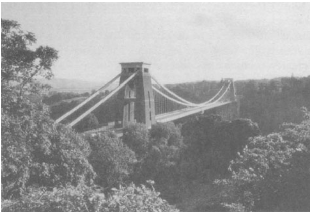
Figure 1.2 Clifton suspension bridge, Bristol (Courtesy of F. Sawko)
