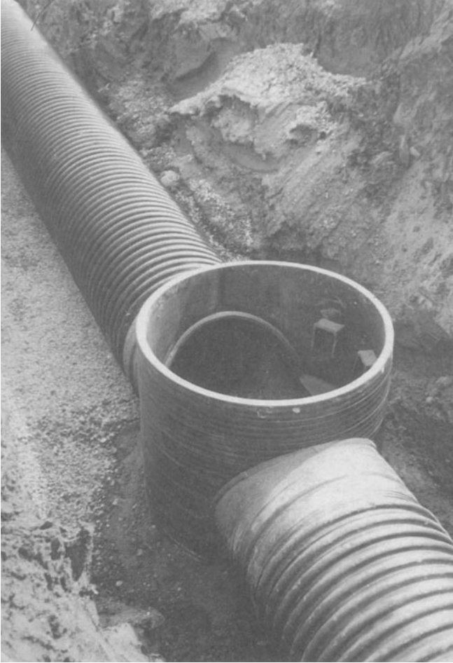
Figure 31.2 Large-diameter HDPE pipe of extruded spiral wall construction used for drainage (Courtesy of Bauku GmbH)
