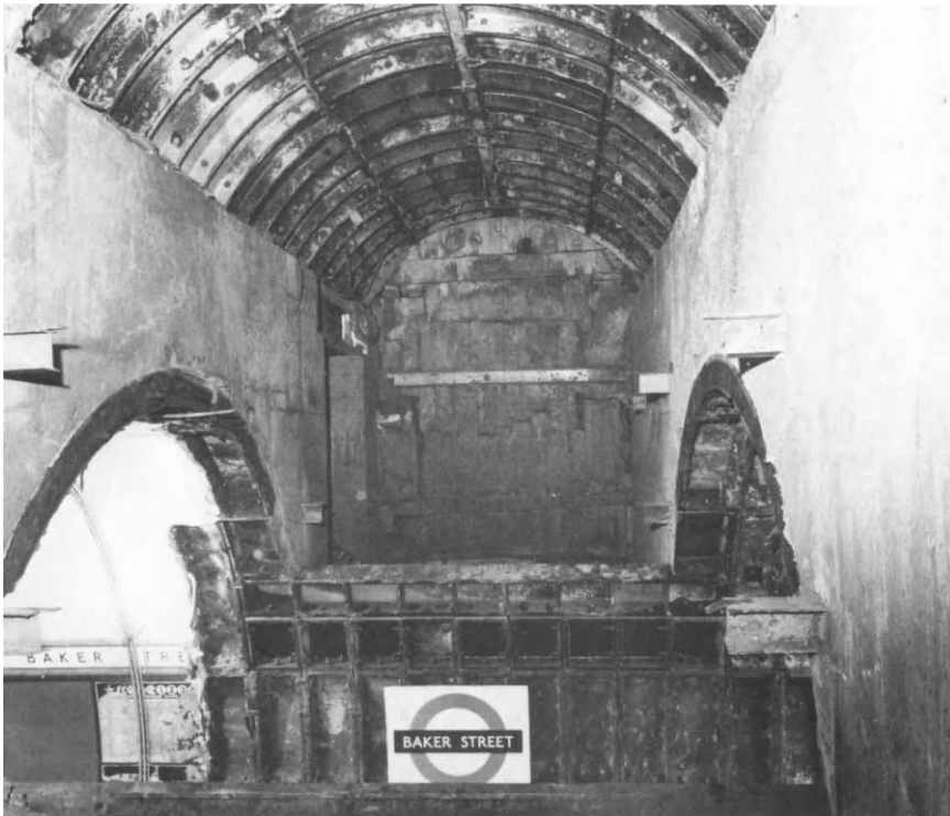
Figure 14.8 Overbridge cut across top of cast iron station tunnel
