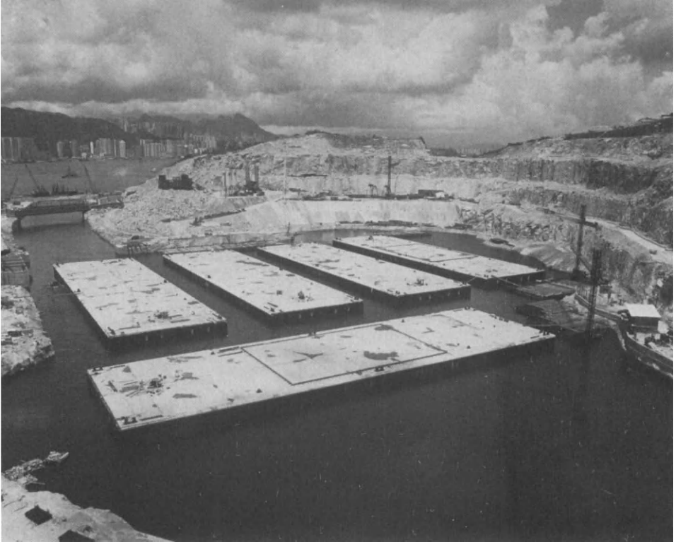
Figure 11.1 Tunnel units ready for towing (Eastern Harbour Crossing)
