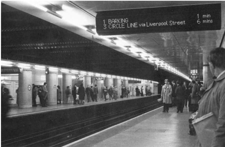
Figure 3.3 A side platform station constructed by cut and cover methods with the steel beam supporting the roof visible over the tracks
