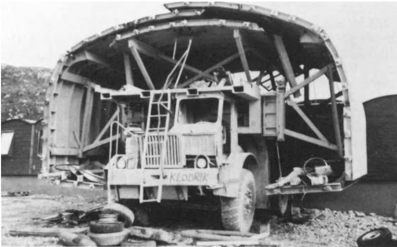
Figure 17.19 Mobile 6 m steel shield for use in a 68 m 2 tunnel
