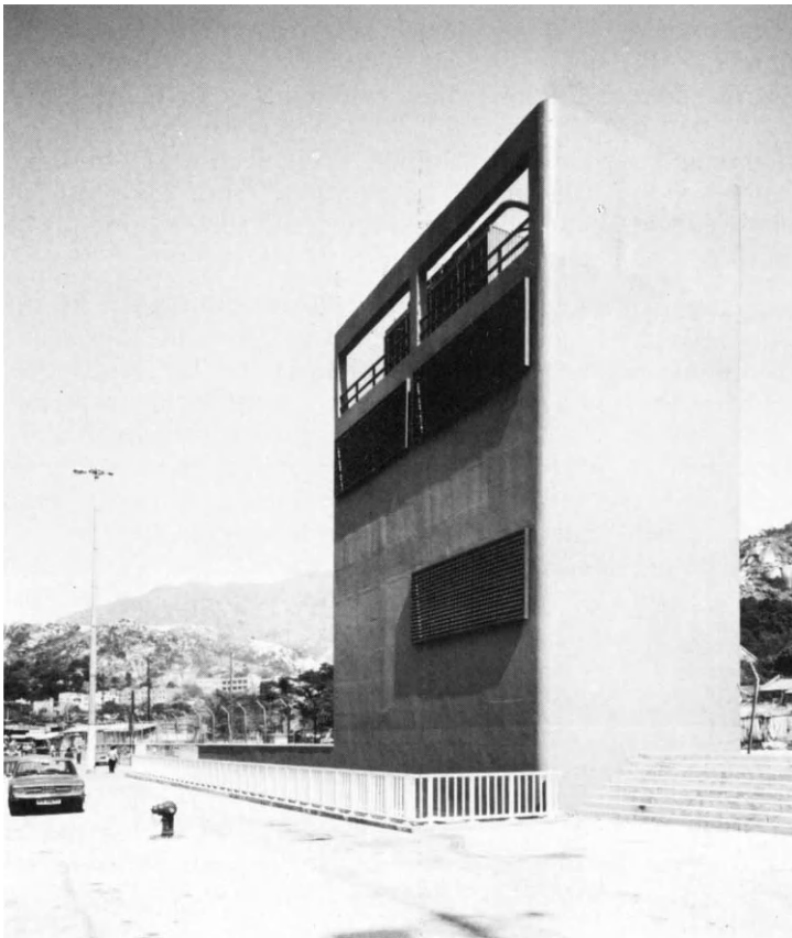
Figure 3.10 A ventilation structure incorporating inlet and exhaust shafts from an underground station, and accommodating chiller units for the environmental control system
