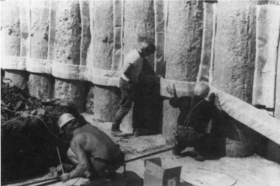
Figure 8.10 Contiguous wall 'drained' with a geotextile fabric (courtesy BTR Landscaper and Cementation Piling & Foundations Ltd)
