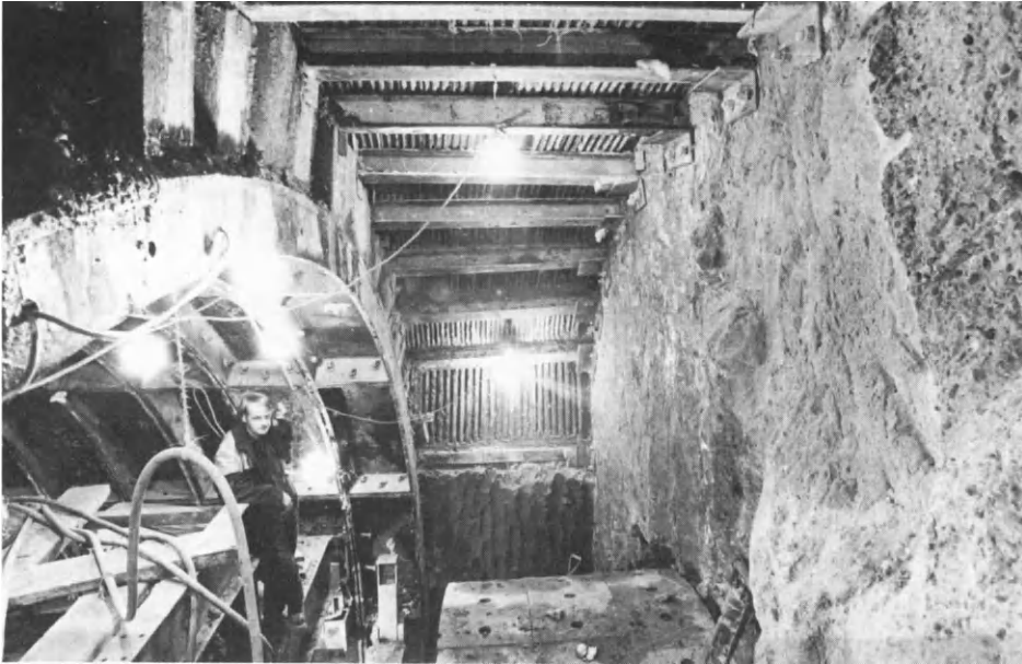
Figure 14.9 Temporary works for ring wall connecting to cut and cover structure
