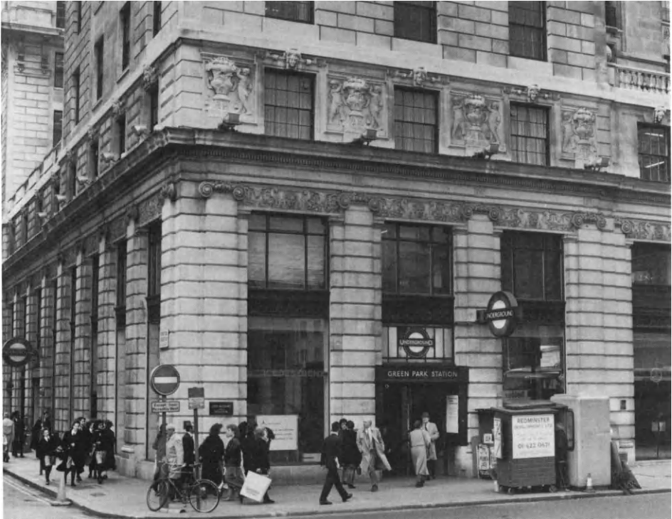
Figure 3.1 An entrance to an underground station incorporated into a high-quality commercial building. The corner site allows two entries to be provided; one on each of the two roads
