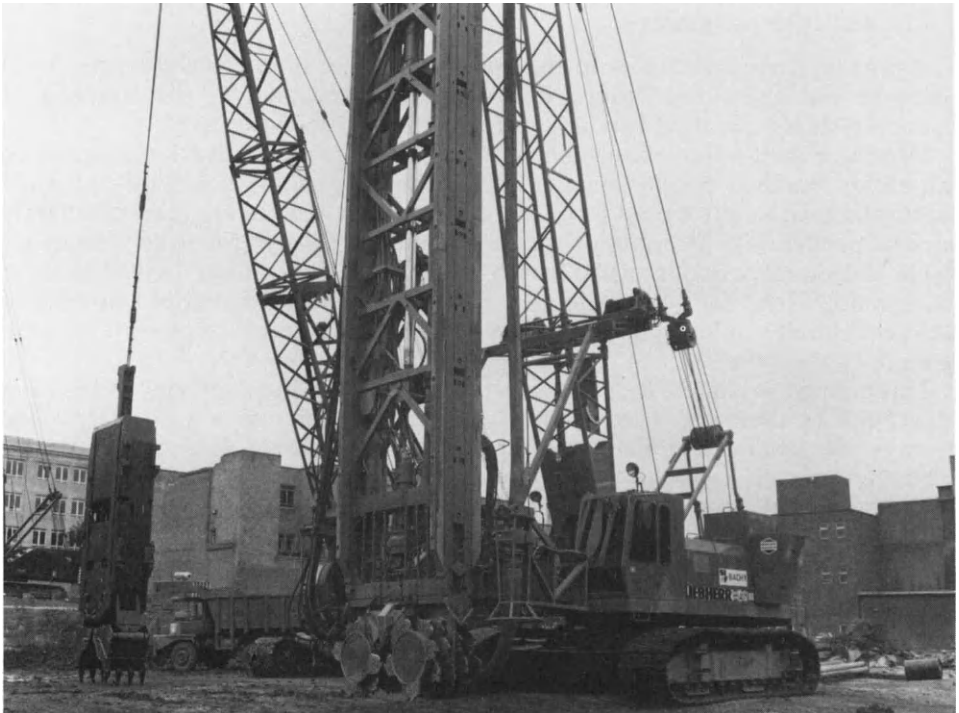
Figure 7.13 Typical diaphragm wall excavation equipment; clamshell grab on the left and trench cutter on the right
