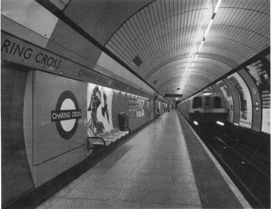
Figure 3.4 A single track and a 3 m wide platform accommodated within a 6.5 m diameter bored tunnel
