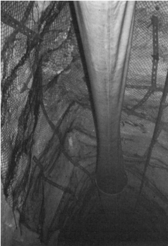
Figure 17.16 Rock mesh and straps between rock bolts in rockburst conditions
