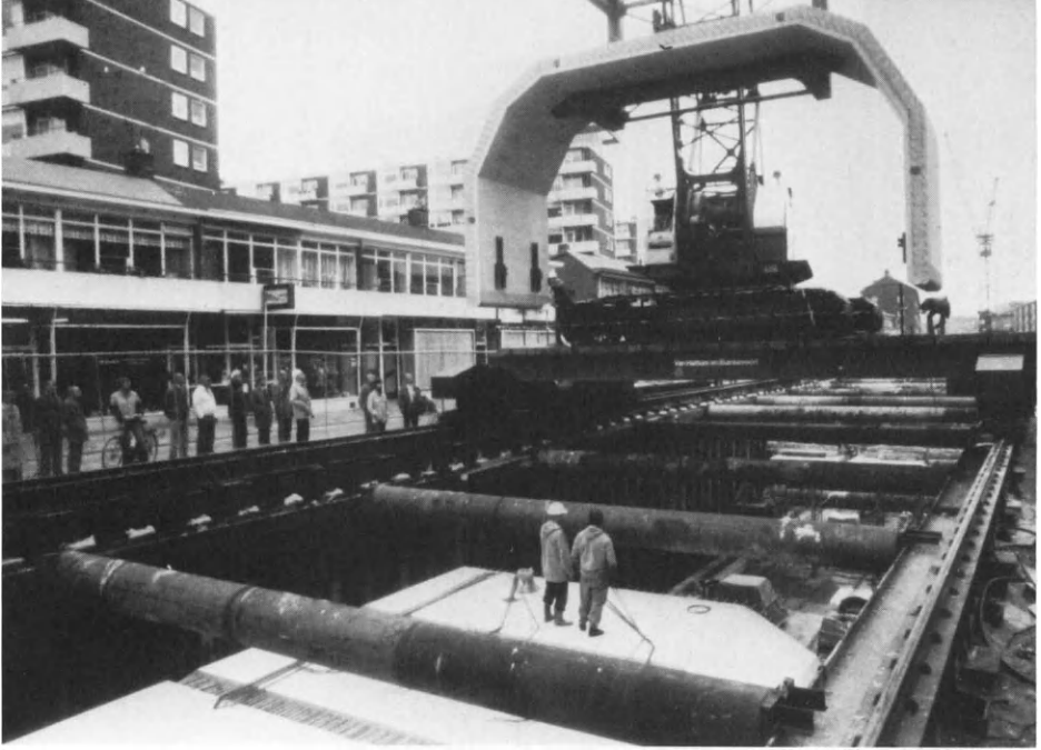
Figure 12.19 Manoeuvring a shell segment into the tunnel trench in Schiedamseweg
