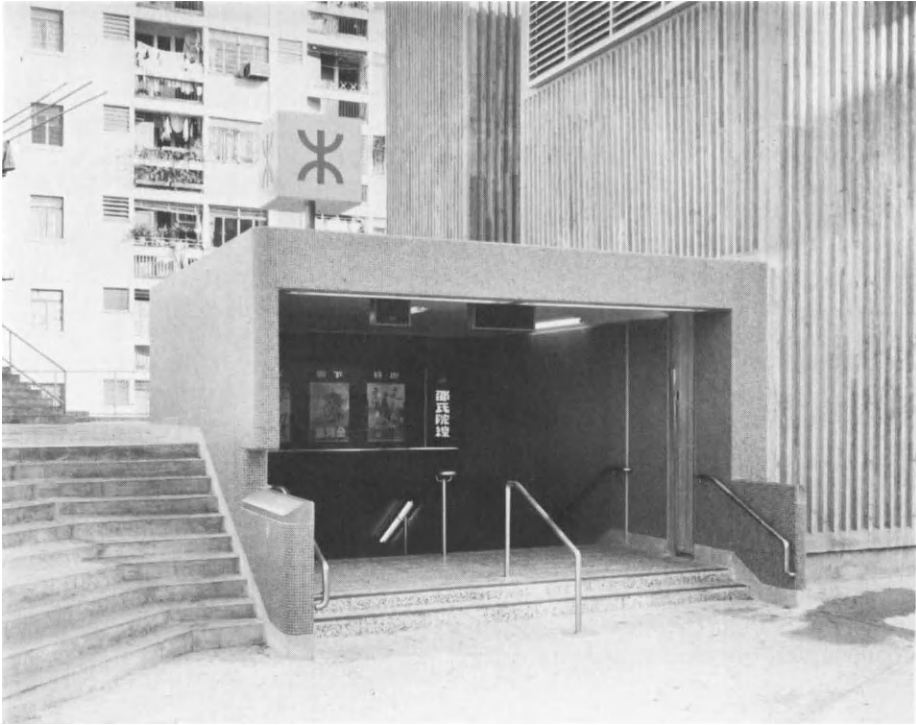
Figure 3.6 A free-standing entrance adjacent to a ventilation shaft structure. The threshold is raised above the street level to prevent the entry of flood water
