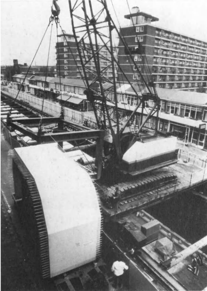
Figure 12.18 Handling a shell segment from a truck transporter in Schiedamseweg
