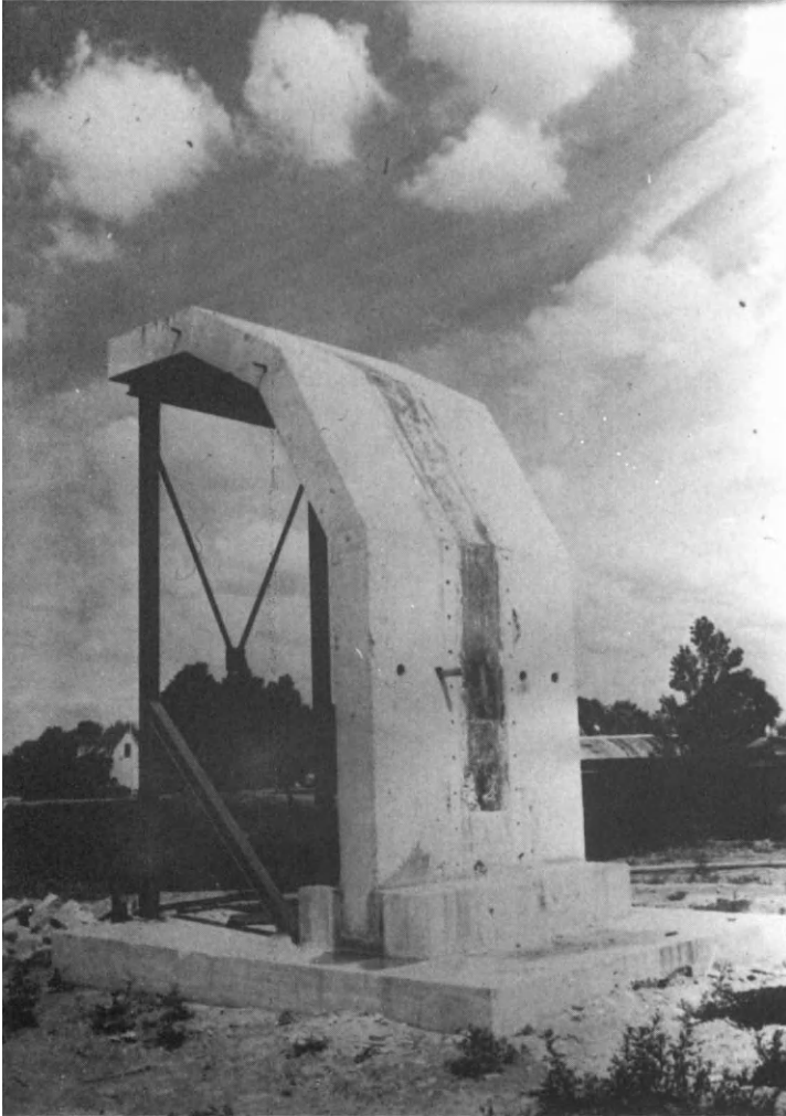
Figure 12.12 Full-size testing of a shell tunnel
