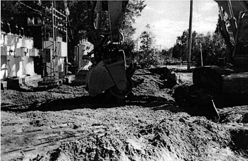
Fig. 1. In situ solidification/stabilization field application.
