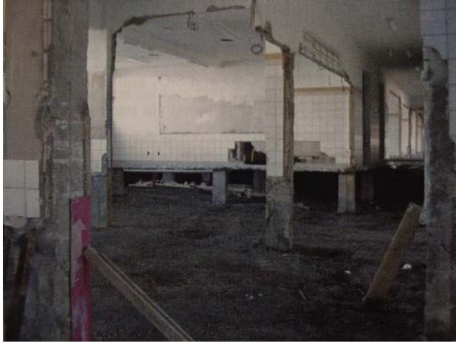
Figure 2.4 Removal of slag applied as fill [25]
