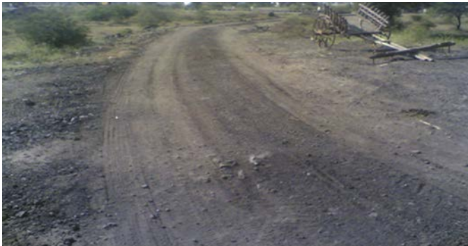
Figure 7.7 WBM approach road Aurangabad–Jalna, MS, India
