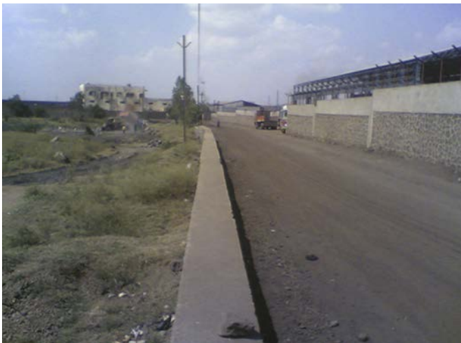
Figure 7.8 Approach road to the Dhanlaxmi Steel Ind. Pvt. Ltd at MIDC, Jalna, MS, India
