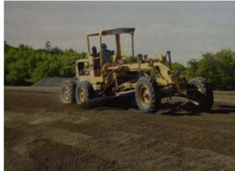
Figure 2.5 Accelerated hydration of instable components in slag; (a) slag splashing; (b) slag mixing [25]
